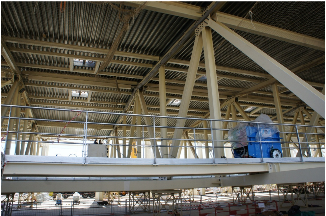
Photograph 12: 2015-08-25 – Walkways installed at the bottom chord level of the roof trusses
