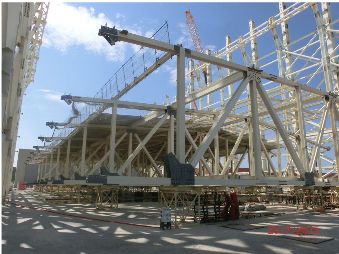
Photograph 16: 2015-07-23 – Roof steelwork and cladding progressing at ground level
