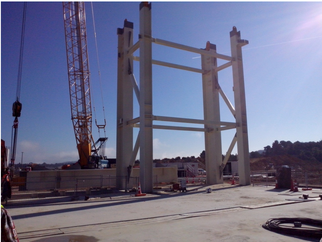
Photograph 38: 2014-10-02 – Four columns installed at Level 1 on the East façade
