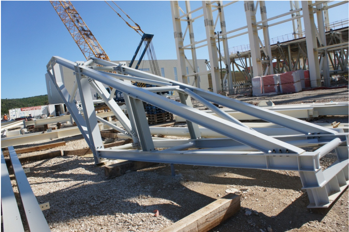
Photograph 9: 2015-08-25 – Lifting frame to be installed at the top of the column
