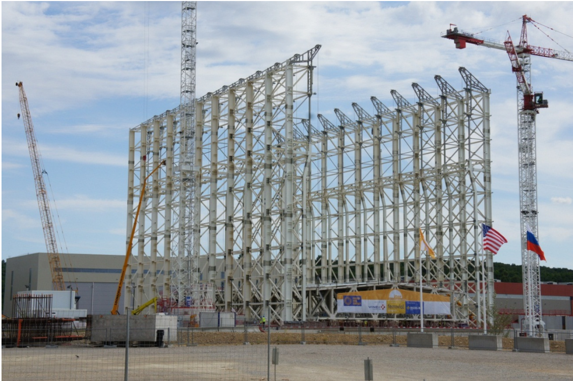
Photograph 5: 2015-09-08 – Columns ready to receive the roof pre-assembled at ground level
