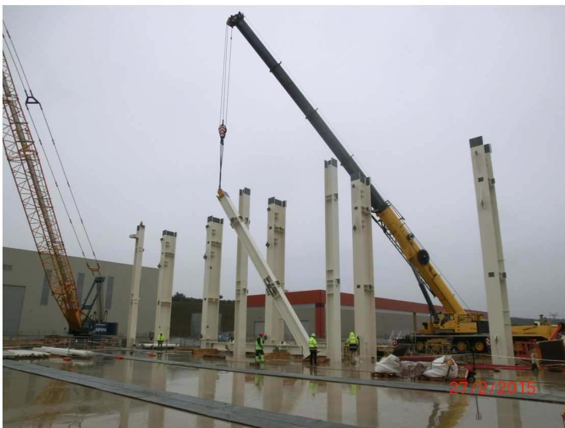
Photograph 28: 2015-02-27 – Installation of Level 1 columns on the West facade
