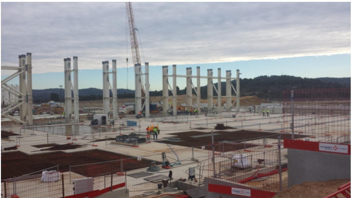
Photograph 32: 2014-12-10 – North West view showing box outs on the ground floor slab
