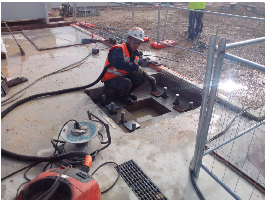
Photograph 43: 2014-09-25 – preparation of HD bolts before column erection
