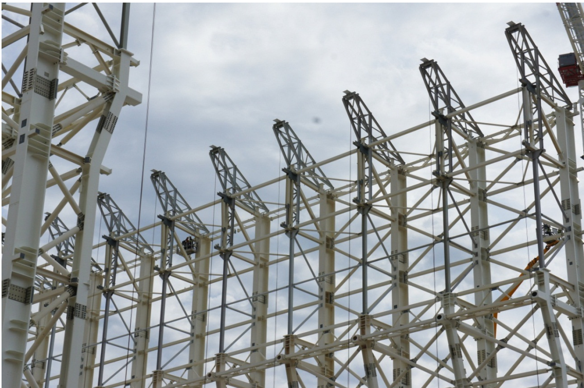
Photograph 6: 2015-09-08 – View of the temporary lifting frames at the top of the columns
