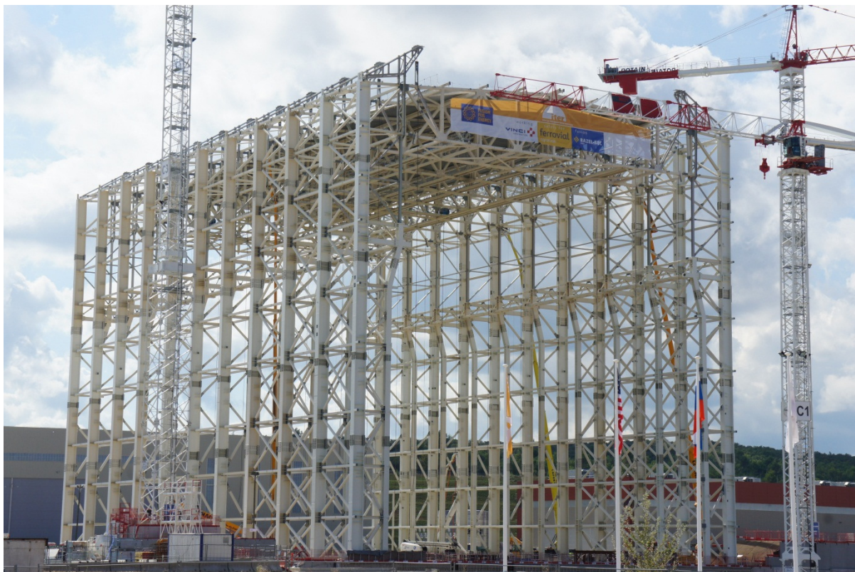
Photograph 1: 2015-09-11 – Roof structure lifted to its final position at 60m height
