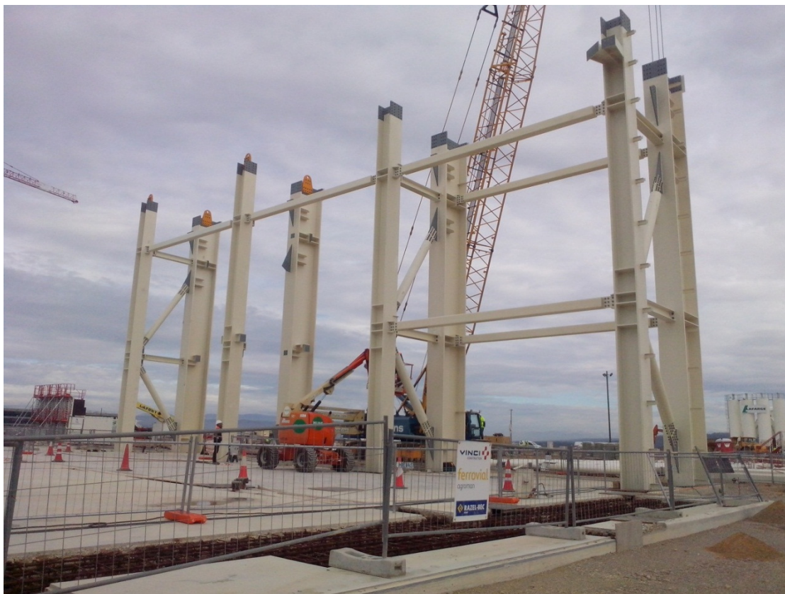
Photograph 35: 2014-10-16 – Eight columns installed at Level 1 on the East façade
