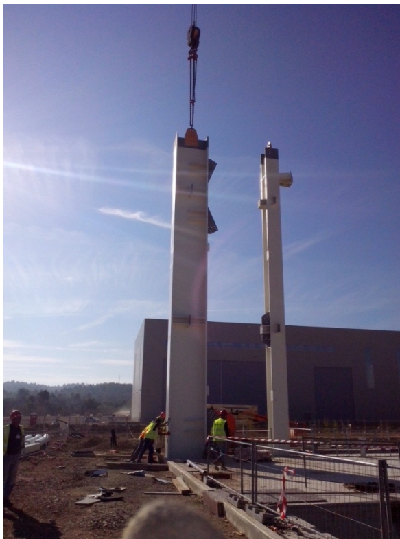
Photograph 40: 2014-09-26 – Two columns installed at Level 1 on the East façade
