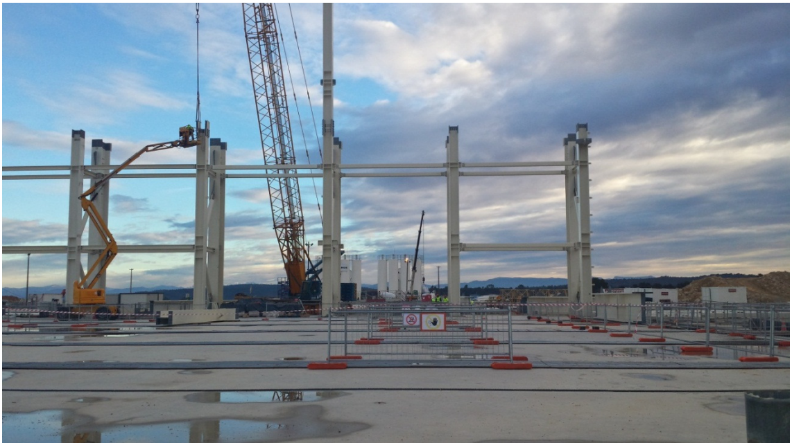
Photograph 30: 2014-12-18 - First Level 2 column installed on the East façade
