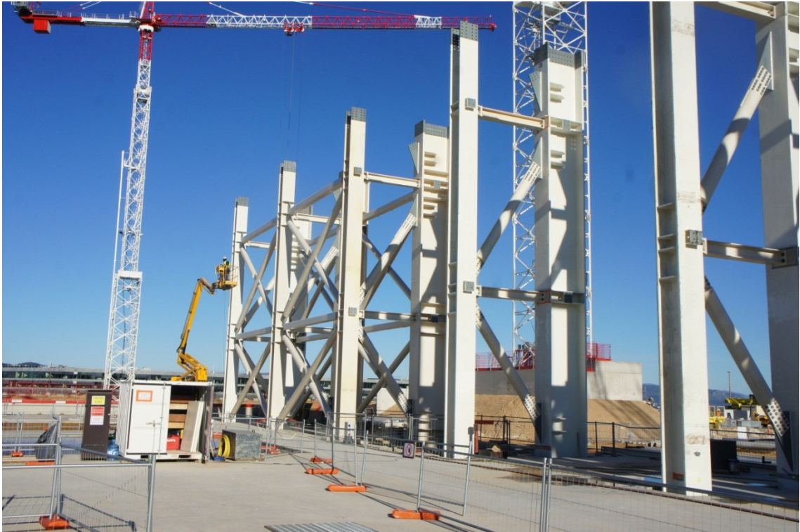
Photograph 31: 2014-12-11 – Cross-bracing at Level 1 East façade
