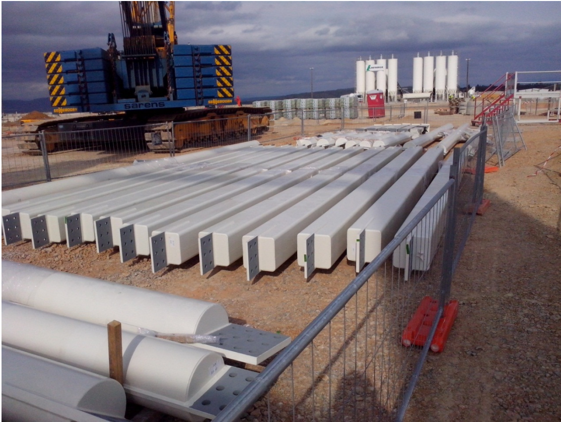
Photograph 37: 2014-10-07 – temporary storage of beam-bracing components on site
