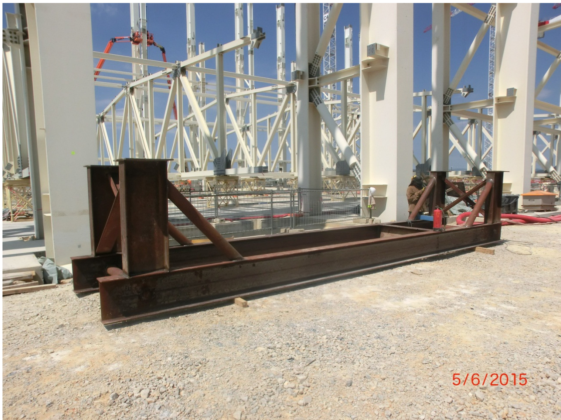
Photograph 22: 2015-06-05 – temporary steel frame to bridge the incomplete box-outs
