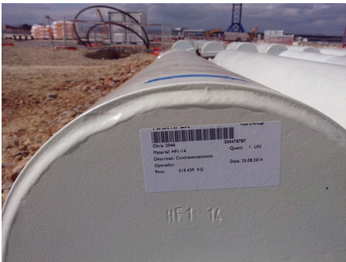
Photograph 44: 2014-09-19 – Hard-stamped component site reference
