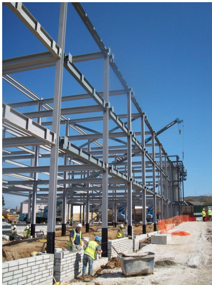
Figure 6.4: Steel frame for a 3-storey building
