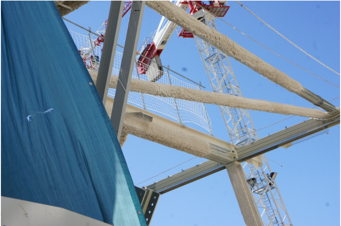
Photograph 11: 2015-08-25 – Vermiculite fire protection being applied to the roof steelwork
