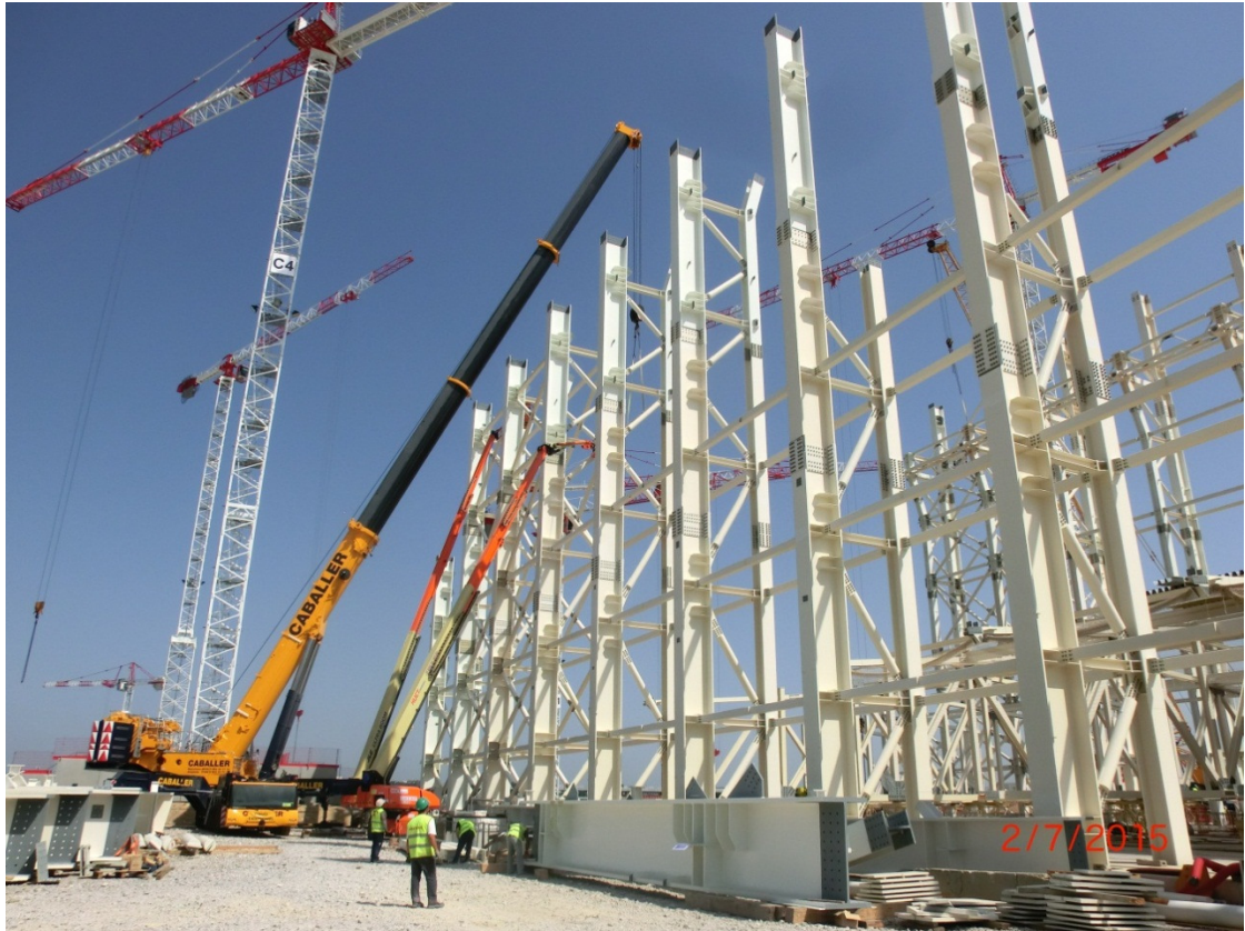
Photograph 19: 2015-07-02 – West façade column erection
