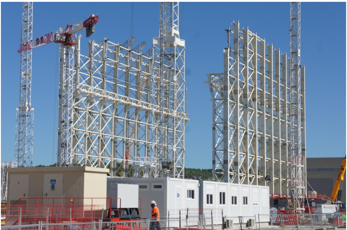
Photograph 14: 2015-08-15 – Some of the lifting frames installed above the Level 5 columns
