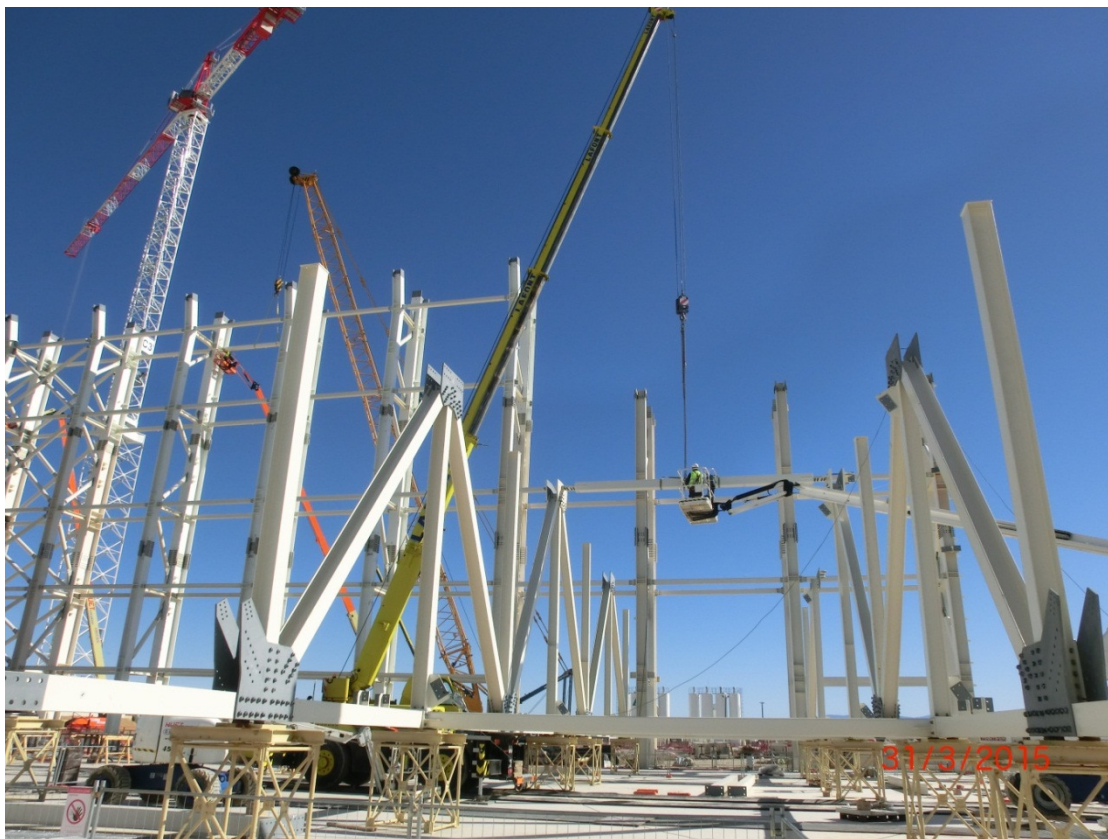
Photograph 27: 2015-03-31 – Start of the roof pre-assembly at ground level
