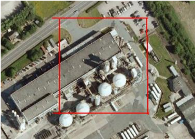
Site 16 - Rose Cottage, Manchester Rd, Carrington, Manchester M31 4AY
