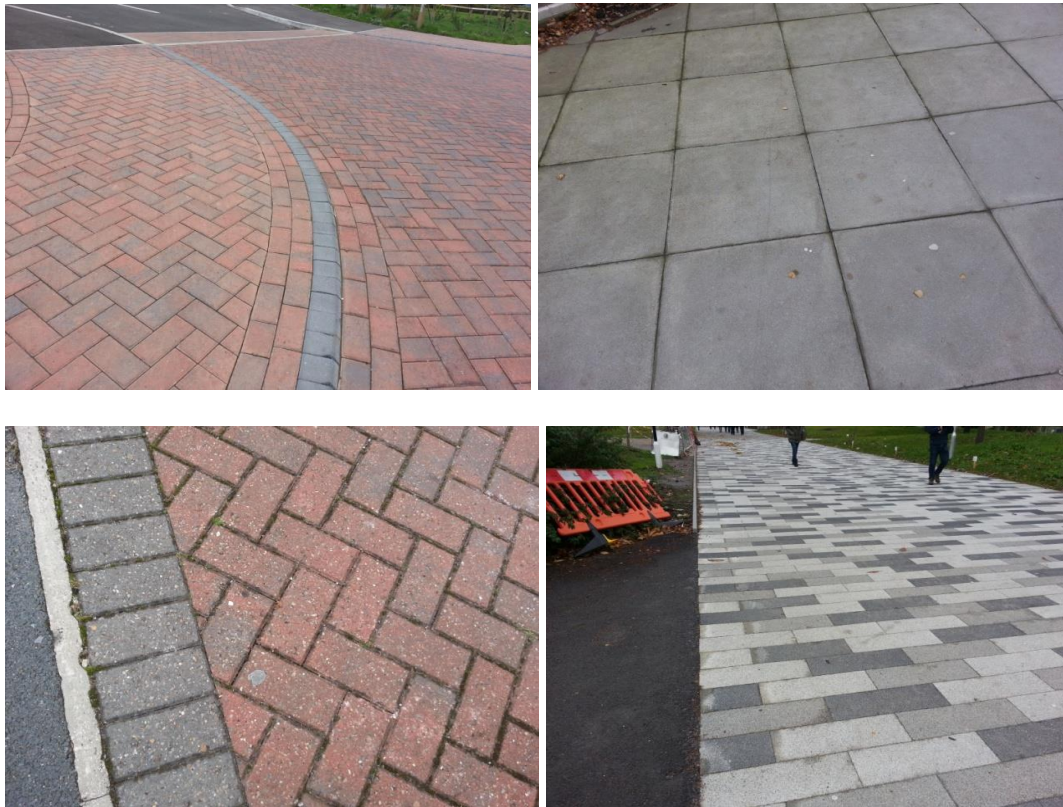
Fig. 6.6: Various forms and designs of permeable pavements from example sites. Photos were taken by Vincent Uzomah.
