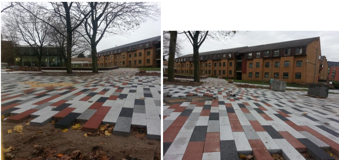
Fig. 6.4: Retrofitting permeable pavements in the presence of mature Norway Maple. A – is the site before retrofitting; B – the site being retrofitting. Photos taken by Vincent Uzomah.
