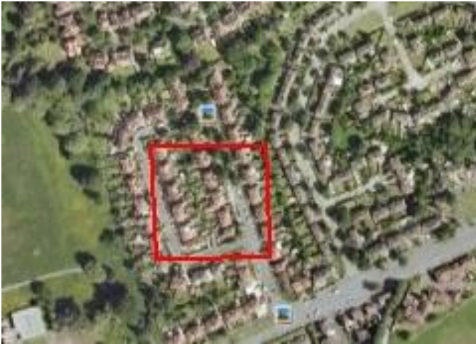
Site 10 - Redland Crescent M21
