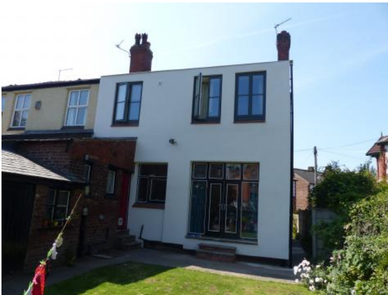
Figure 15 Completed External Wall Insulation on Carbon Co-op house
