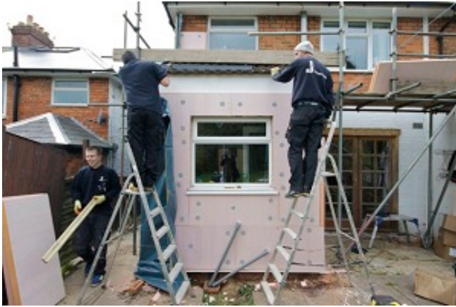
Figure 20 ESC Competition winner's external wall insulation in progress (Northfield Ecocentre, 2015a)
