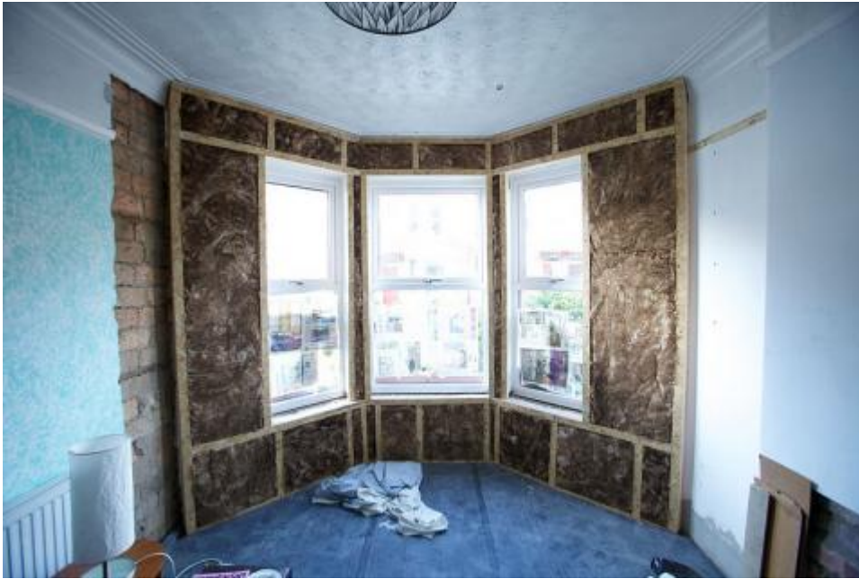
Figure 16 Internal wall insulation being applied to Carbon Co-op house
