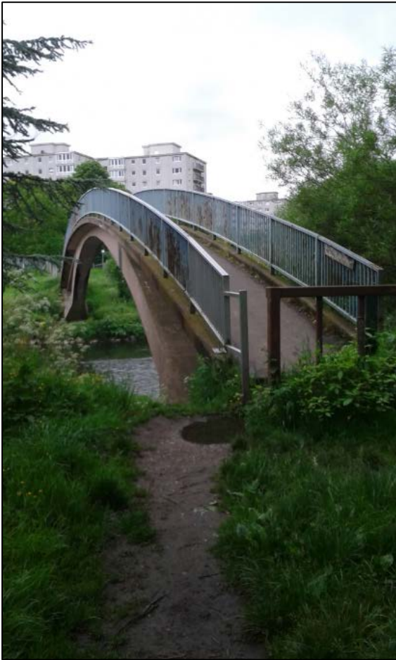
Figure 5.5 – Footbridge at the western entrance of Castle Irwell
