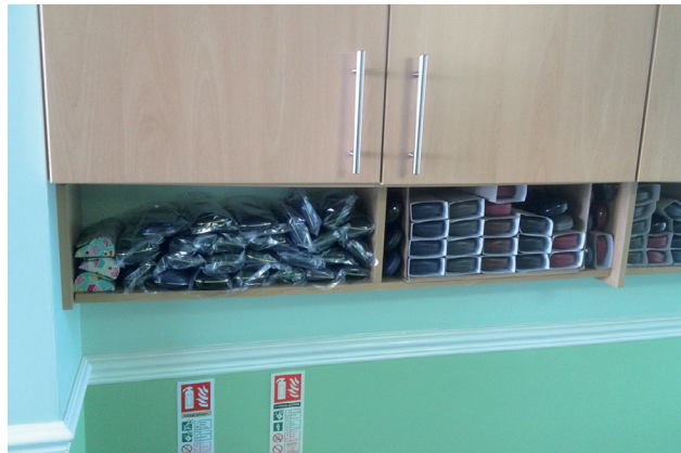
Figure 11: High value items raised above the previous flood height.
