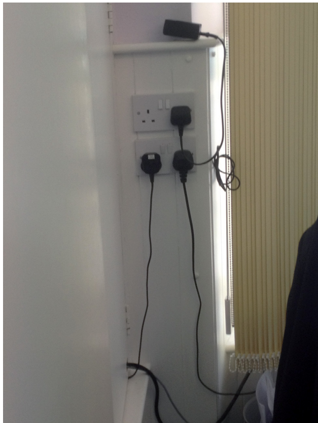
Figure 15: Raised wall sockets for safety.
