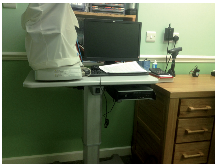
Figure 16: Cost significant items on height adjustable stands and height adjusted once perceived flood risk thresholds are reached.
