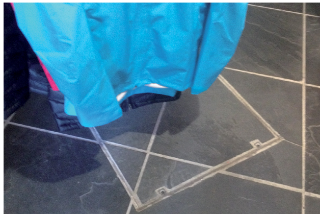
Figure 12: Firm fixing of an under floor drain that previously caused internal flooding.
