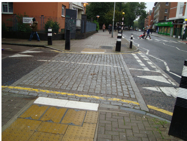
Figure 9. Tactile paving and sets are uncomfortable and can lead to imbalance
