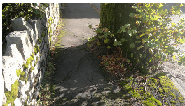
Figure 7. Bitumen surface made uneven by tree roots
