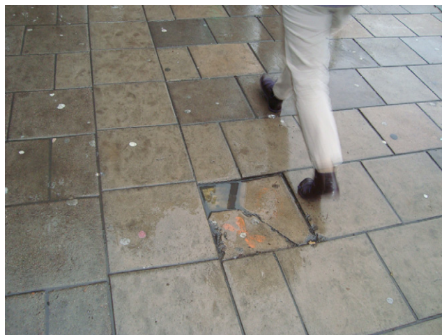
Figure 6. Cracked paving flag and wet conditions
