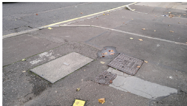
Figure 3. Changes in levels due to manhole covers
