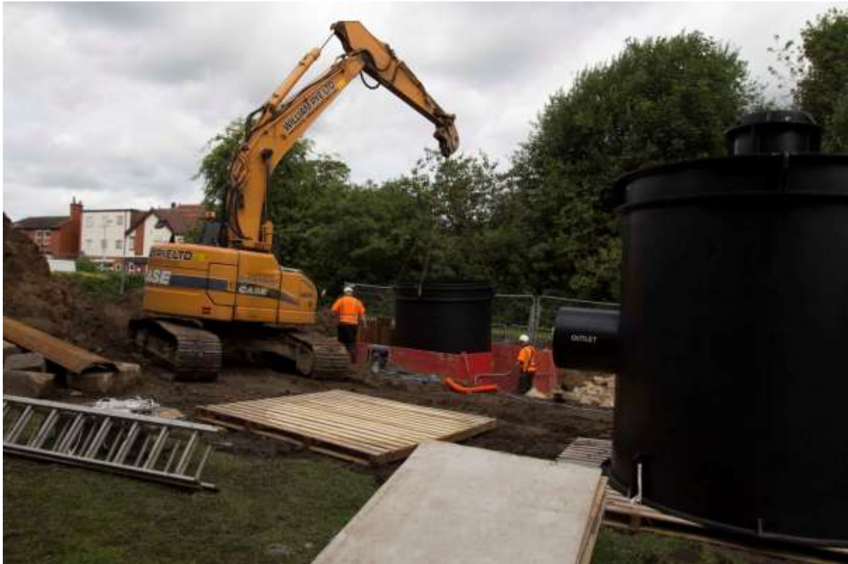
Figure 15 - DD Sump placement
