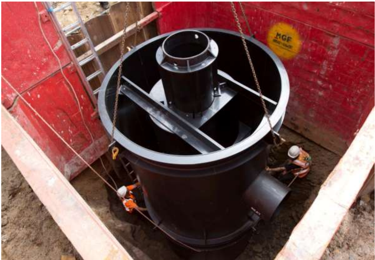
Figure 16 - DD being lowered in to place
