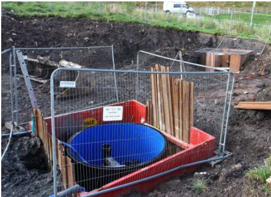
Figure 30 - X4 chamber (foreground) and upstream diversion manhole (background)
