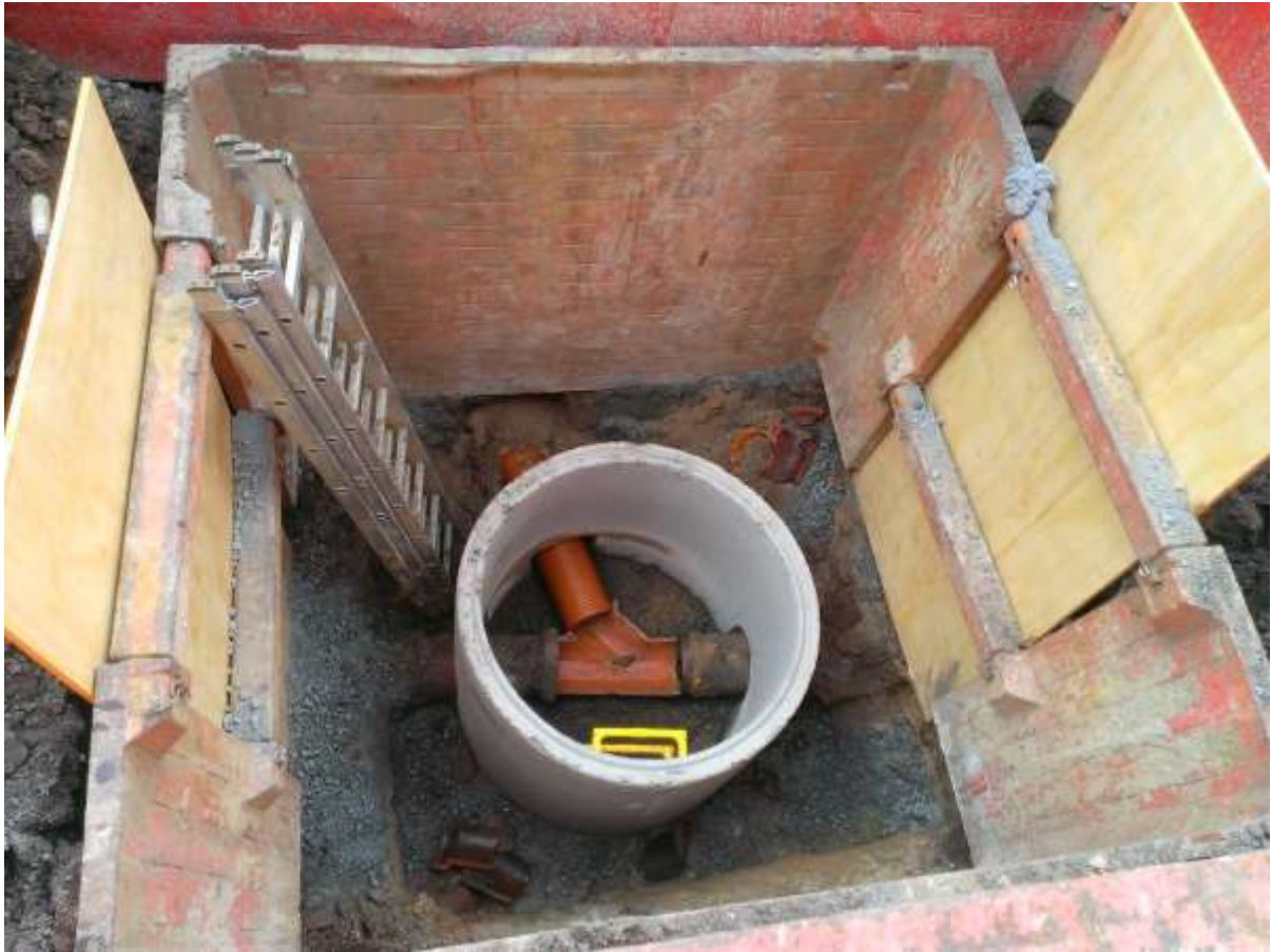
Figure 17 - Upstream Diversion chamber construction
