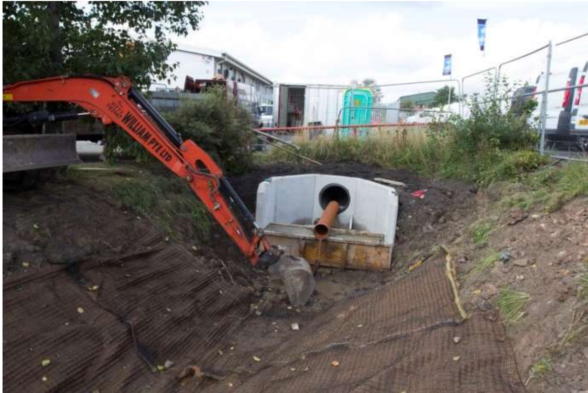
Figure 37 - View of the new wing wall
