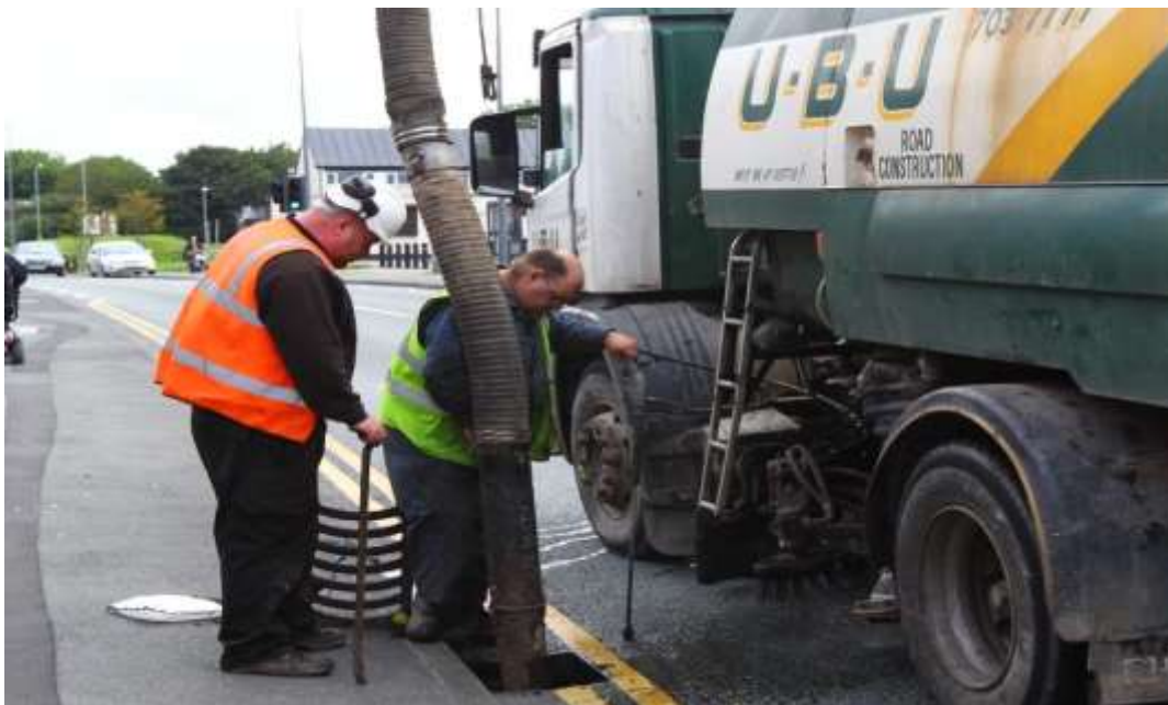
Figure 40 - Cleaning of the road gully prior to skimmer installation
