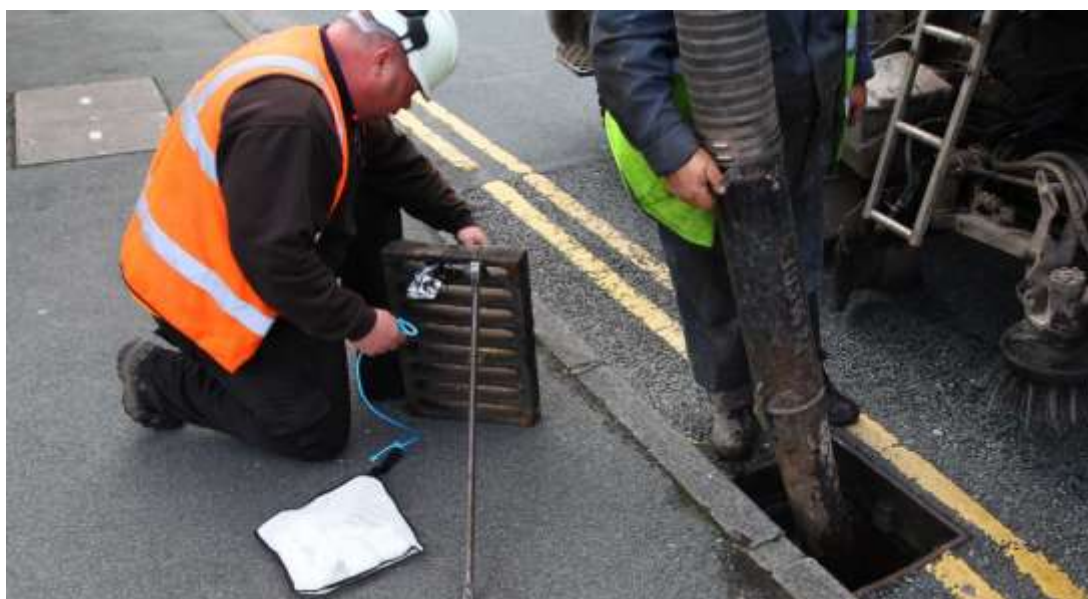
Figure 41 - Fixing of skimmer to manhole lid
