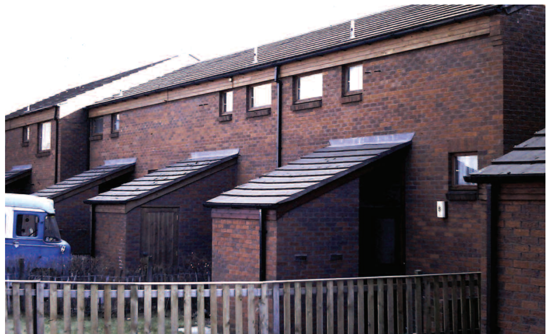
The NW facade of the prototype terrace in 1980 [3]
