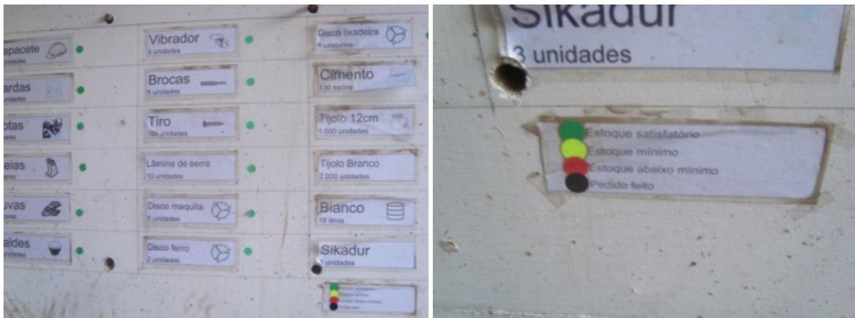
Figure 18-Material/consumables/hand tools stock control board on a construction site
