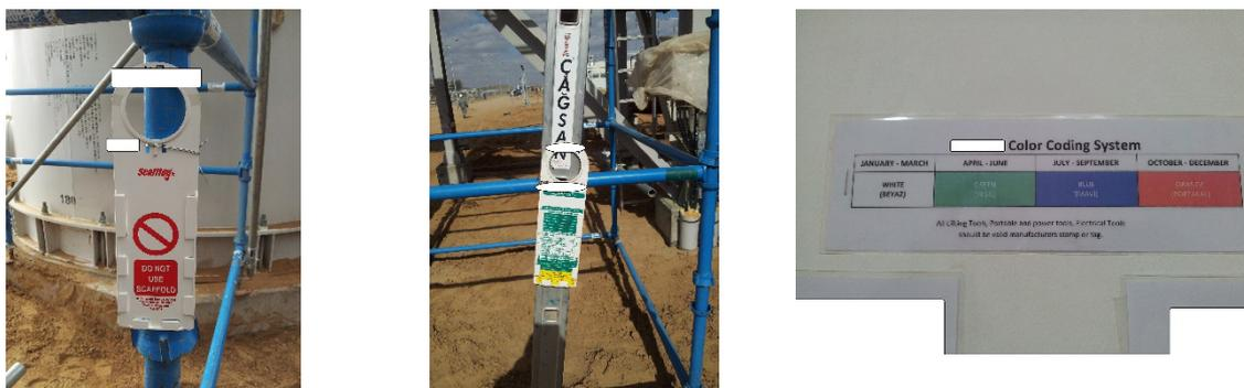
**Figure 34-Colour-coded safety tagging (adopted from Tezel et al., 2013)**
