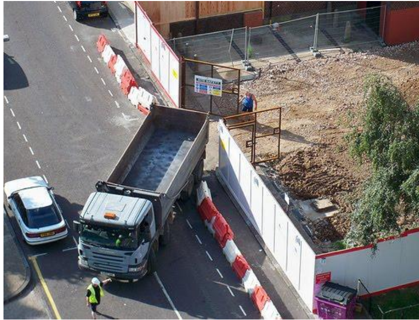
Figure 2-5: Loss of parking spaces due to manoeuvre space provided for the lorry (MERA, 2010)
