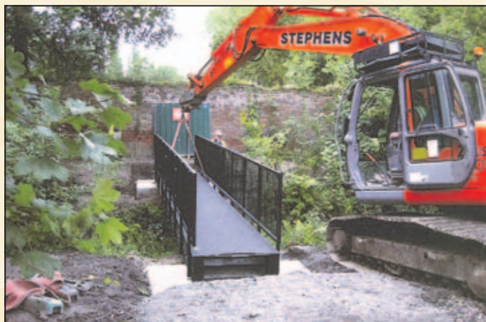
Lowering the new bridge over the moat into position in 2011
