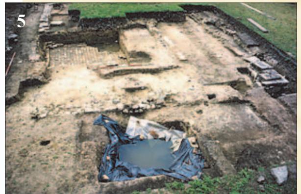
The stone and brick foundations of the eastern wing of the 17 th century ball looking south
