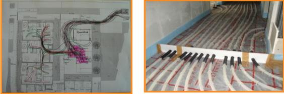
Figure C.2: Improvement of the floor heating installation process
