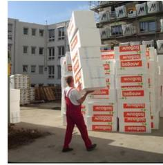
Figure 4.2(d): Storing large amounts of material onsite led to extra work for the construction workers who had to move it about
