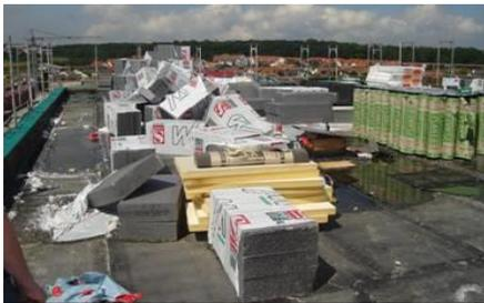
Figure 4.2(e): Material damaged after rainfall
