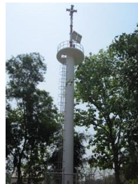
Automatic weather monitoring station, detected rainfall amount by the solar radiation, located in Wat Santi Wiharn temple
