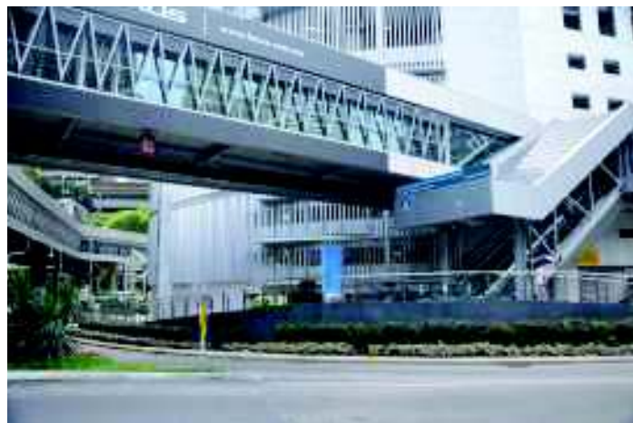
Figure 3. 30 Elevated walkways connecting KL Convention Centre and Pavilion Mall
