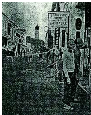
Figure 3. 8 A street scene in the Old Town Kuala Lumpur in 1900 (Tate et al., 1987)
