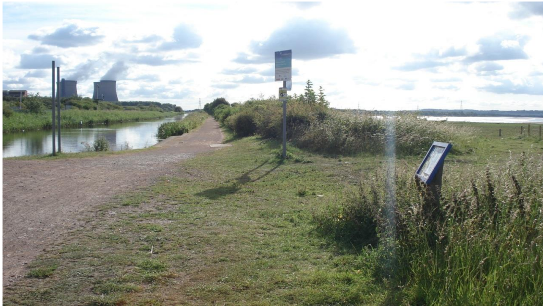
Figure 38: View towards Fiddlers Ferry approach from the main viewing area. Grazing area to the right.
