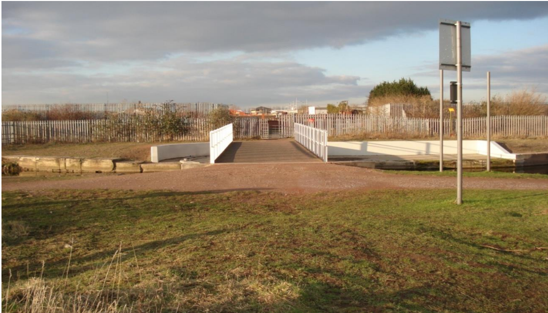
Figure 40: View towards the Tan House Lane approach from the main viewing area.
