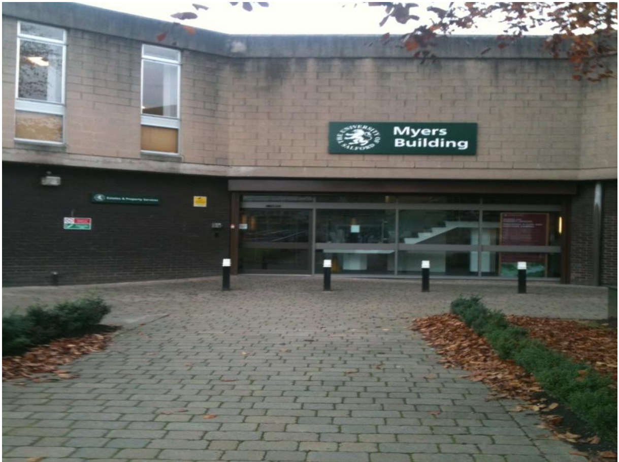
Figure 64 One of the University buildings where change was implemented.
