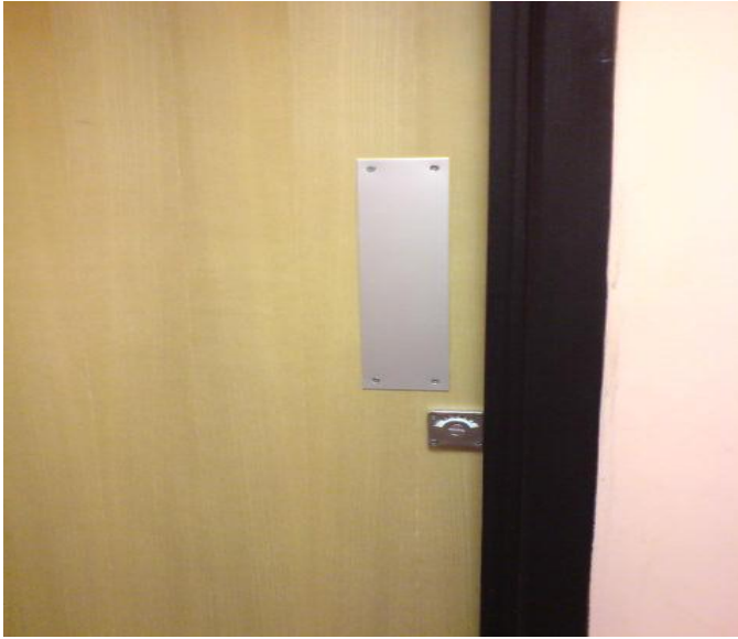
Figure 7 Door with a vertical metal plate
