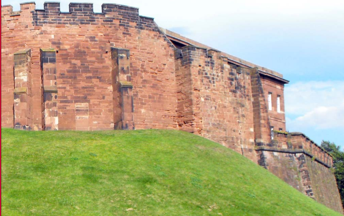
Fig 1: Chester Castle, showing the later medieval curtain wall standing on top of the motte erected in 1070 on King William's orders.
