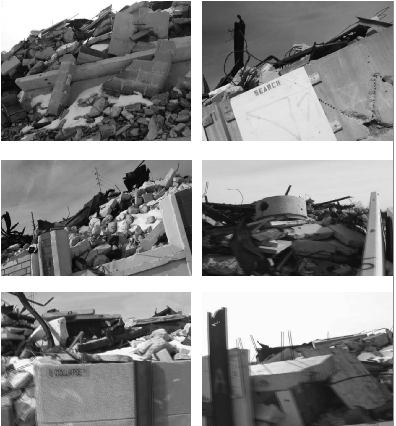
Fig. 11. Video frames and still photographs captured during initial building damage reconnaissance operation undertaken on mobility platform: (a) top — photo capture while riding; (b) lower — video frames captured while riding
