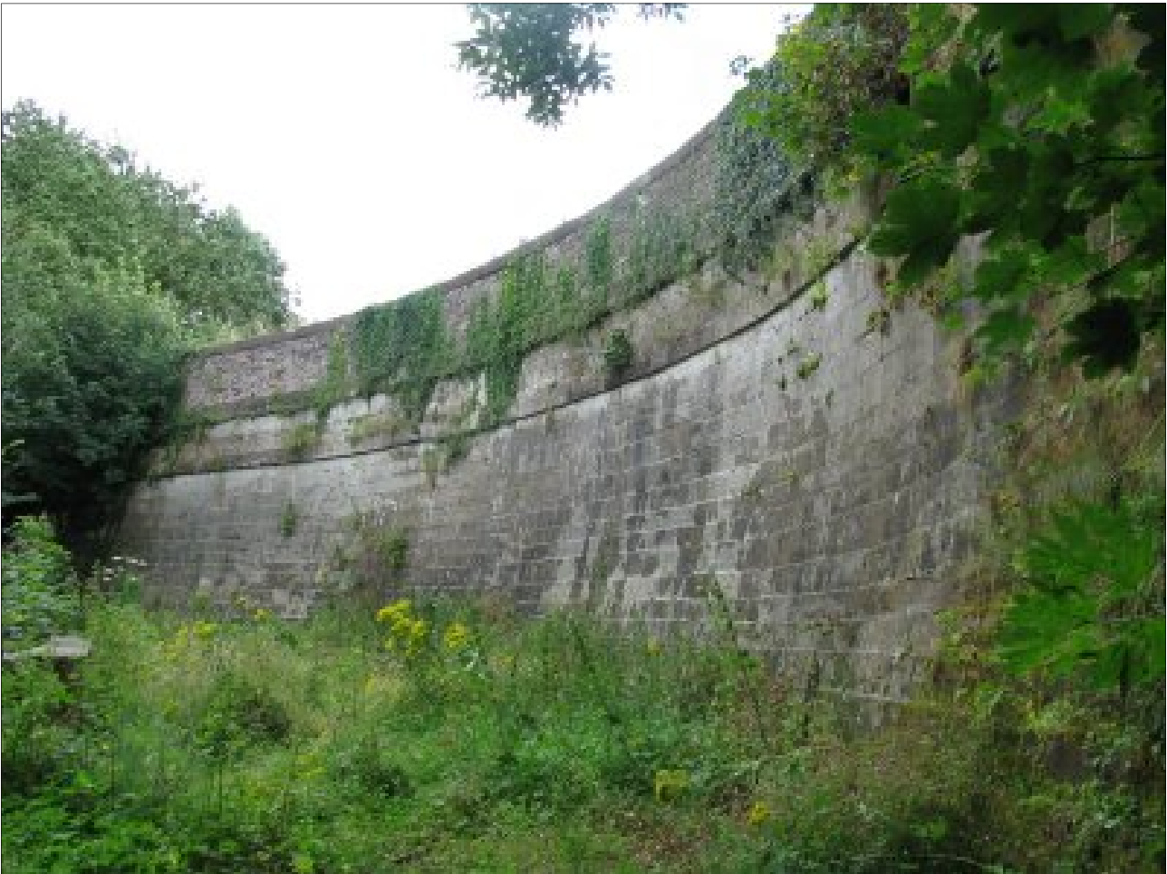
Fig 10.5: The north-western curved retaining wall for the Bollin aqueduct (copyright MRLAS).
