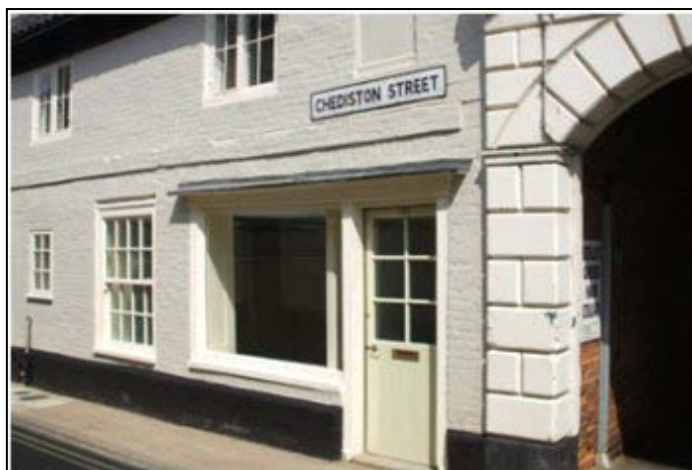
The adjoining building now houses 2 affordable homes and a retail unit (©FE)
