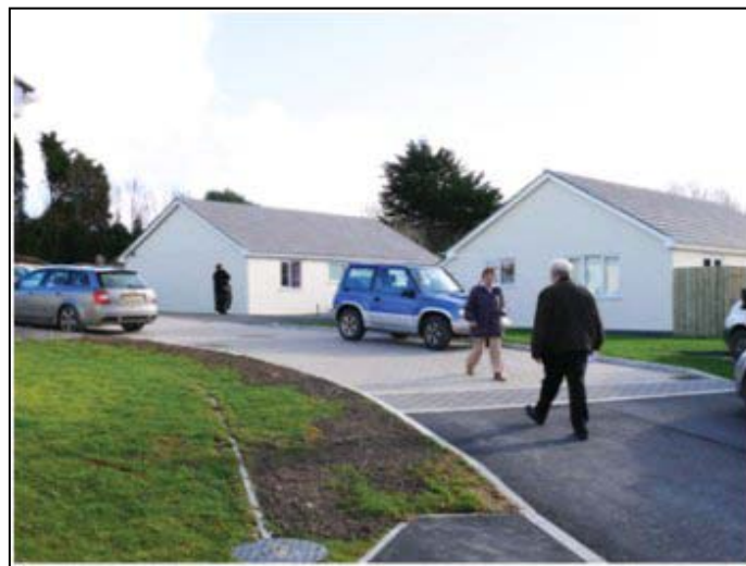
Completed homes at St Minver (©CLT Network)
