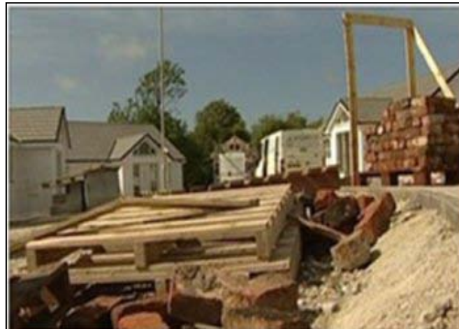
Saint Minver under construction (©BBC)
