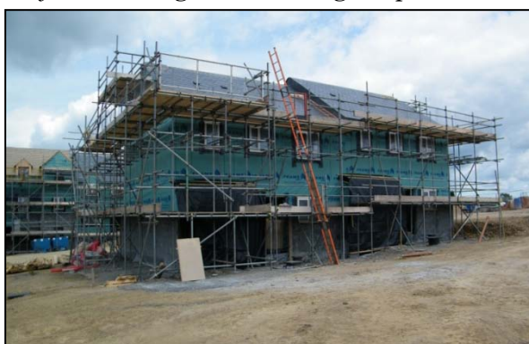
Current work on Little Bickington Farm Development (©HBCPT)
