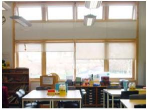
Figure 19: Small windows at the top, allowing ventilation without draught (Rolls Crescent Primary School, Manchester, UK - Confirmatory Case)
