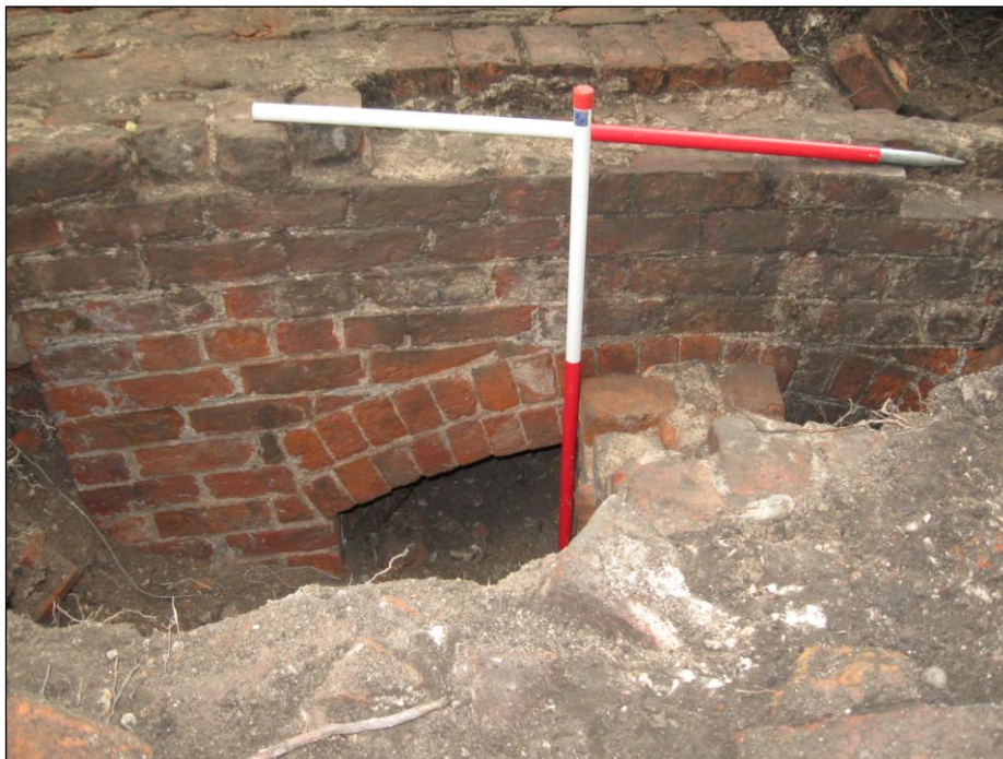
CG-10 Plate 12: Interior face of wall (106) showing segmental arch and abutting wall (107). Looking south.
