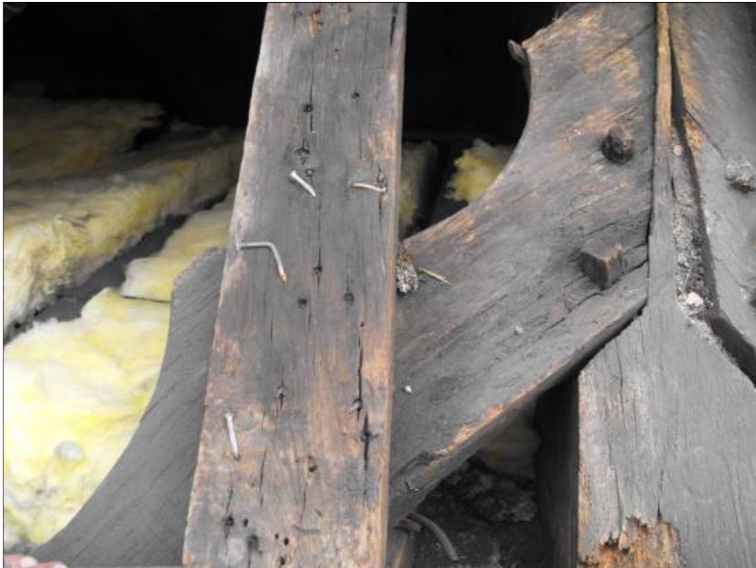
Fig 3: Detail of the scalloped-decorated wind-brace on the southern side of the fourth truss.
