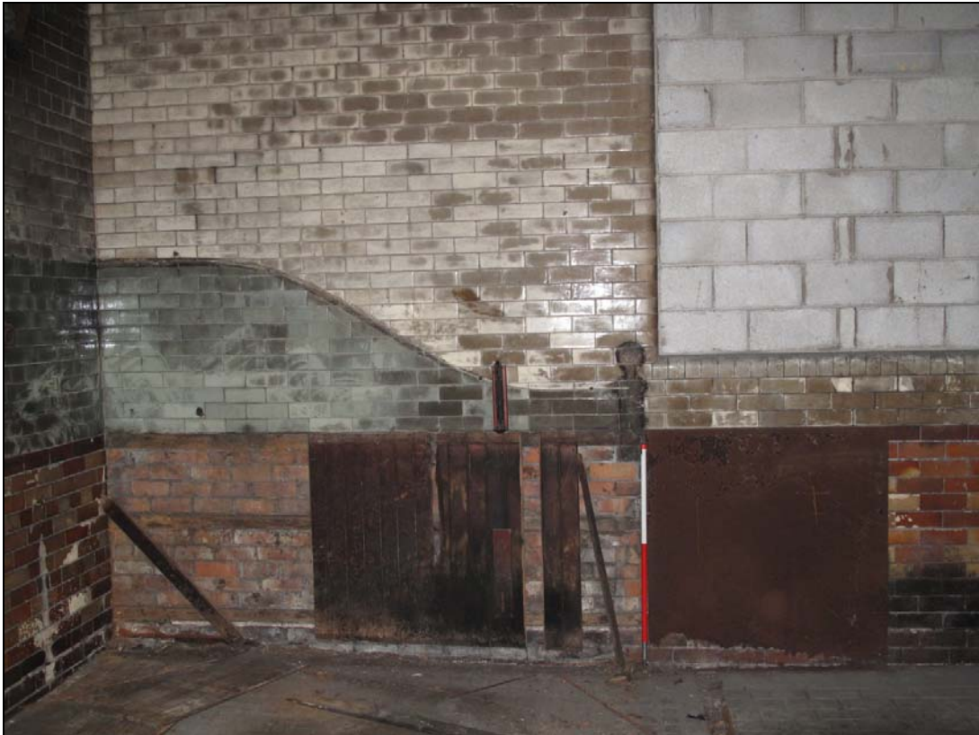
Fig 62: 1GFc showing the 'ghost' outline of horse box partitioning on the western elevation wall.
