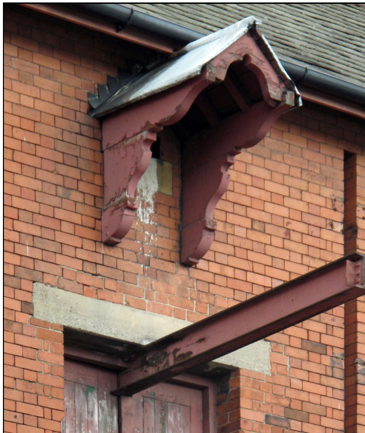
Fig 54: Similar as 21; detail of the original hoist timber rooflet.
