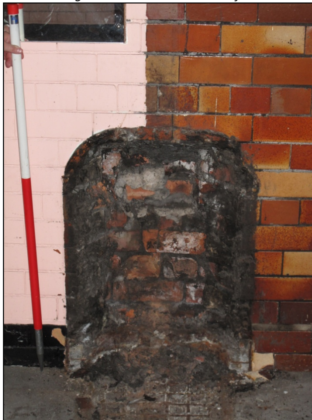
Fig 58: Similar as 57 detail of shallow fireplace central to the northern dividing wall.
