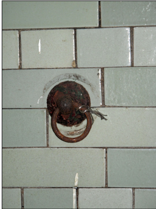
Fig 60: Similar as 85 detail of cast iron tie-ring on southern dividing wall.
