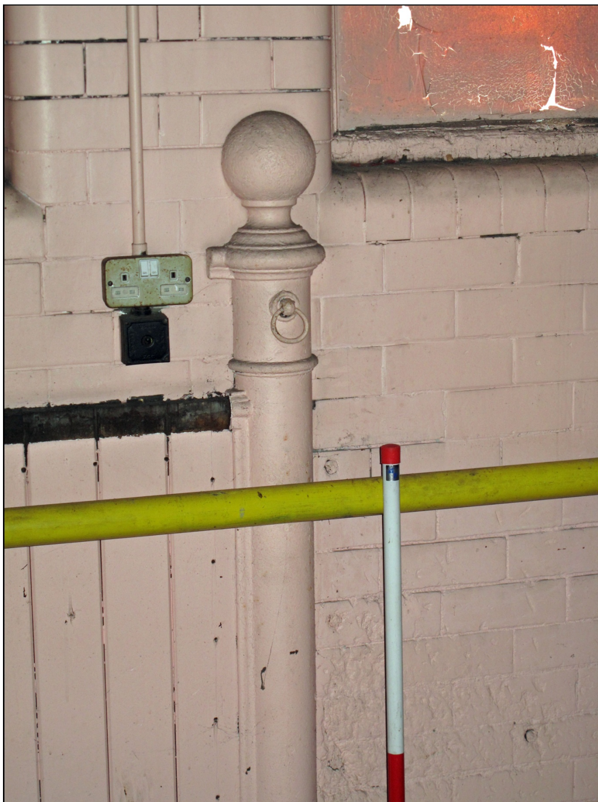
Fig 59: Similar as 57; cast iron horse stall post at S. End of the W. Elev., wall.
