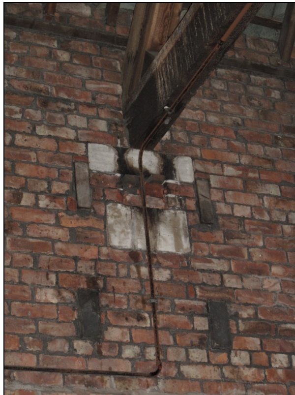
Fig 78: Similar as 131; detail of blocked opening for the original timber hoist arm.
