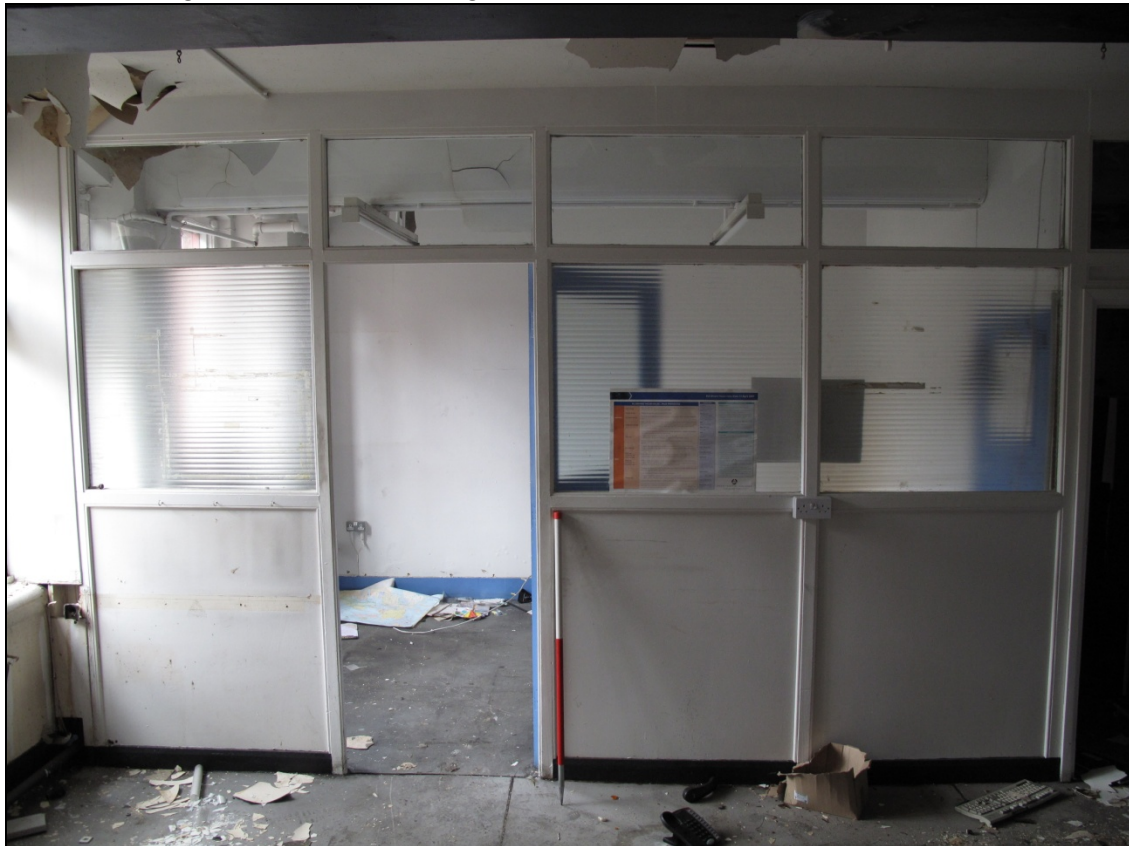
Fig 37: GF1 area 'e' showing glazed office partitions to the N end.
