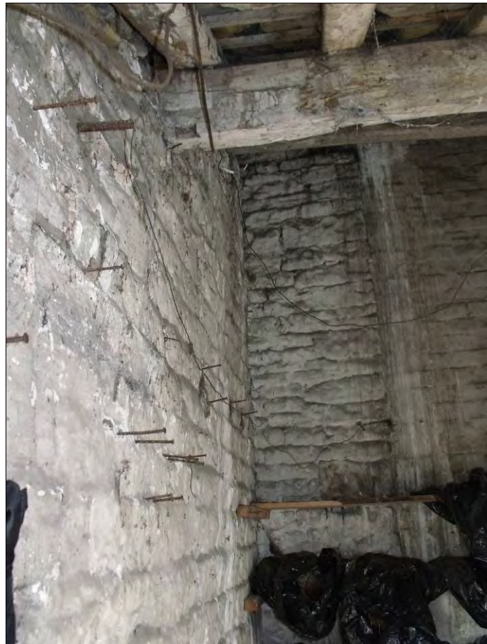
Fig 38: Room G5 looking north-westwards at the watershot stone partition with room G3, which was a former gable wall.
