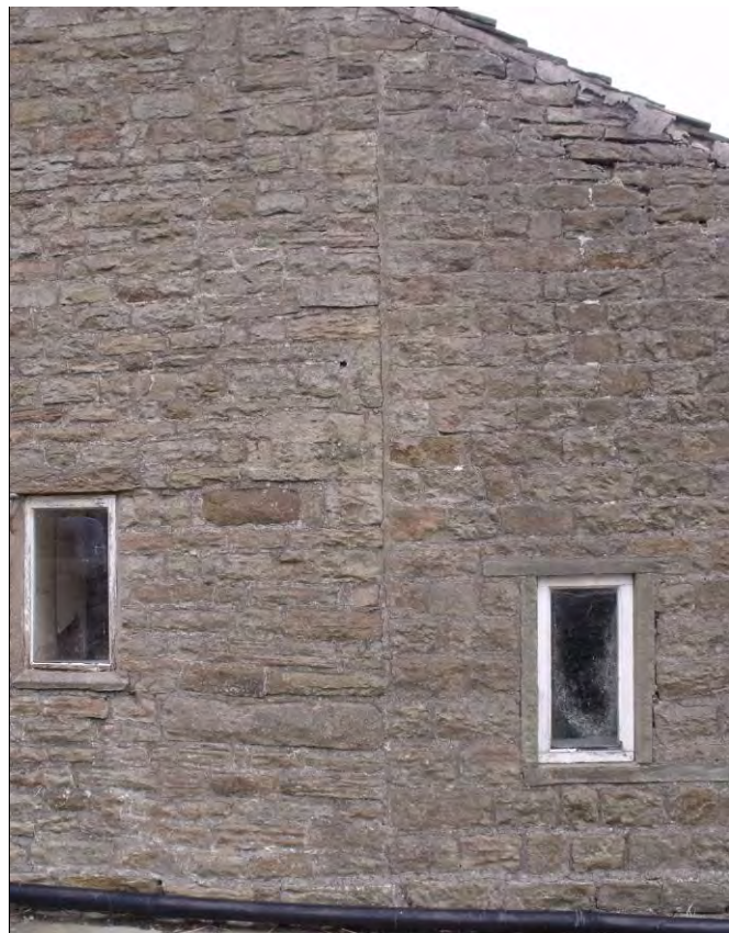
Fig 16: detail of the western gable of 35 Barnsfold Road showing the break at the south-west corner
