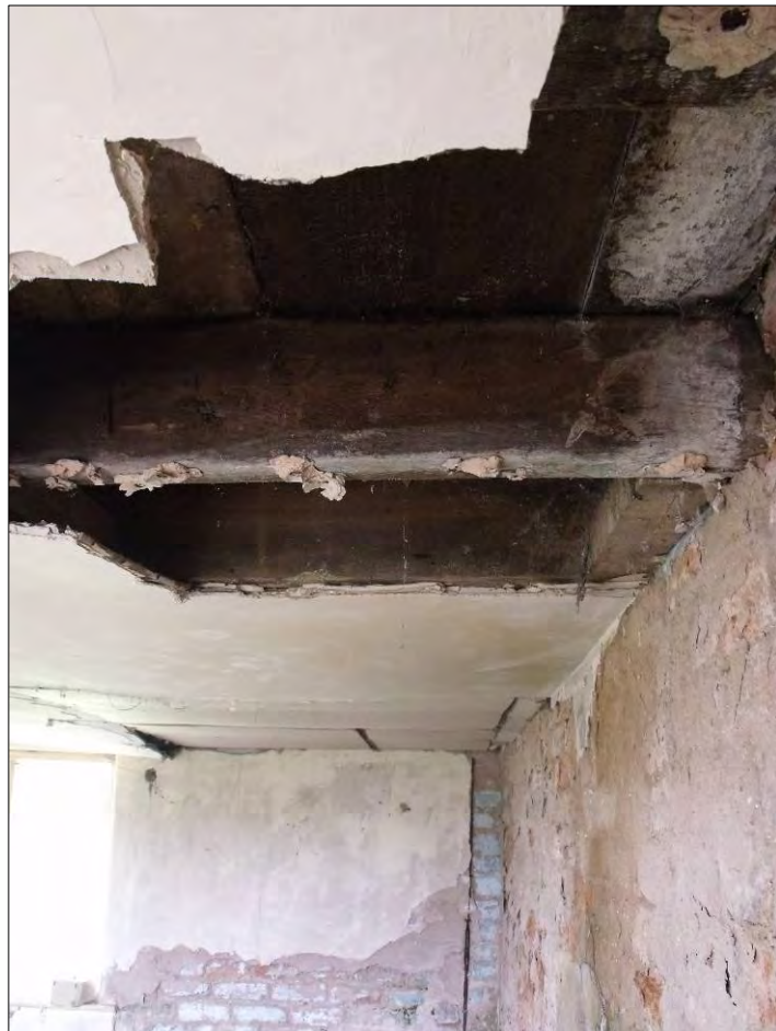
Fig 21: Detail of the ceiling joists along the western wall of room G1.
