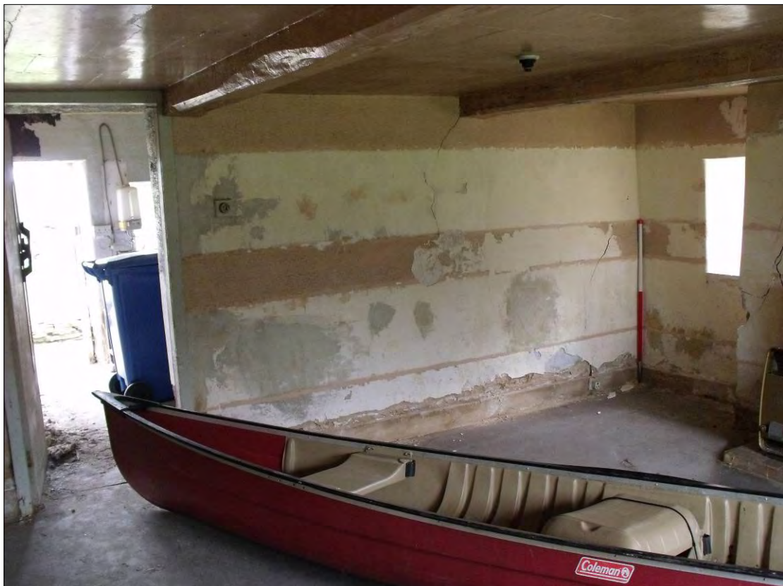
Fig 30: Room G2 looking southwards towards the kitchen area, room G3. Note the chamfered ceiling beams.
