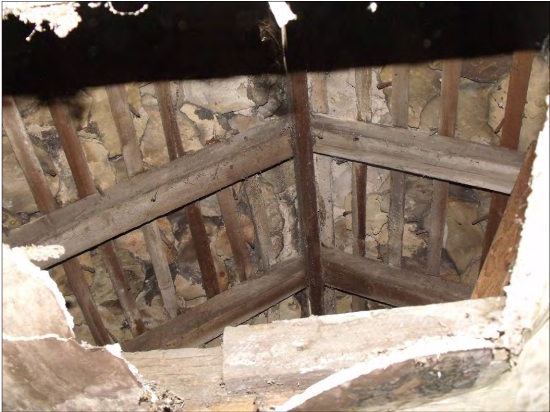
Fig50: Detail of the roof structure (machine-cut pine rafters) above room FF2.
