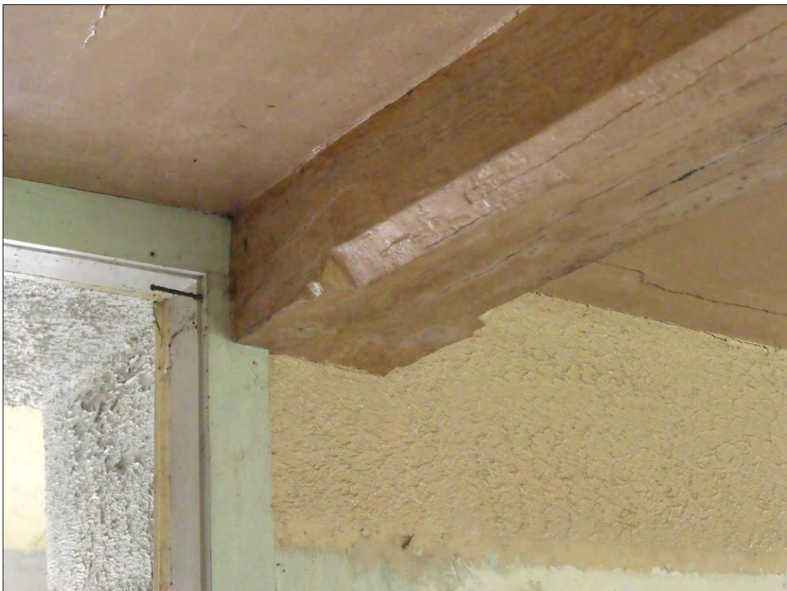
Fig 28: Room G2 looking at the southern end of the eastern ceiling beam. Note the deep chamfering and run out stops.
