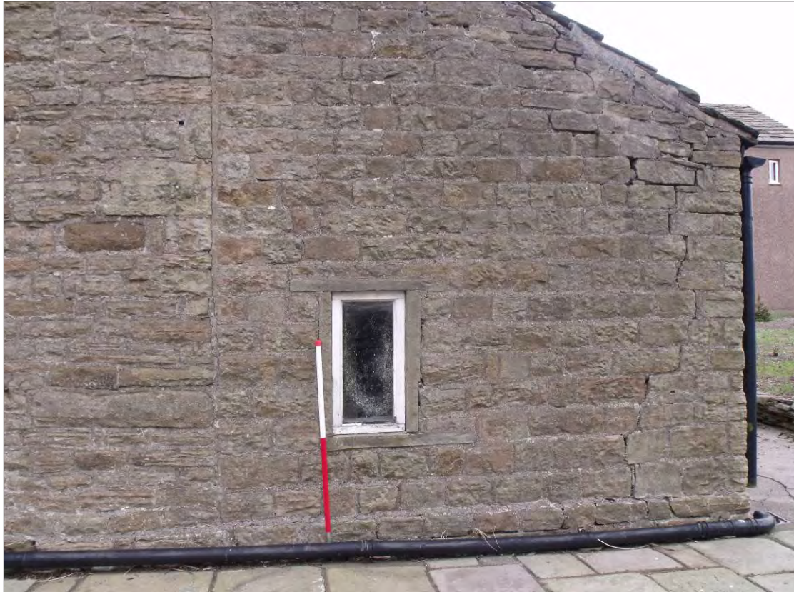
Fig 16: detail of the western gable of 35 Barnsfold Road showing the break at the south-west corner
