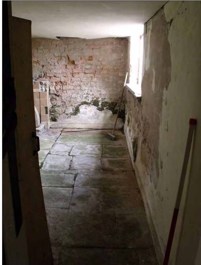
Fig 20: Detail of room G1 looking along the southern wall. Note the brickwork and the flag-flooring.
