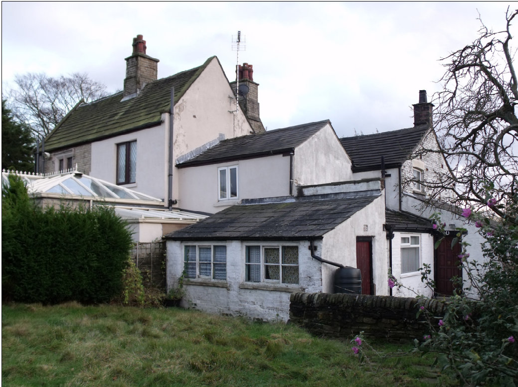
Fig 3: The eastern and northern elevations of Gothic Farm Cottage.
