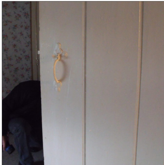
Fig 7: The hand-forged handle to the plank and baton door in FF4.
