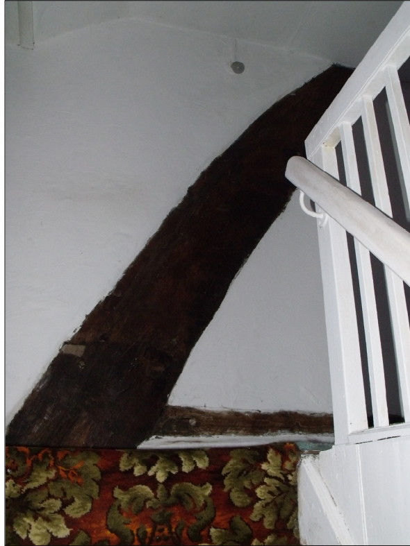
Fig 8: The western cruck blade in the landing area FF1 looking east.
