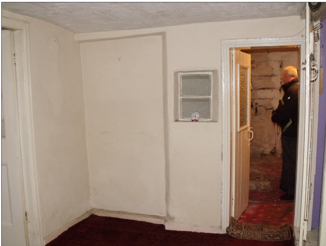
Fig 5: The blocked doorway and earlier window in G2, looking south.
