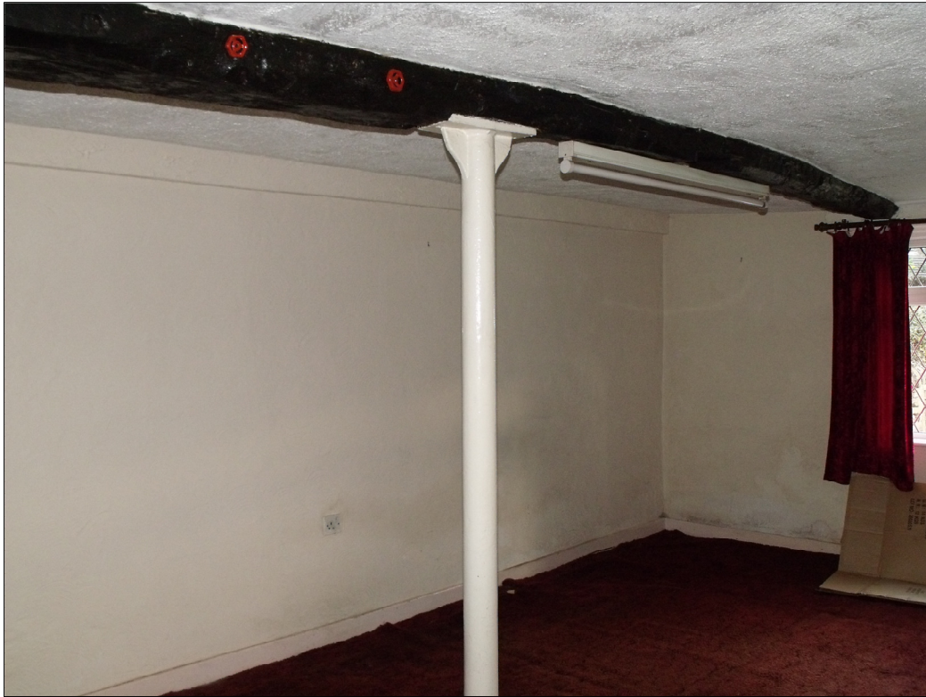
Fig 4: The transverse beam and cast-iron column in G3 looking south.
