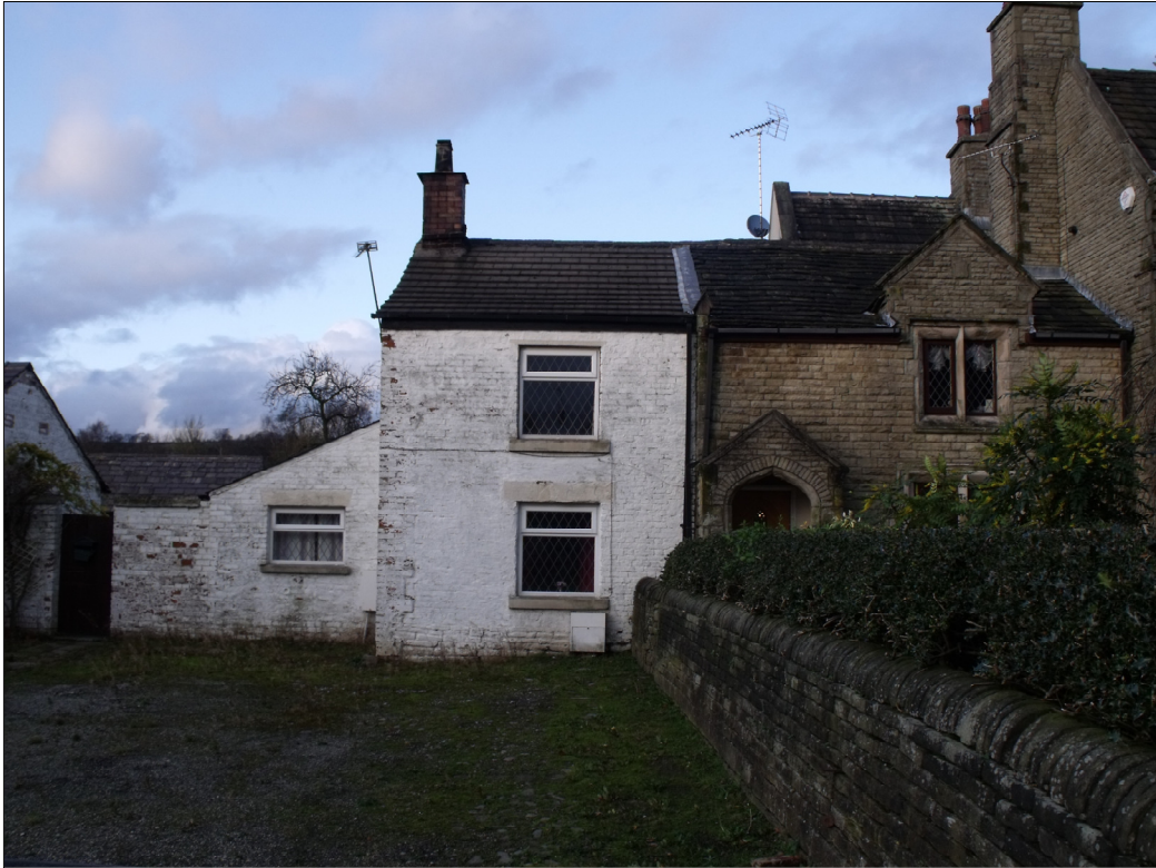
Fig 2: The southern elevation of Gothic Farm Cottage (the white brick building).
