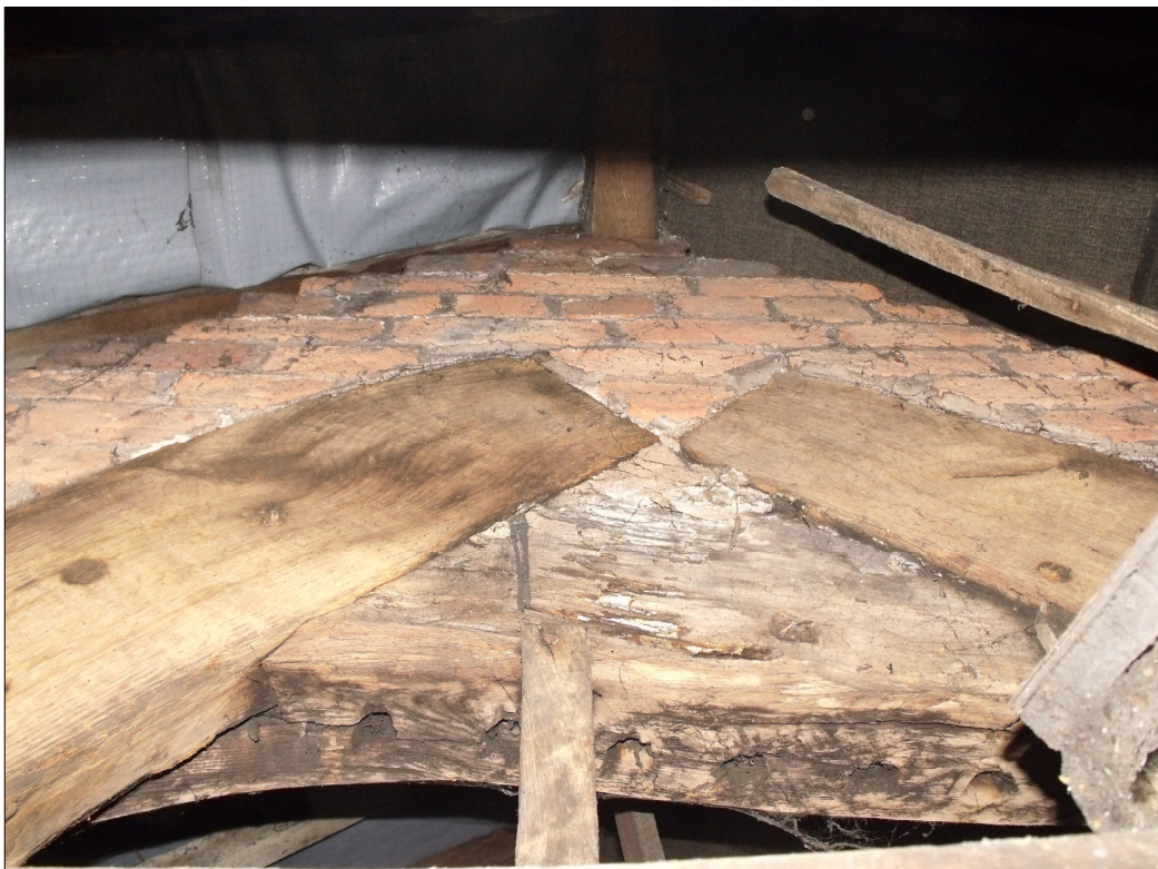
Fig 9: A detail of the apex form of the cruck truss in the roof space above FF1.
