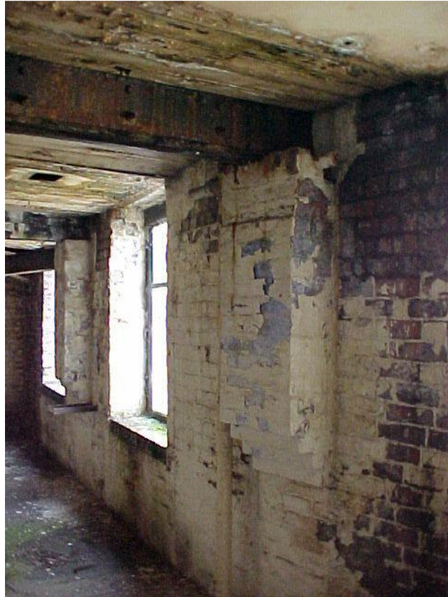
Figure 31. Detail shot of corbelled brick support for RSJ beam, third floor
