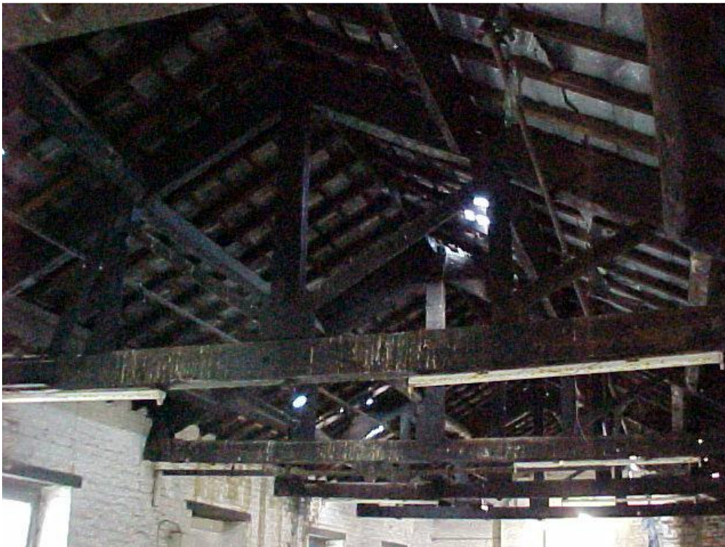
Figure 34. Detail of kingpost trusses, fourth floor
