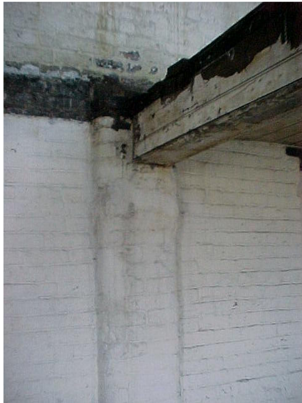
Figure 30. Detail shot of pilaster and beam between third and fourth floors
