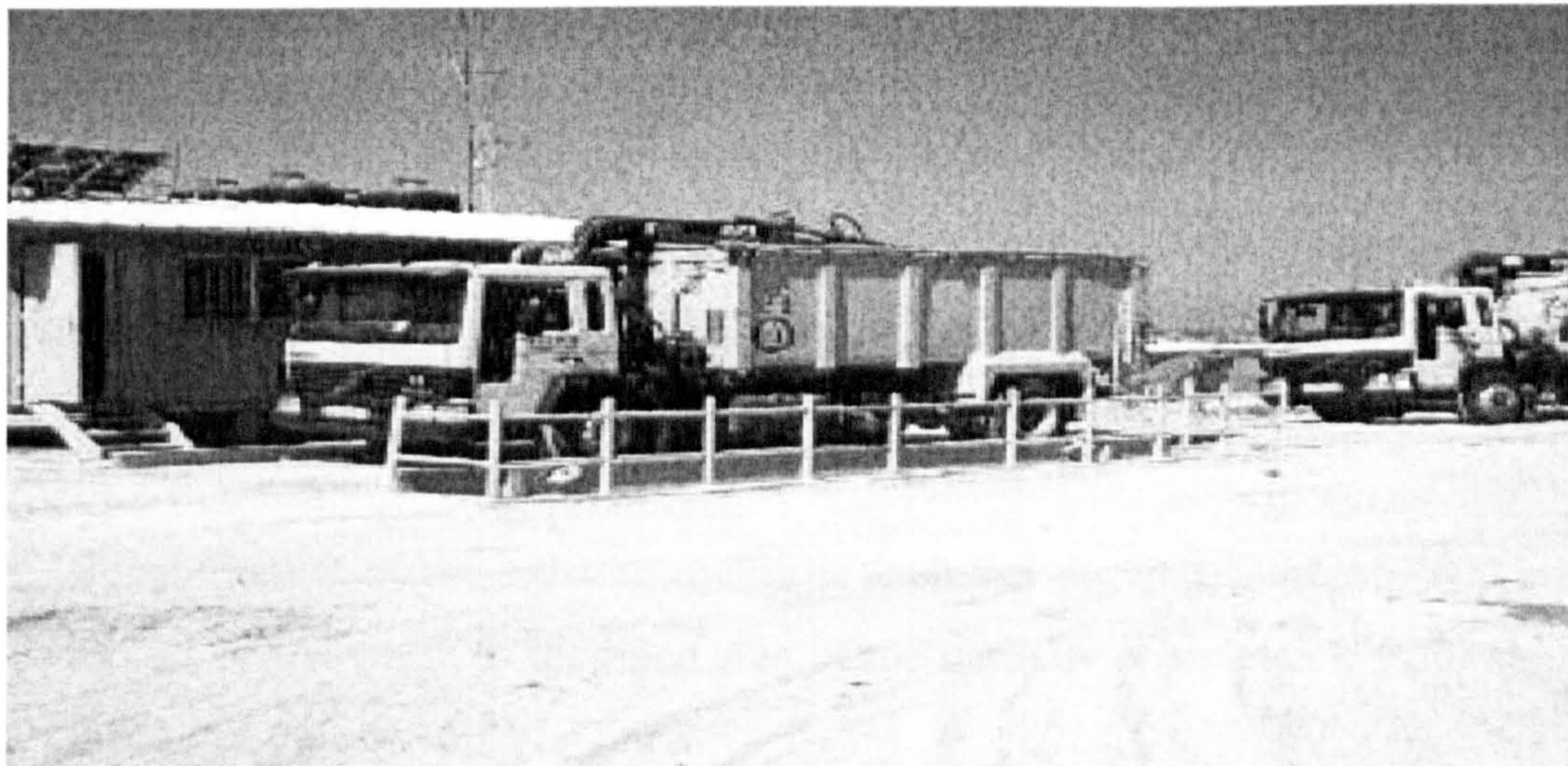
Photo 7.2: Access control. The structure for the site office is based standard shipping containers, and the electricity for the weighbridge and computer is generated by solar panels
