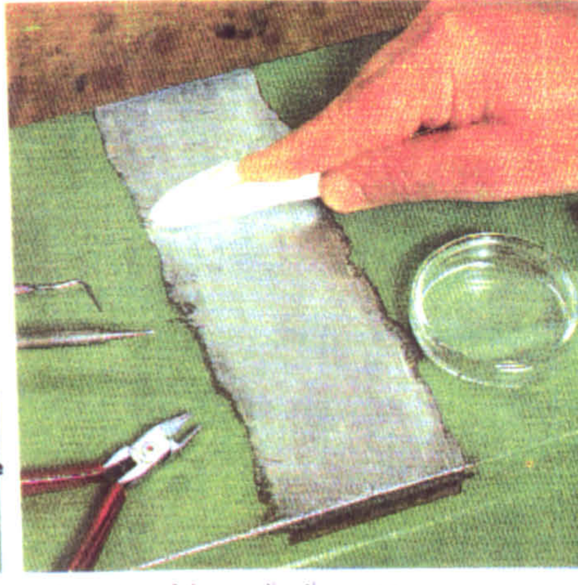
2. Cleaning of the application area
