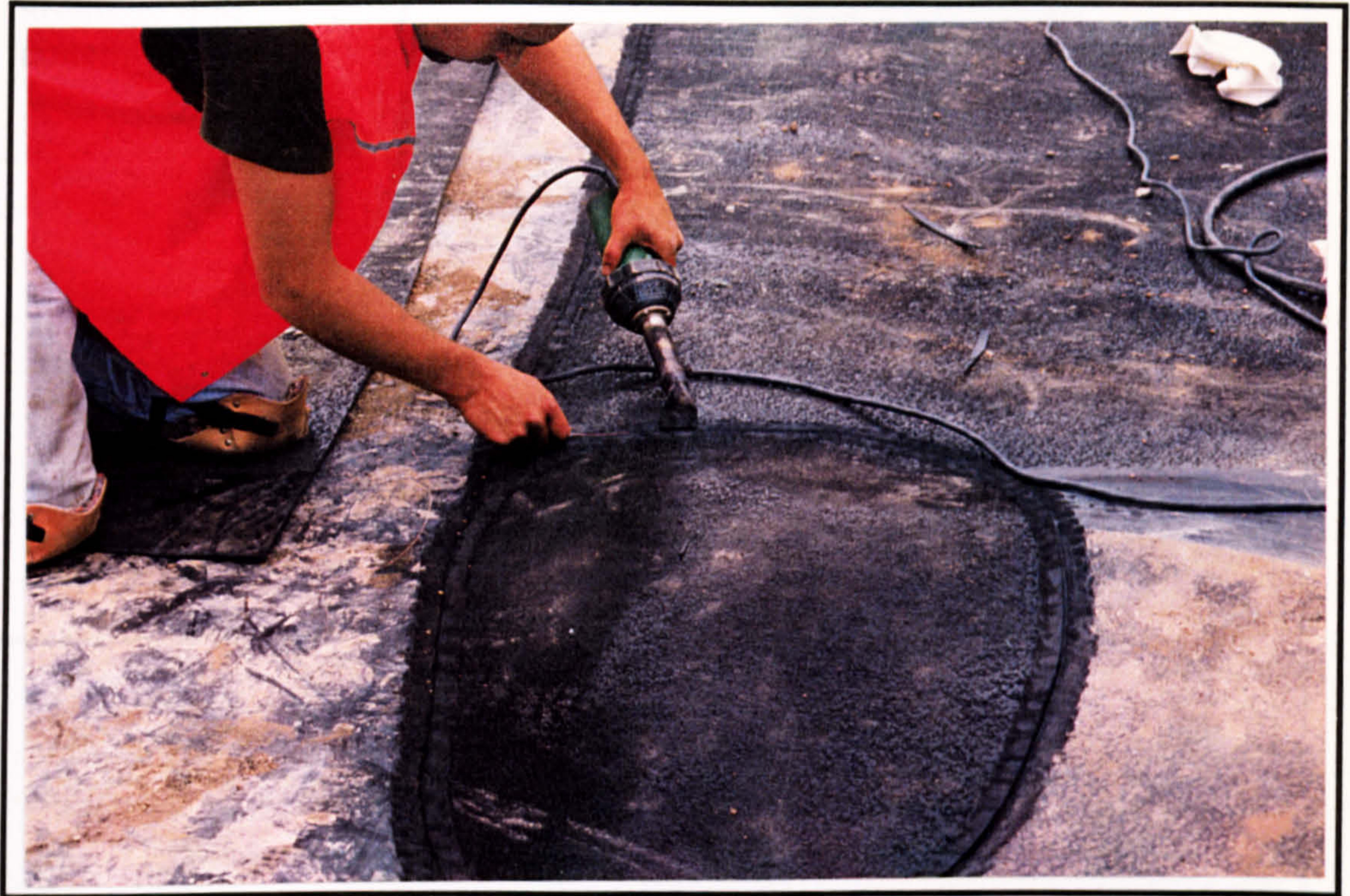
Plate 1-5: Sealing special wire in between the HDPE liner joints
