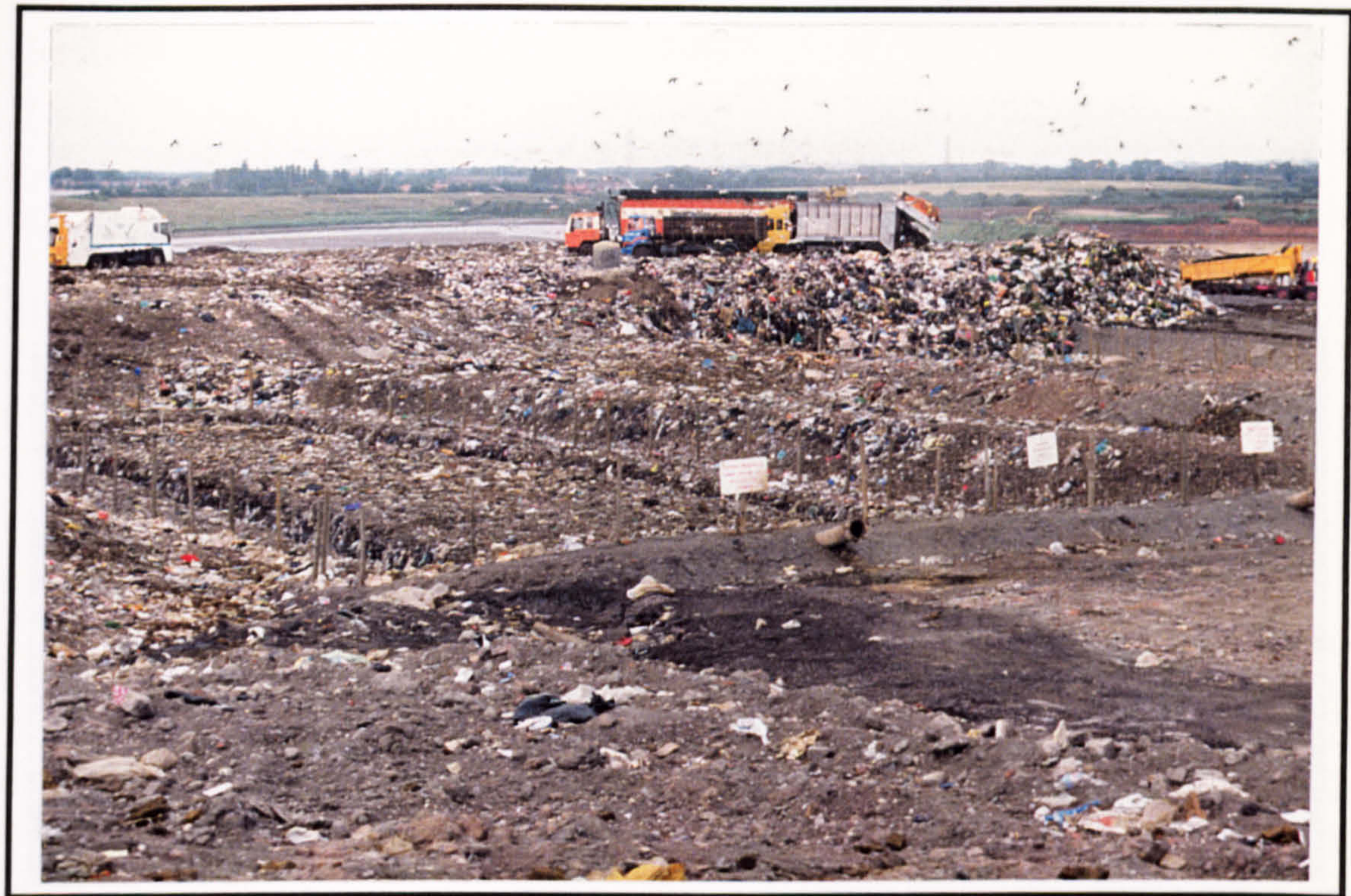
Plate 1-11: Filling of wastes in progress and encroaching towards the co-disposal pits
