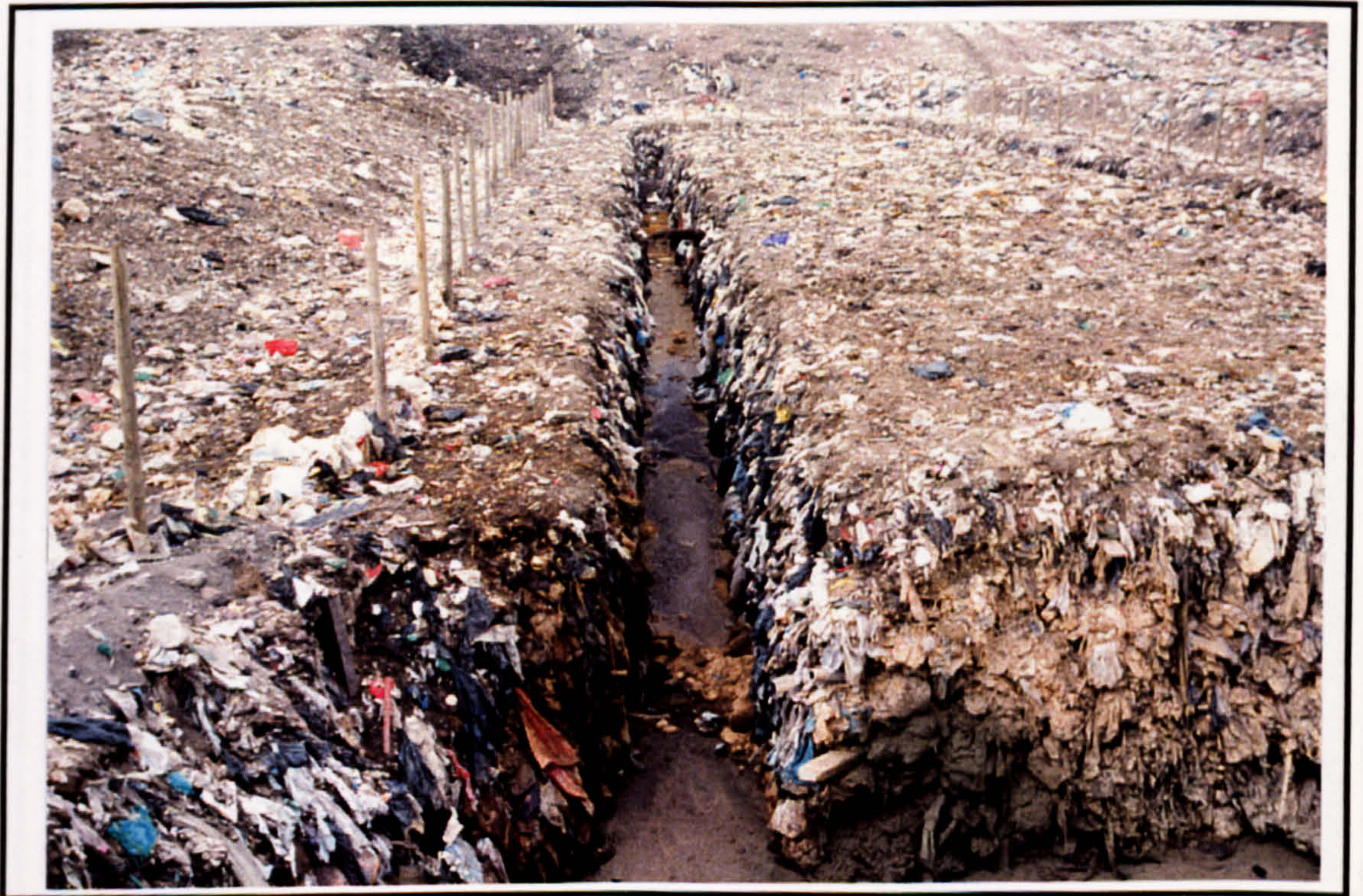
Plate 1-14: The sludge or liquid wastes is distributed to other area in the pit by interconnecting drains
