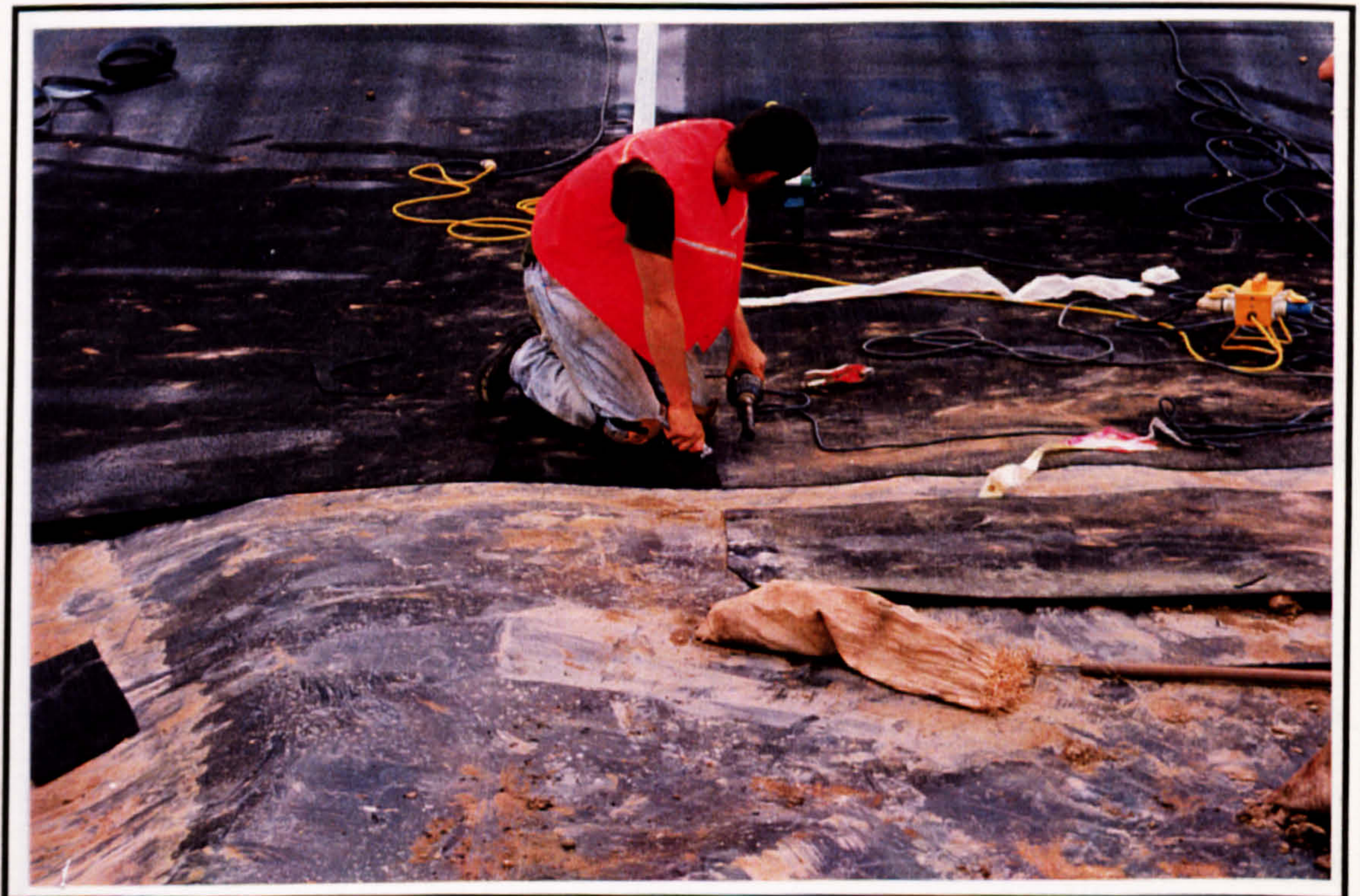
Plate 1-4: Joining work on the High Density Polyethylene Liner (HDPE)
