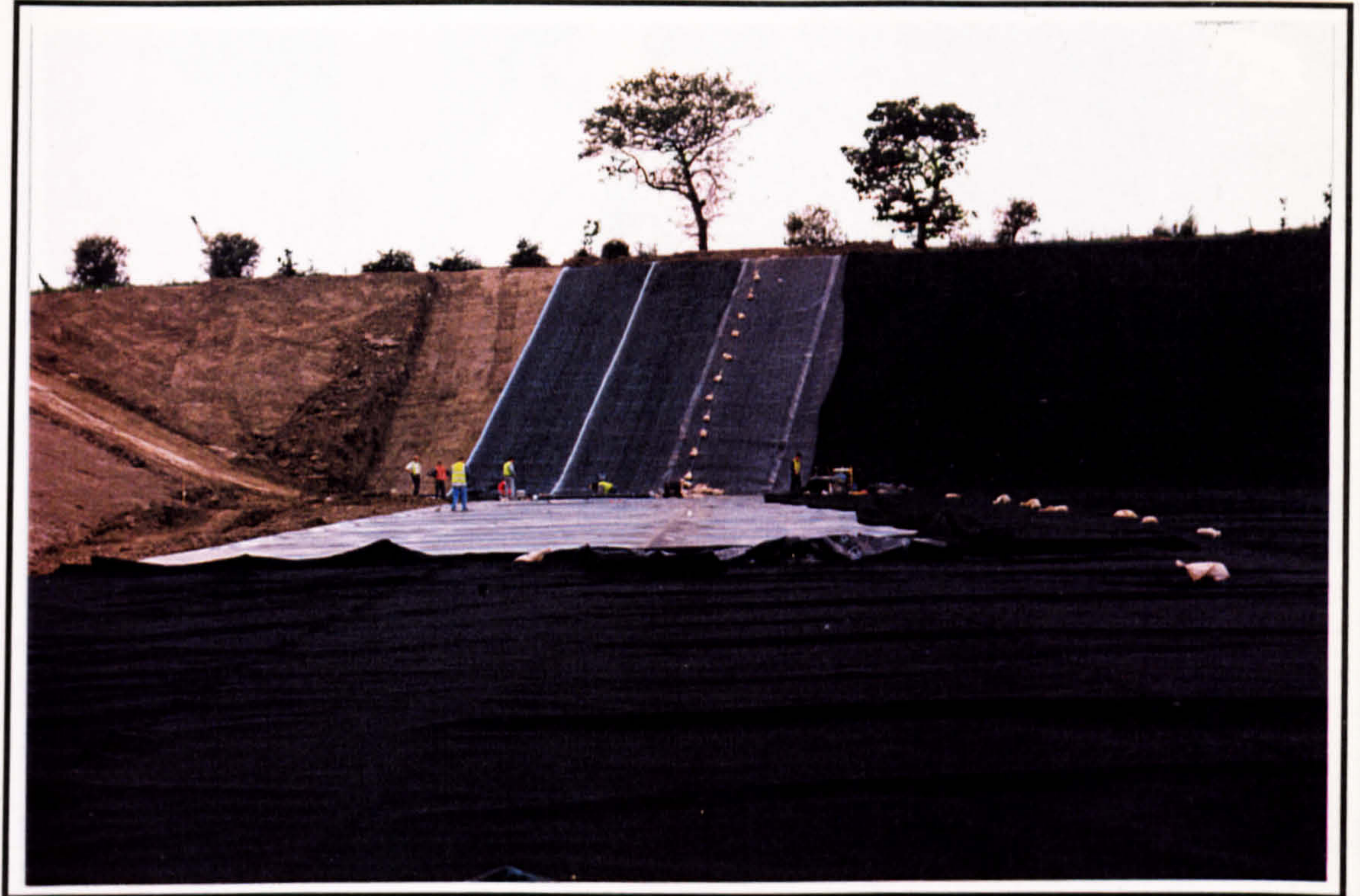
Plate 1-3: Layering of High Density Polyethylene Liner (HDPE)
