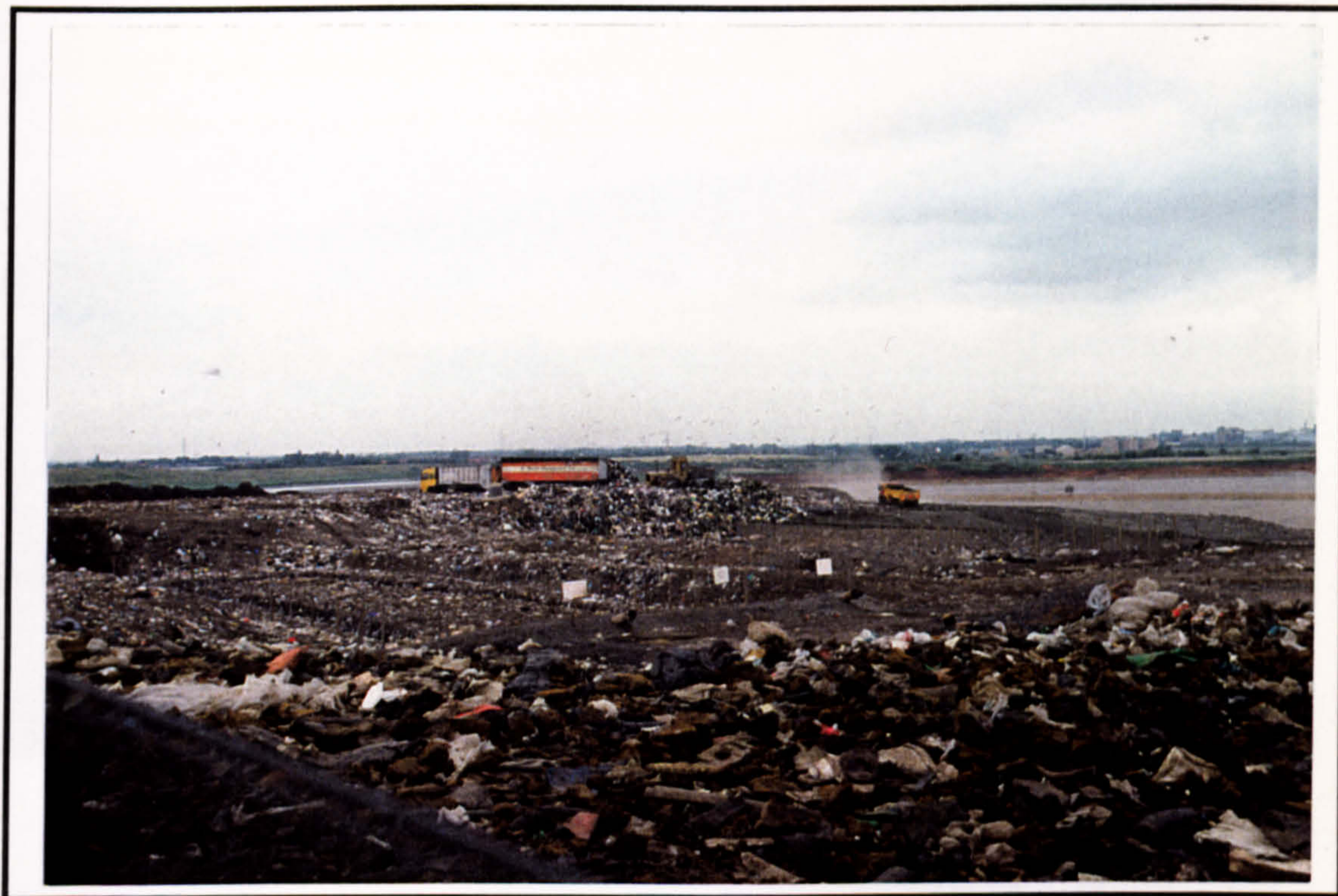
Plate 1-15: Fore view shows inert materials are used to cover the upper most layer of the filled waste
