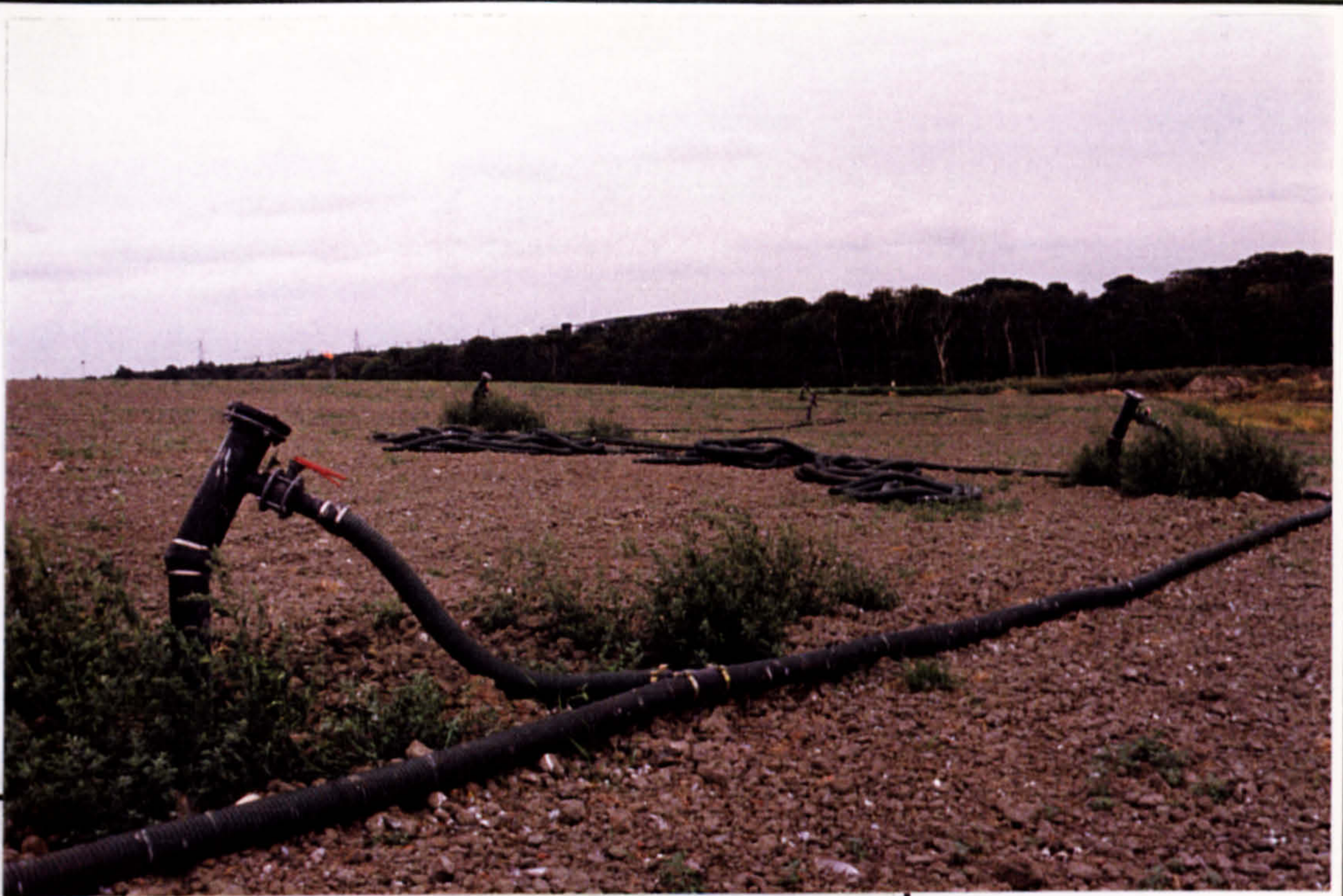
Plate 1-17: System of interconnecting pipes collecting methane
