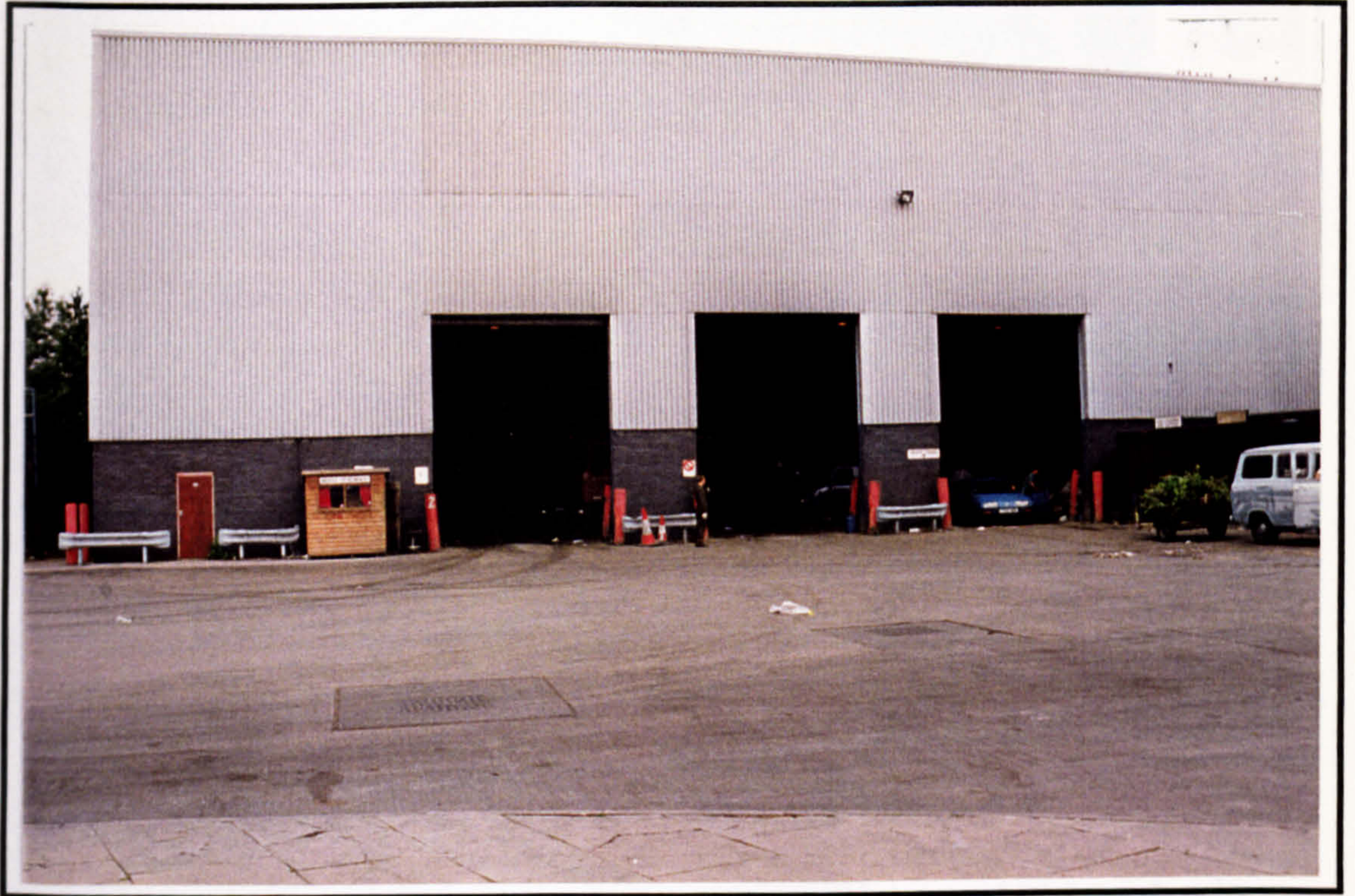
Plate 2-1: Main entrance to the reception hall
