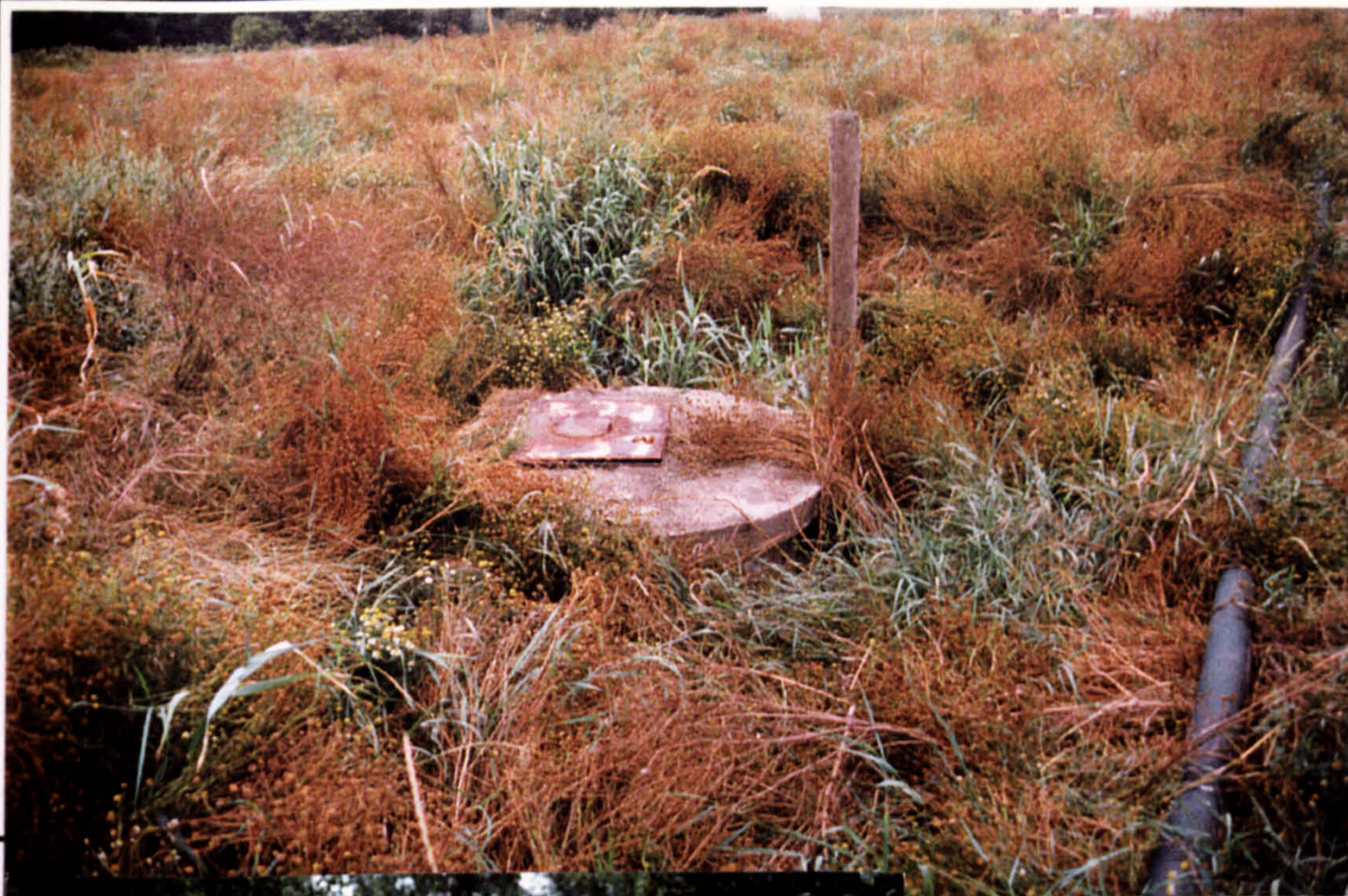
Plate 1-19: Leachate collecting well securely covered
