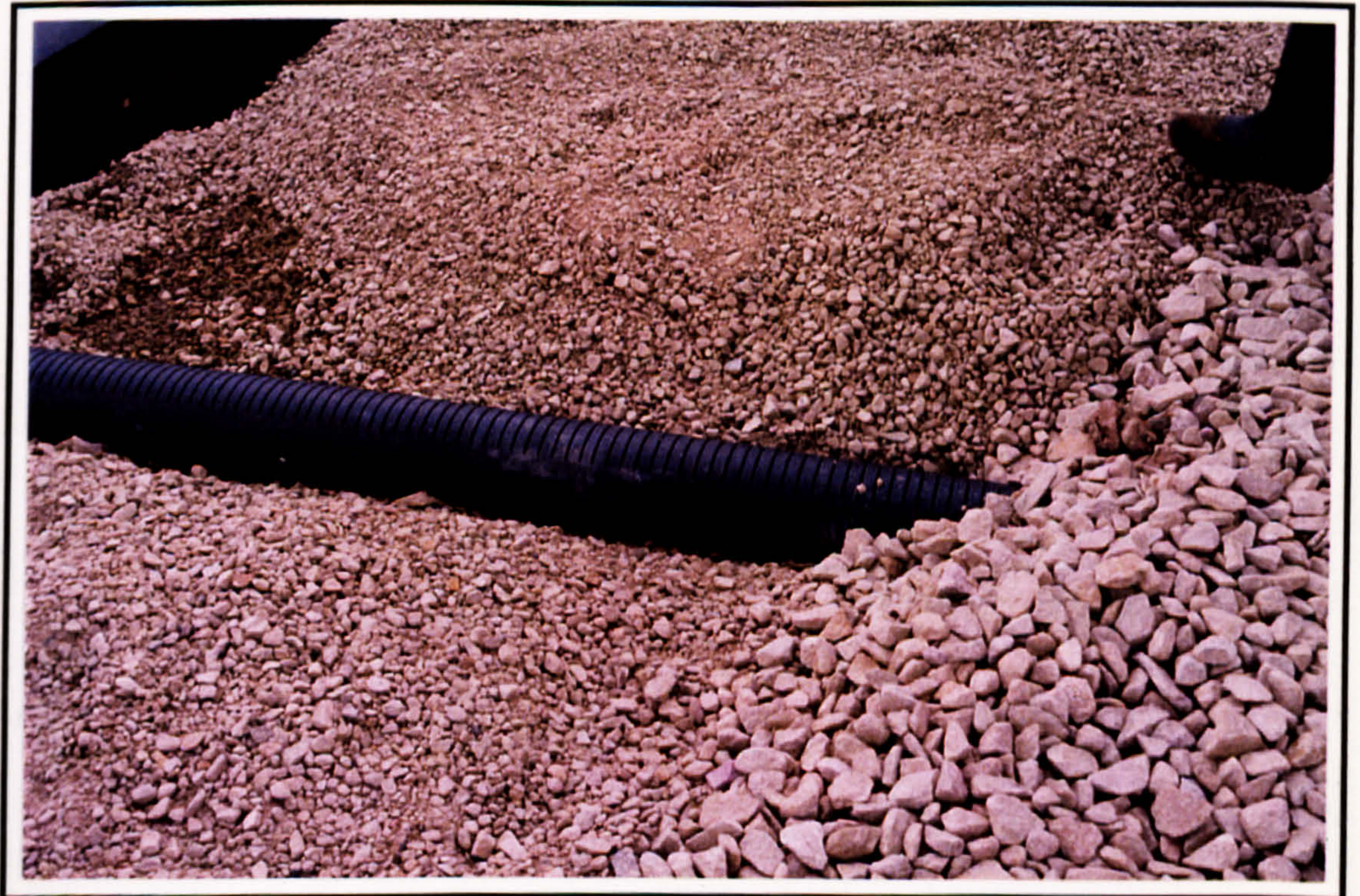
Plate 1-2: Layering of aggregates and leachate drainage pipe
