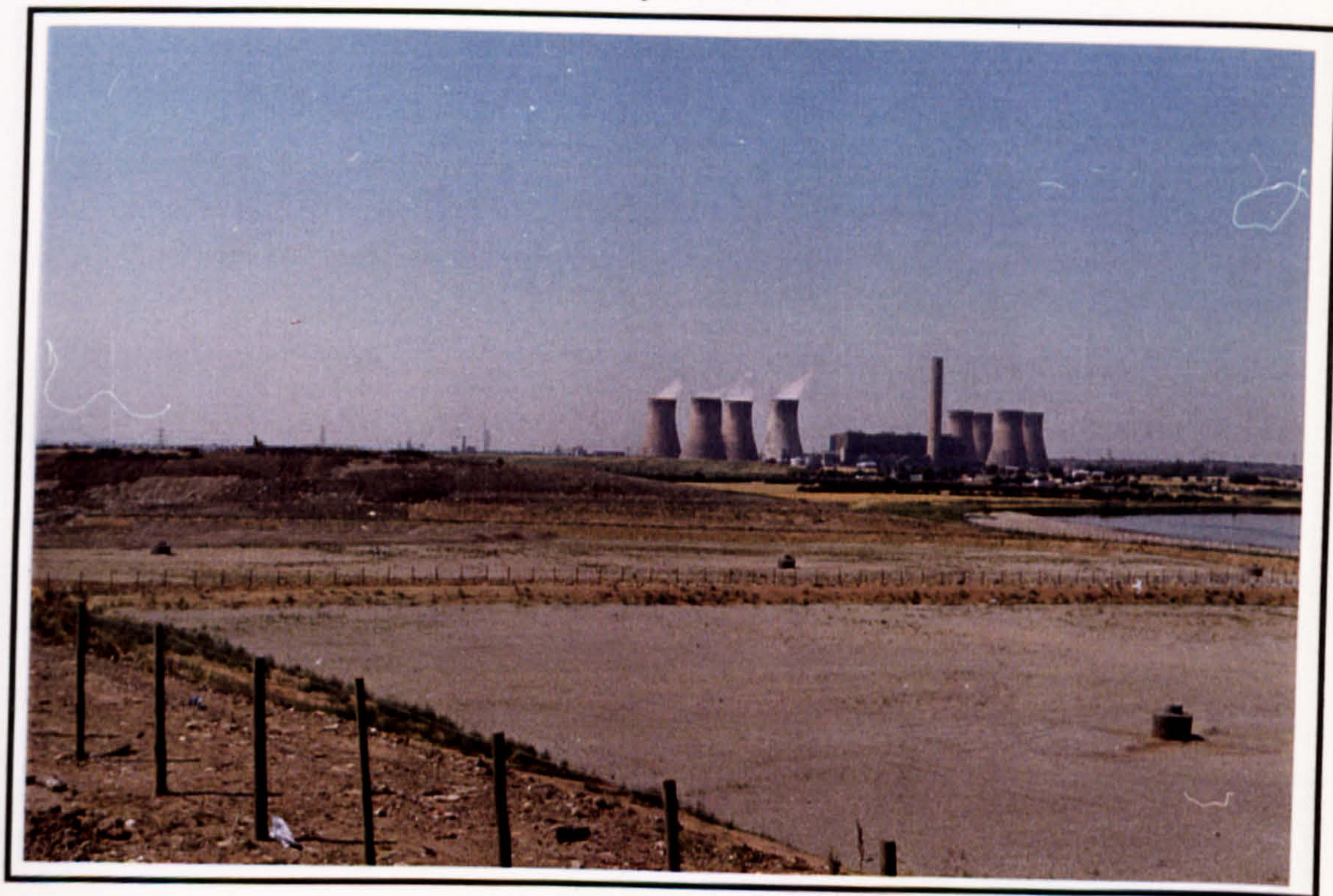
Plate 1-10: Ready cells with security fences
