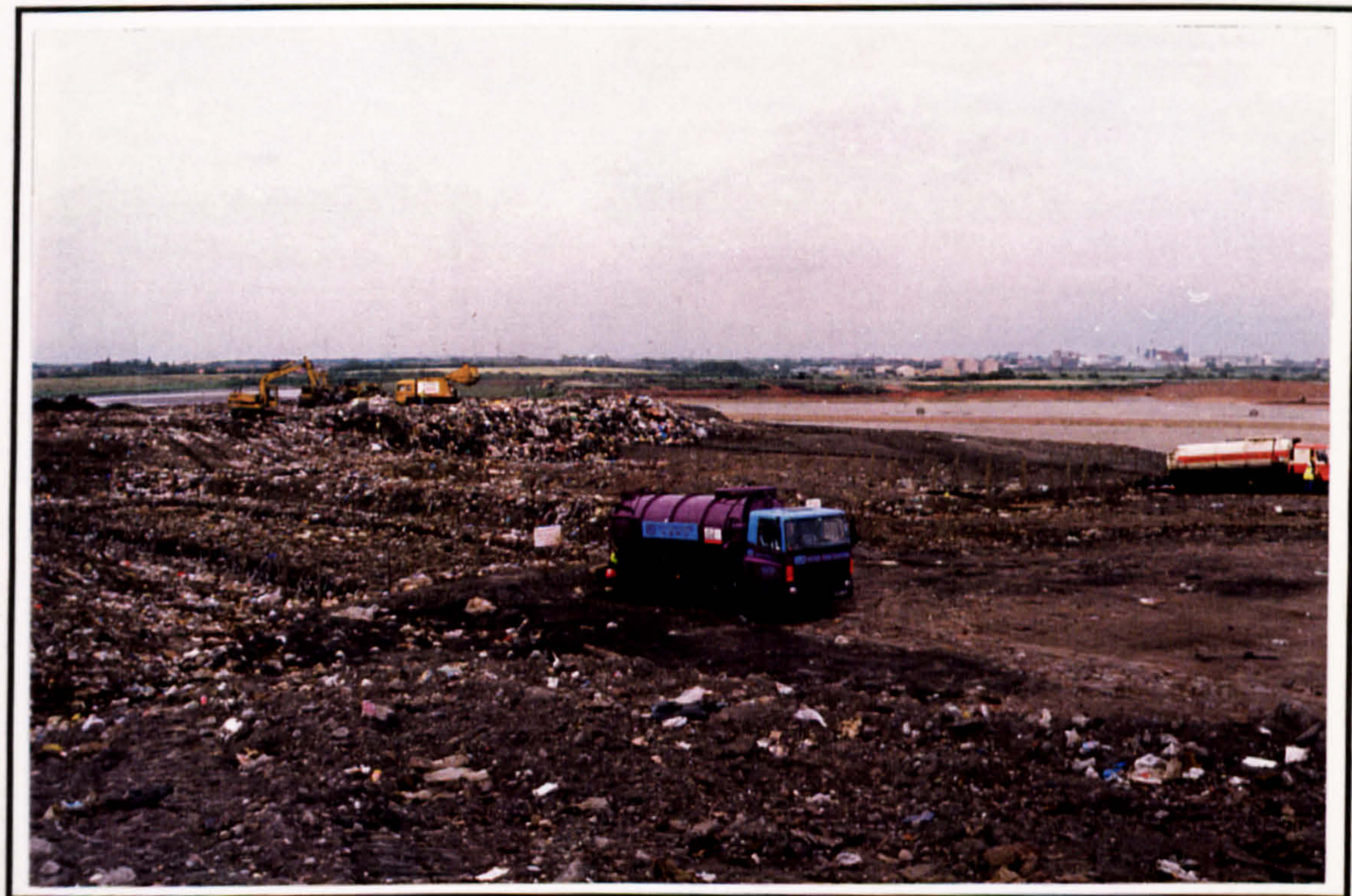
Plate 1-12: Tankers taking position to unload and discharge sludge and liquid wastes in the co-disposal pits
