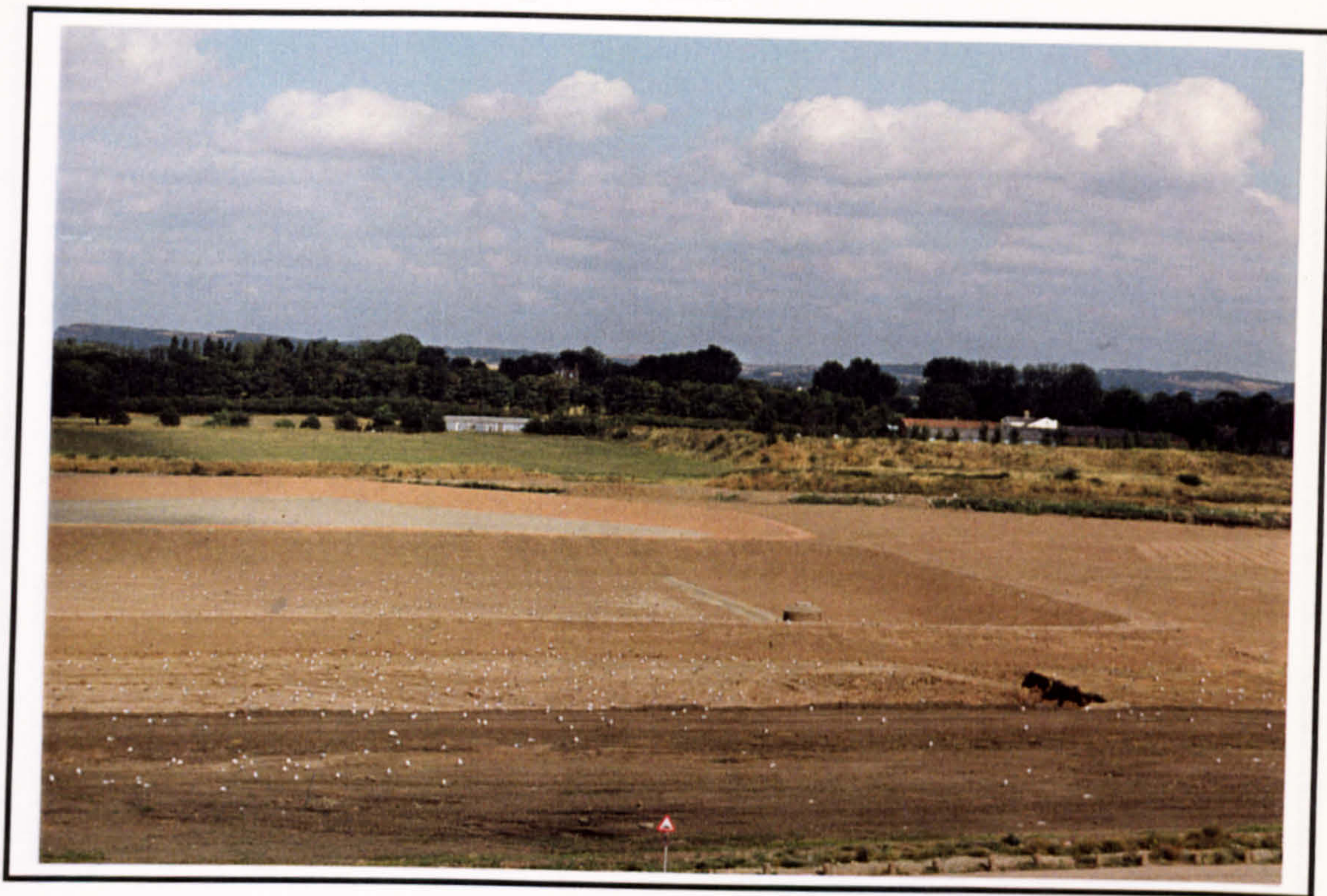
Plate 1-9: Two completed cells with bund
