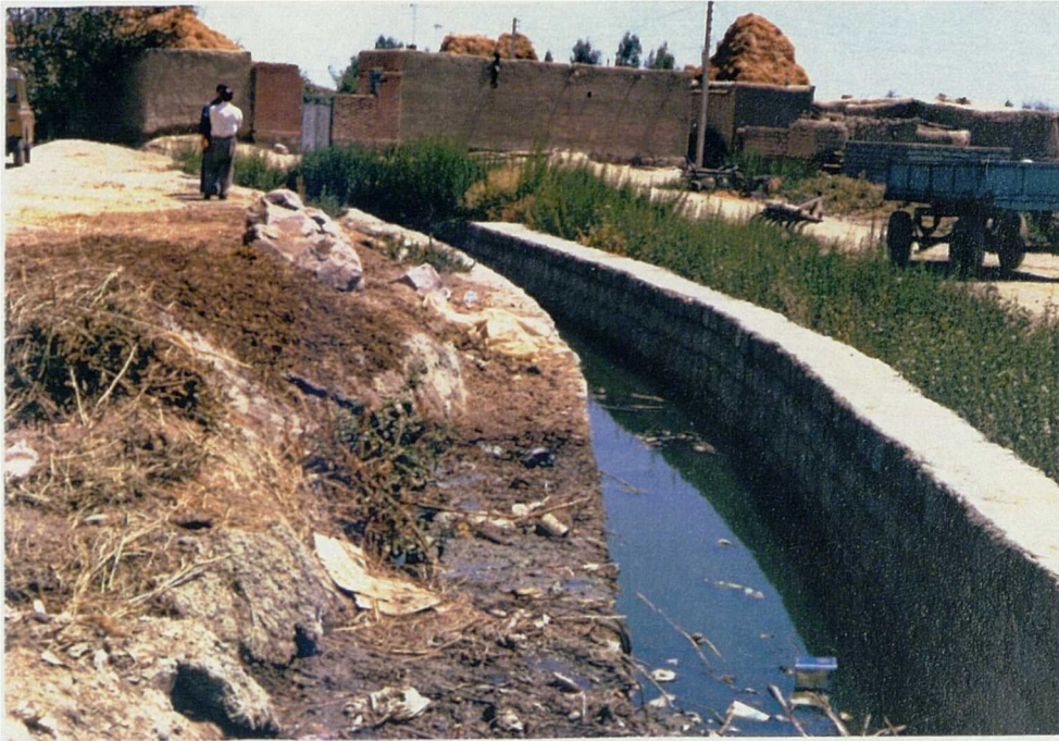
Photo 7.7 Flowing of waste water to open canal (village A)
