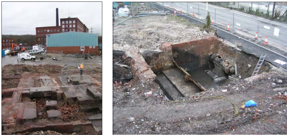
Fig. 122. Portwood Mill. Left: general view of the engine house during excavation. Right: the wheelhouse with the Gilkes twin turbine in situ.
