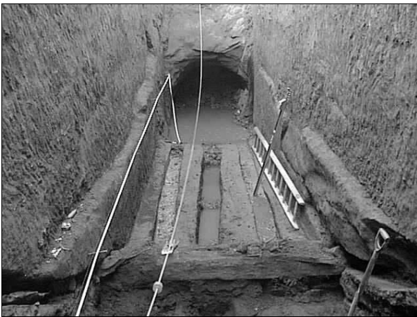
Fig. 118. Castle Mill: the wheelpit during excavation. Top: general view showing the rock-cut niches (arrowed); bottom: detail of the base timbers showing the cross-beam.
