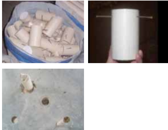
Figure 48: A Poka-Yoke System on the Pipe Head
