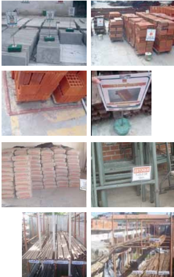
Figure 6: Locating and Identifying the Construction Materials
