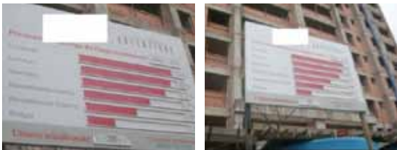
Figure 38: The Construction Progress Board
