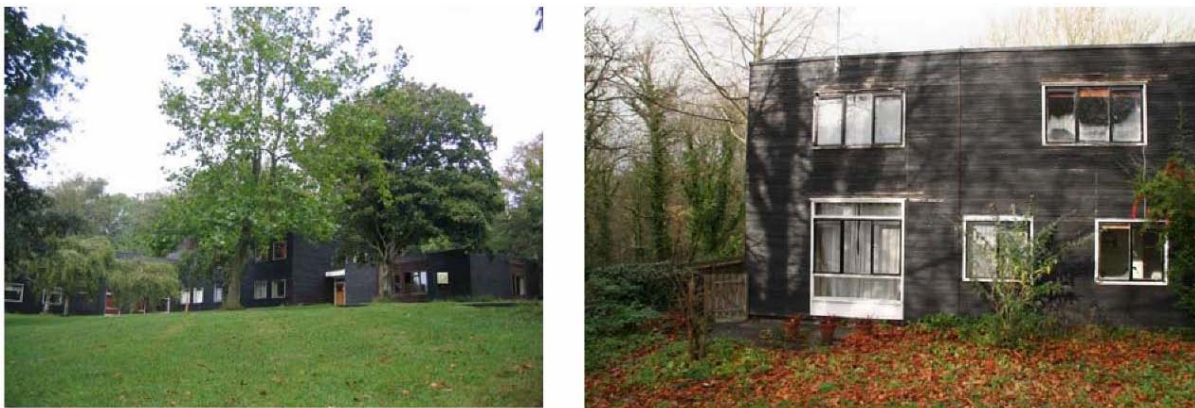
Figure 2.5 One of the three accommodation blocks at Atlantic College prior to renovation. Image from; (Gillard et al 2008).
