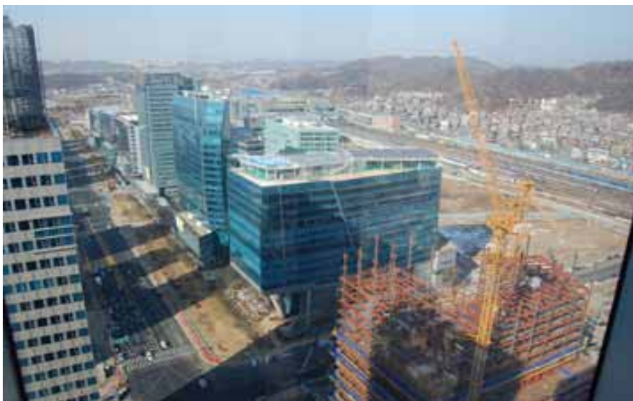
Figure 2.5 Seoul DMC under construction (NCC Workshop, 2009)
