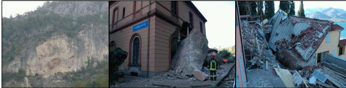
Figure 1: A case of rockfall happened at Fiumelatte di Varenna (Northern Italy); on the left is shown the rock face where in november 2004 several big masses fell and hit a railway station and a house
