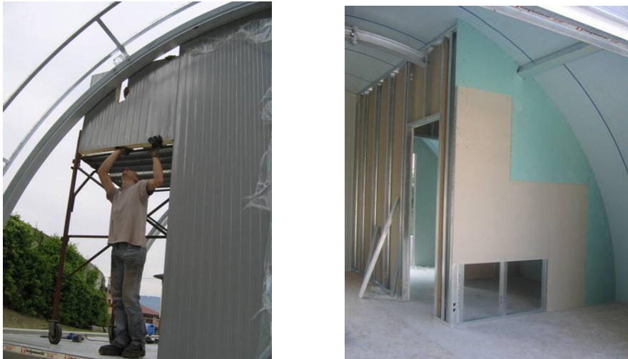
Figure14,15 Construction assembly of external sandwich façade and internal gypsum board walls
