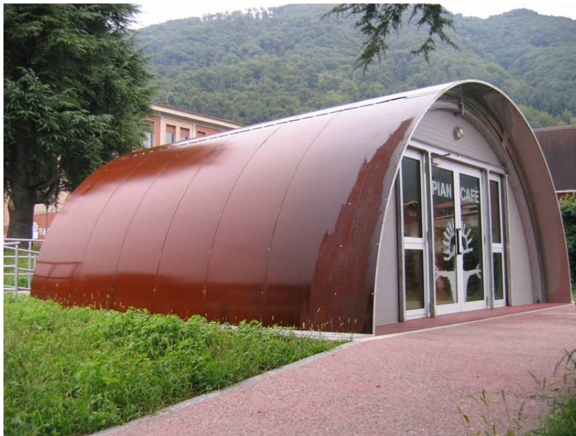
Figure16 South Façade and corten steel high durability outer shell
