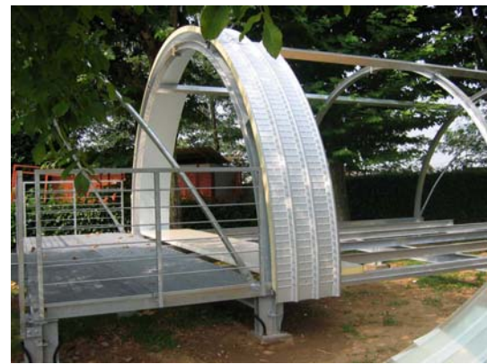
Figures 5,6,7,8 The 3 hinged main arches are in ordinary steel profiles HEA 120 mm and they carry the secondary rectangular beam section profiles on which is fixed the curved Elycop panel. On the floor a sandwich panel of 80 mm which acts as bearing structure fixed on main steel beams. The final shape allows energy equipment to be integrated.
