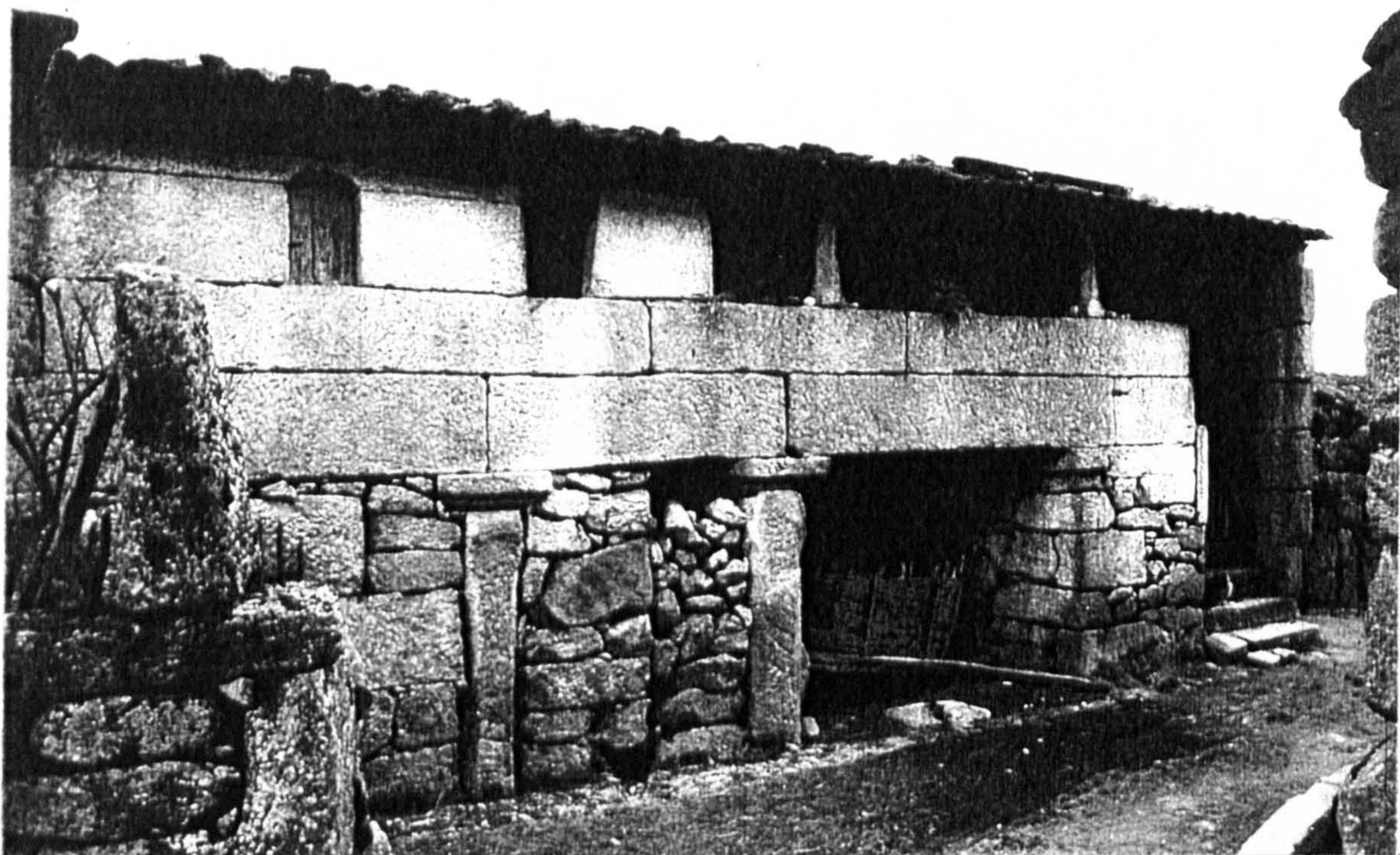
(1) - Illustrations and drawings collected from "Arquitetura Popular em Portugal" and from its remains
