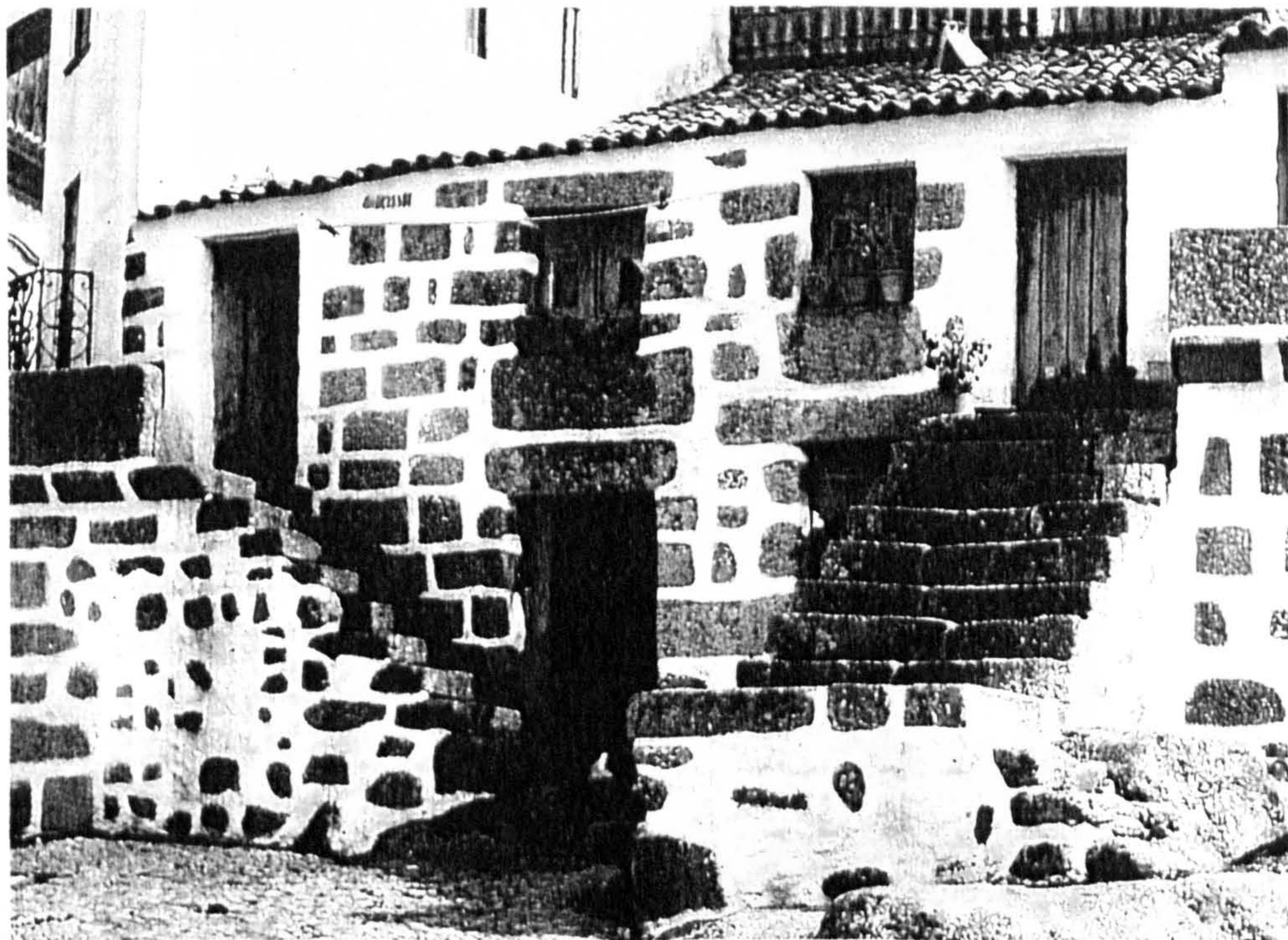
(1) - Illustrations and drawings collected from "Arquitetura Popular em Portugal" and from its remains
