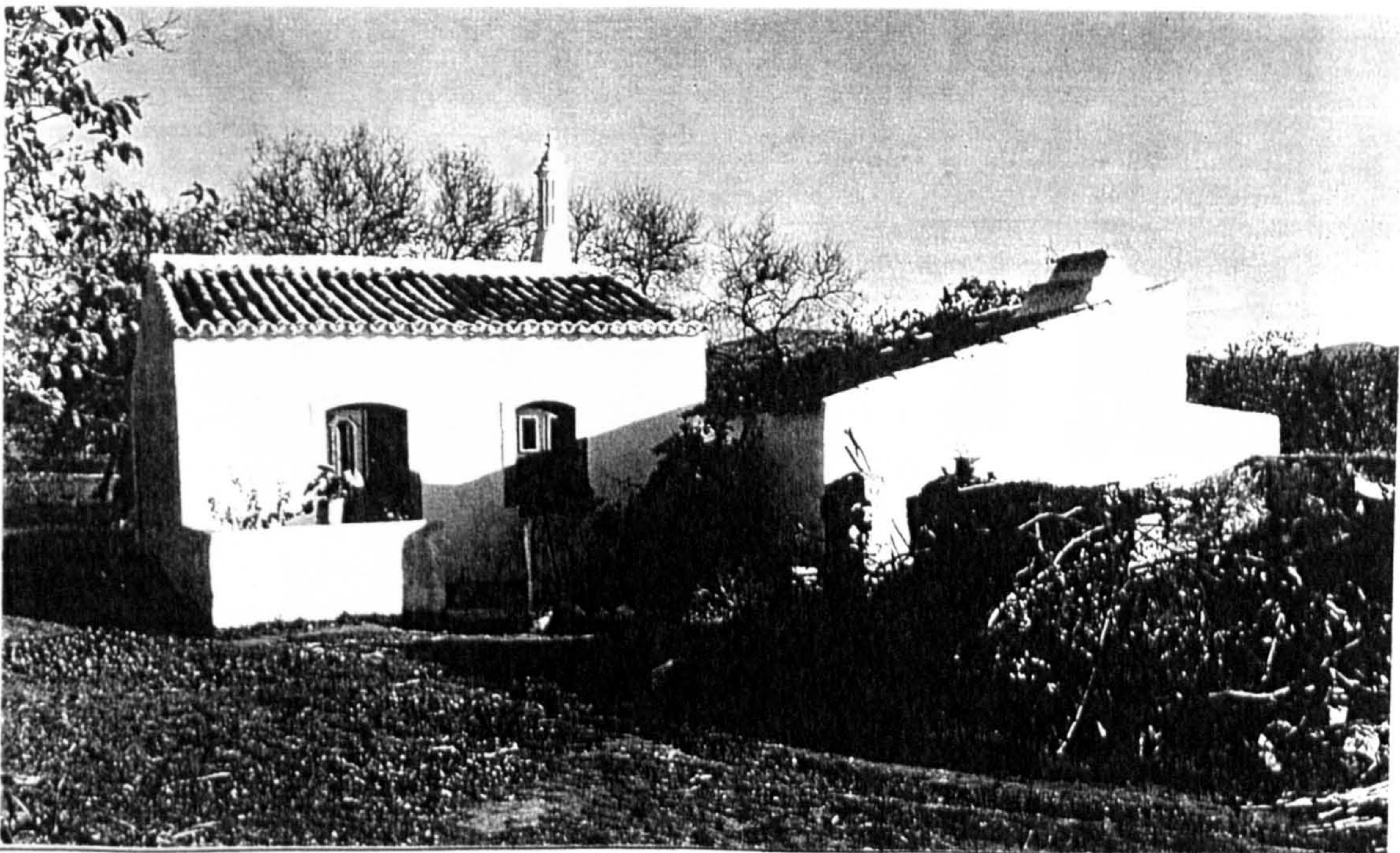
(1) - Illustrations and drawings collected from "ArquitECTURA Popular em Portugal" and from its remains
