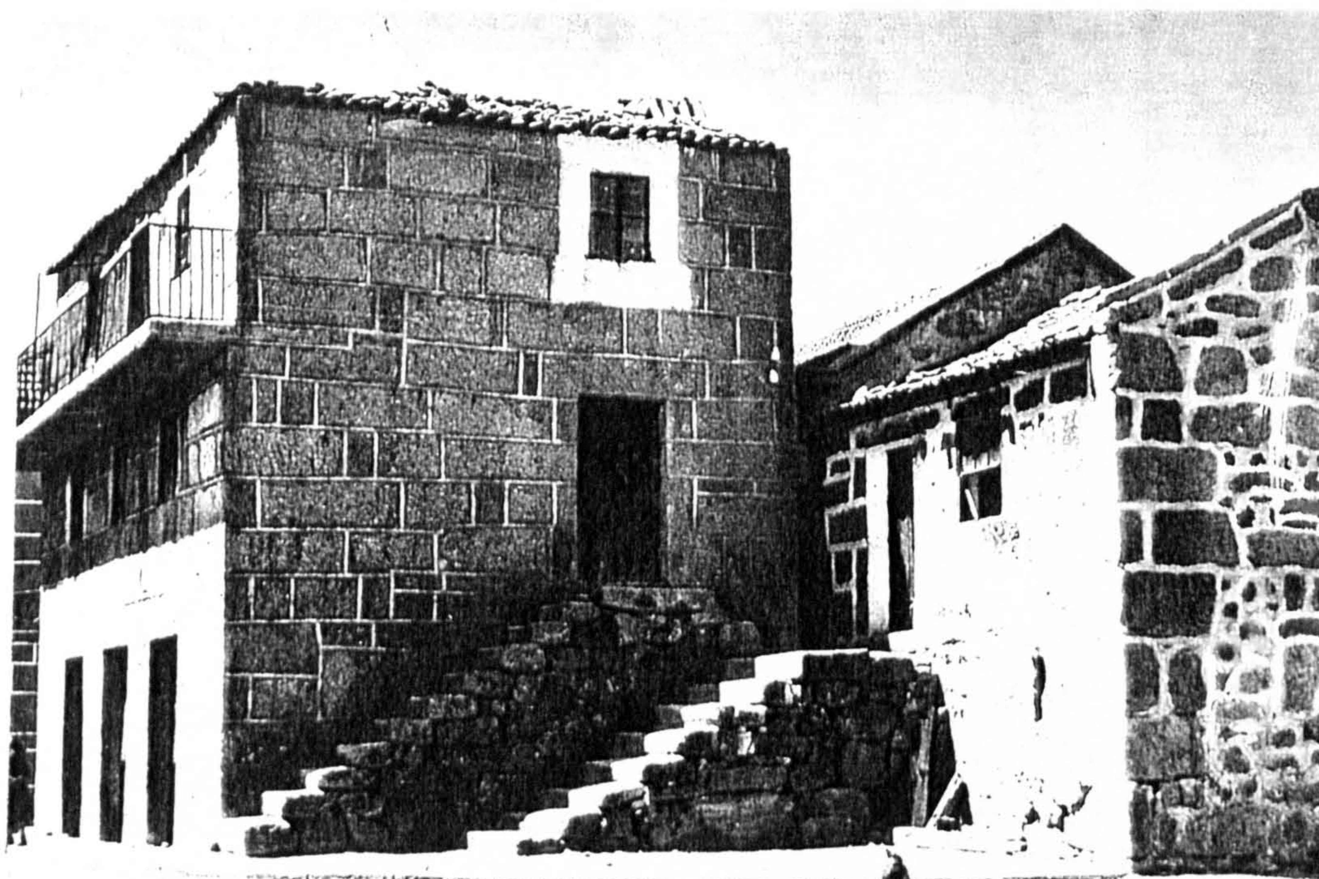
(1) - Illustrations and drawings collected from "Arquitetura Popular em Portugal" and from its remains
