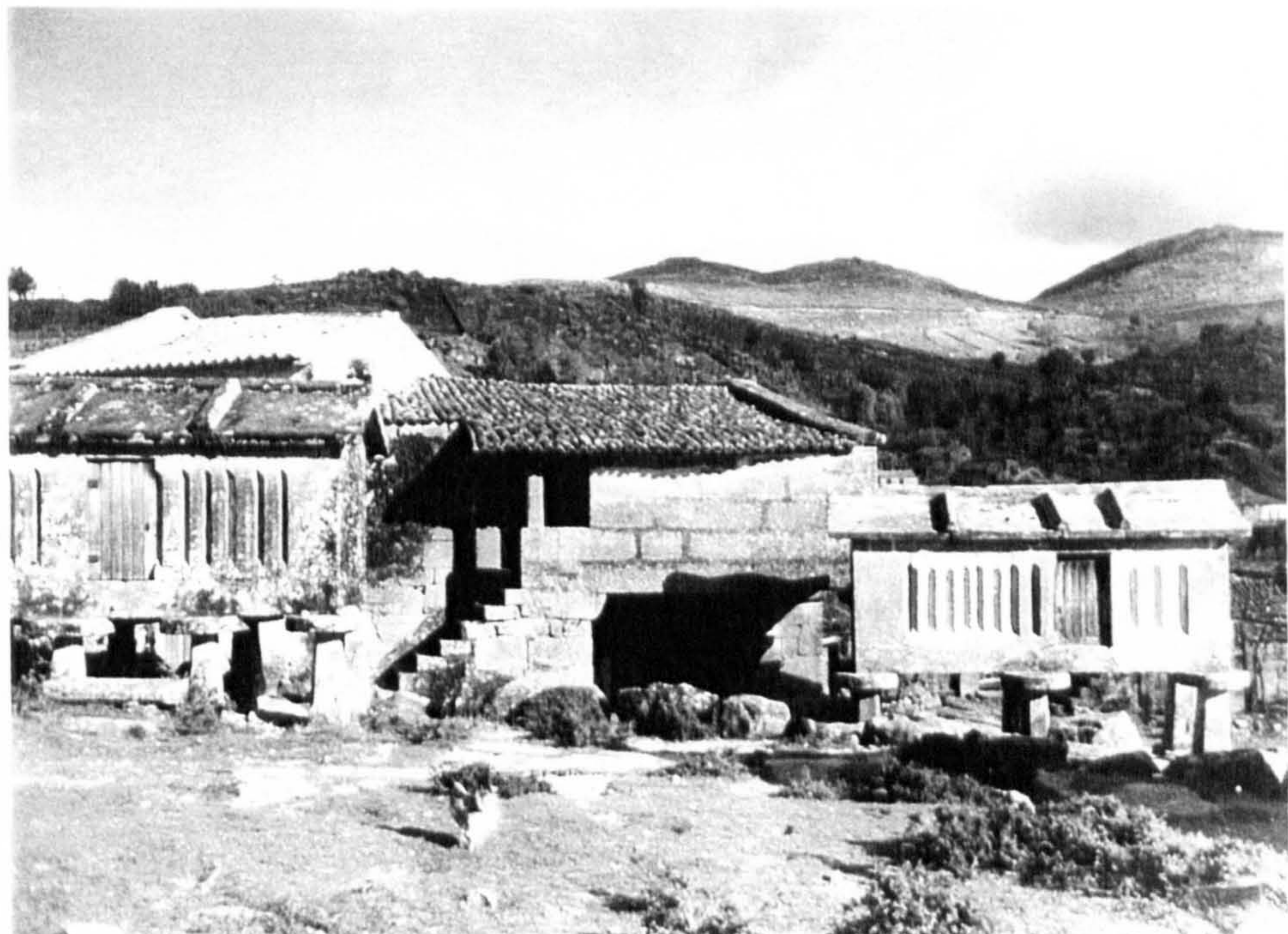
(1) - Illustrations and drawings collected from "Arquitectura Popular em Portugal" and from its remains
