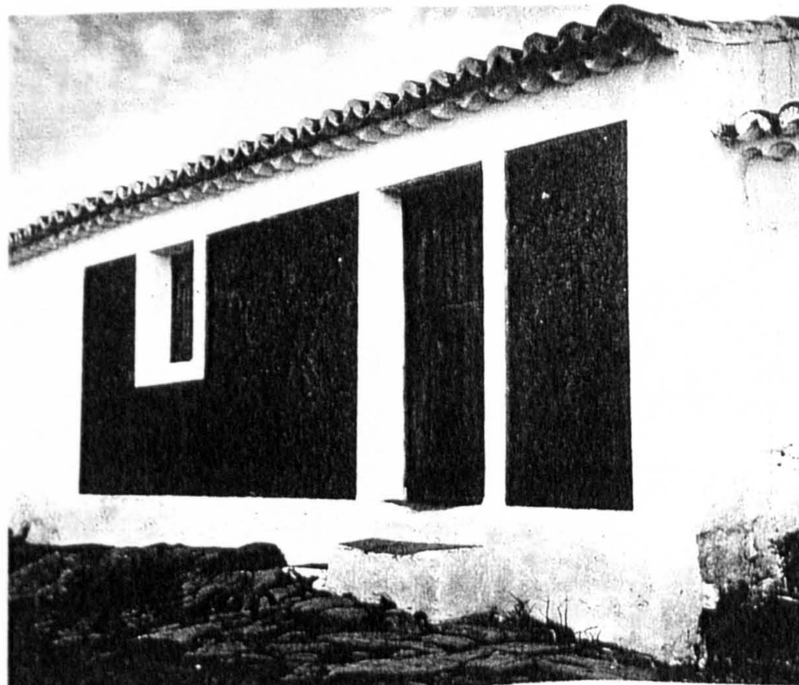
(1) - Illustrations and drawings collected from "Arquitectura Popular em Portugal" and from its remains
