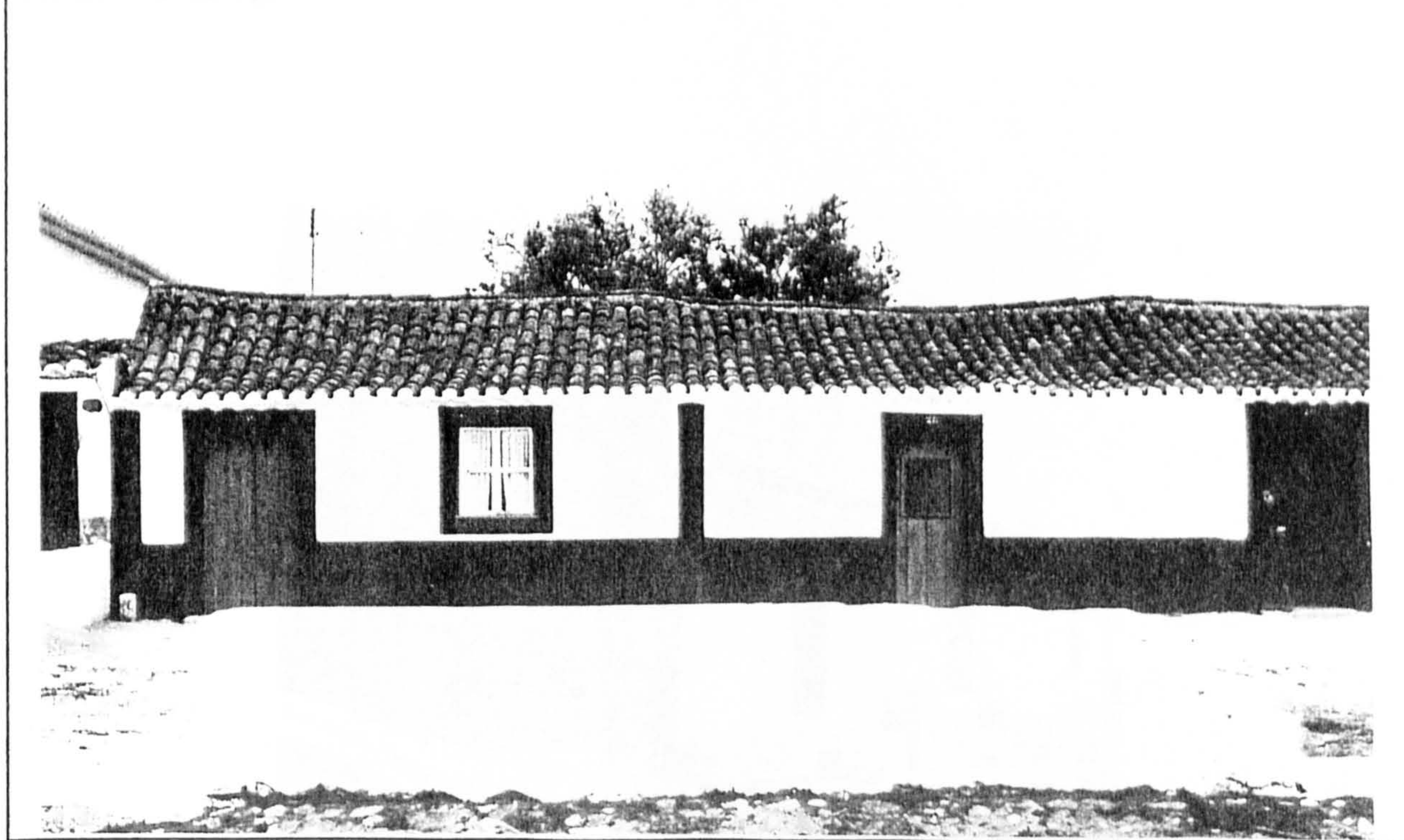
(1) - Illustrations and drawings collected from "Arquitectura Popular em Portugal" and from its remains
