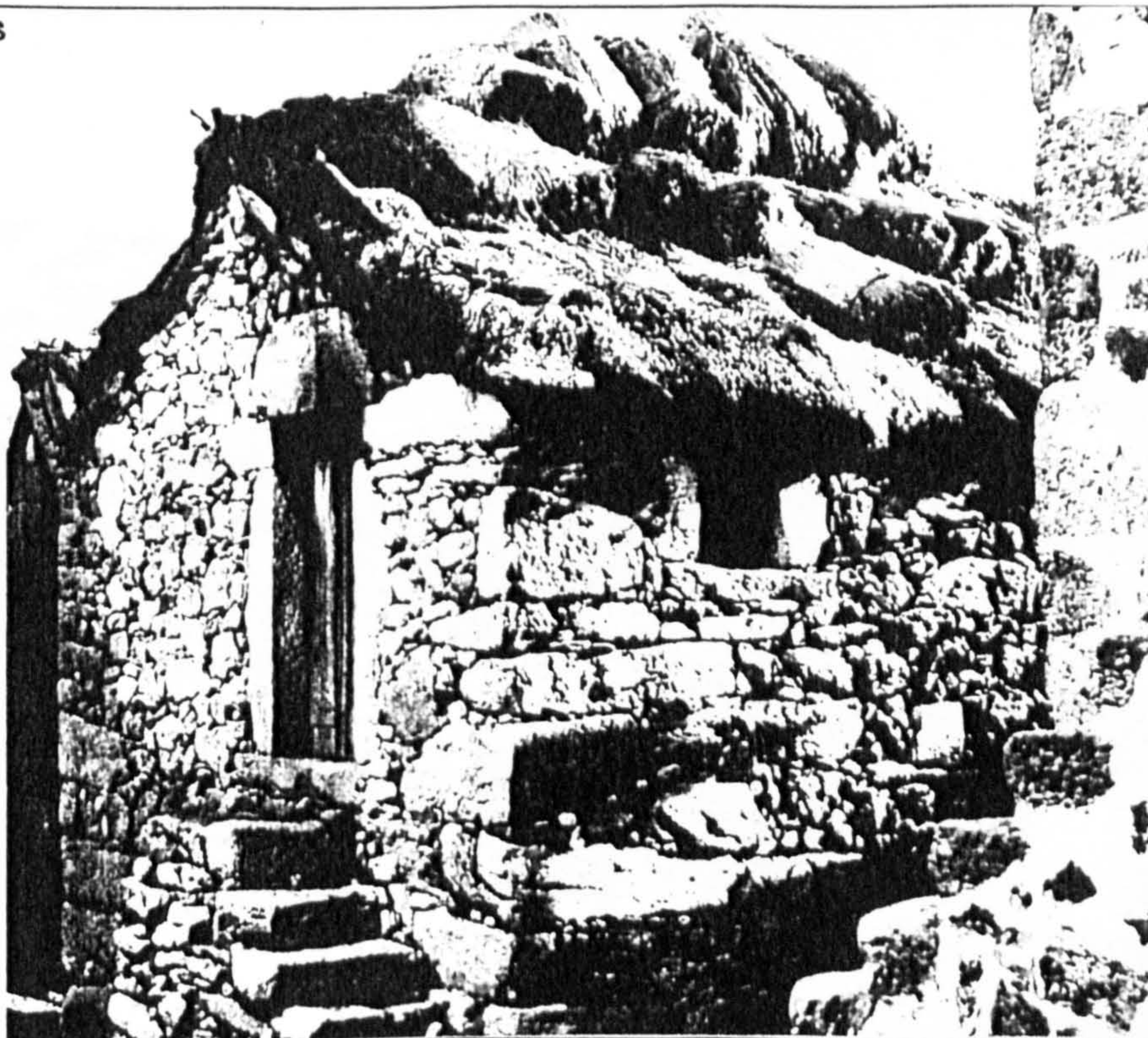
(1) - Illustrations and drawings collected from "Arquitetura Popular em Portugal" and from its remains
