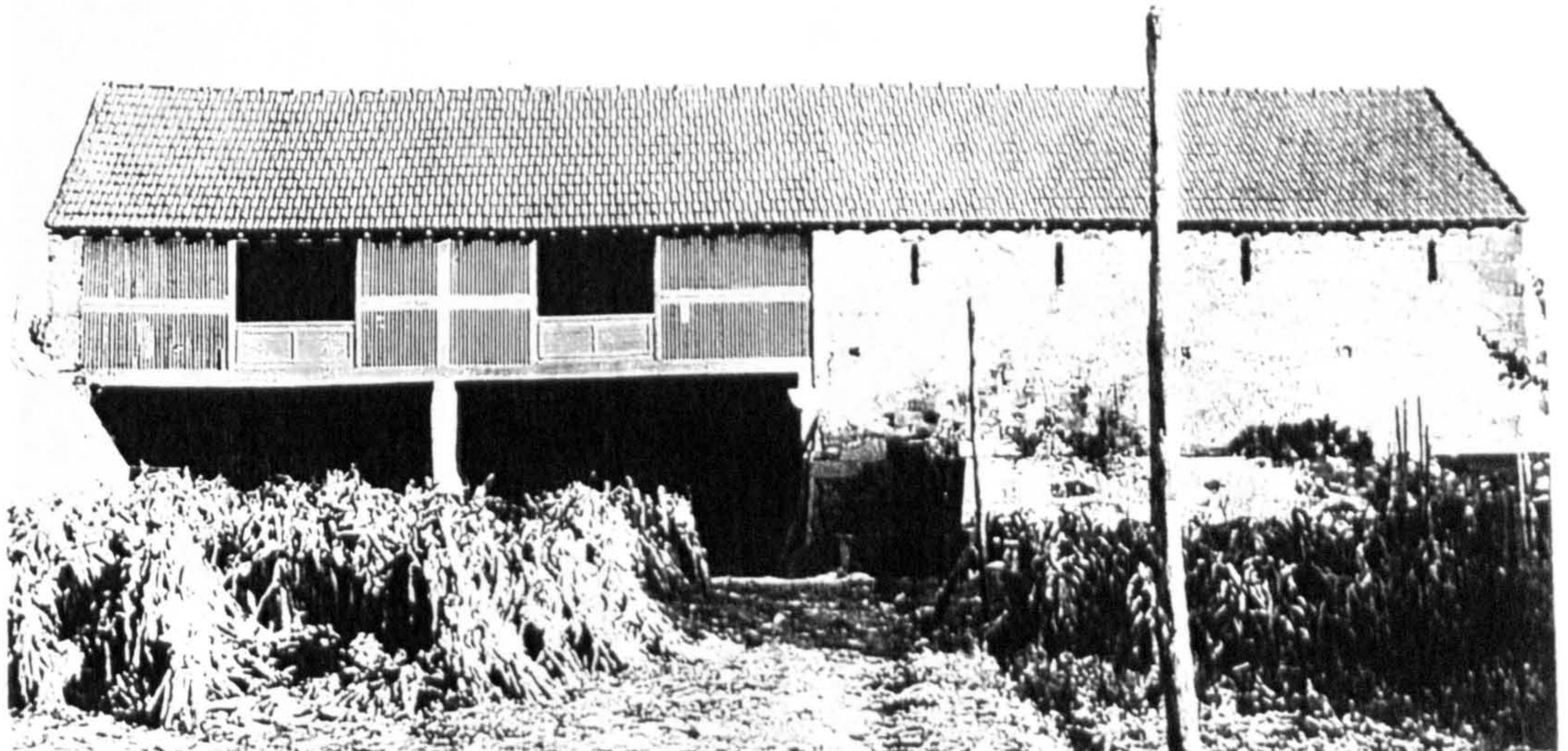
(1) - Illustrations and drawings collected from "Arquitetura Popular em Portugal" and from its remains
