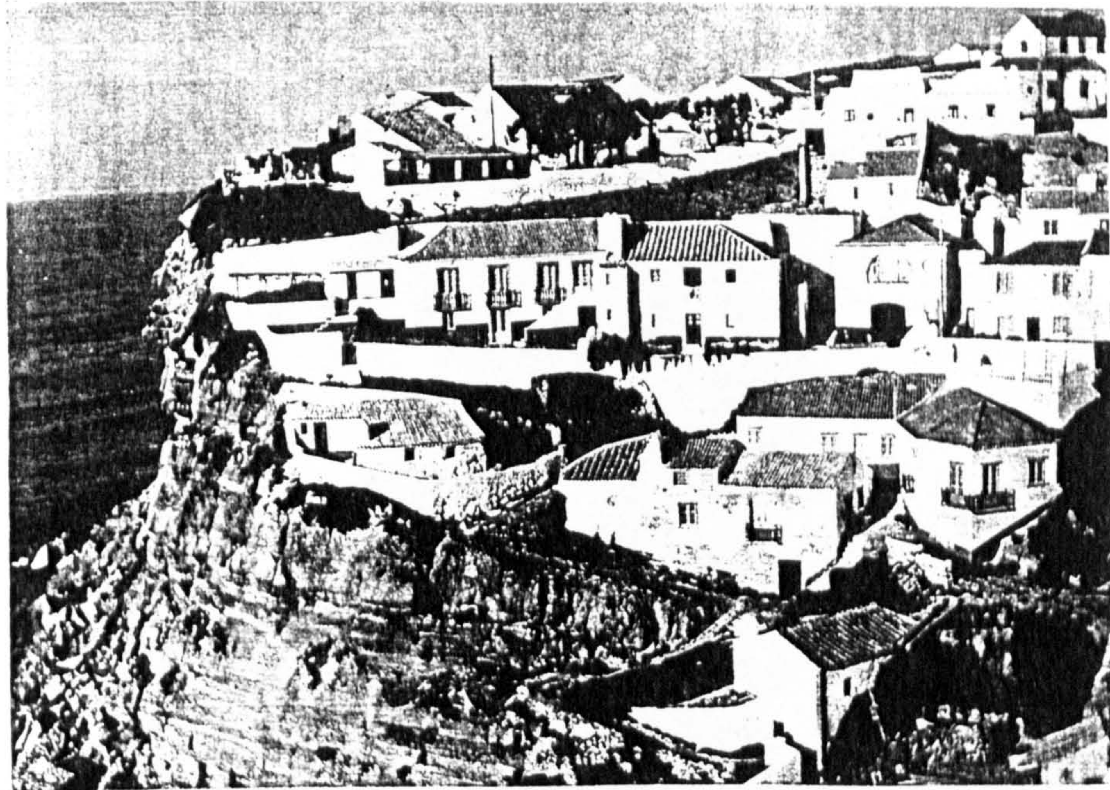
(1) - Illustrations and drawings collected from "Arquitetura Popular em Portugal" and from its remains
