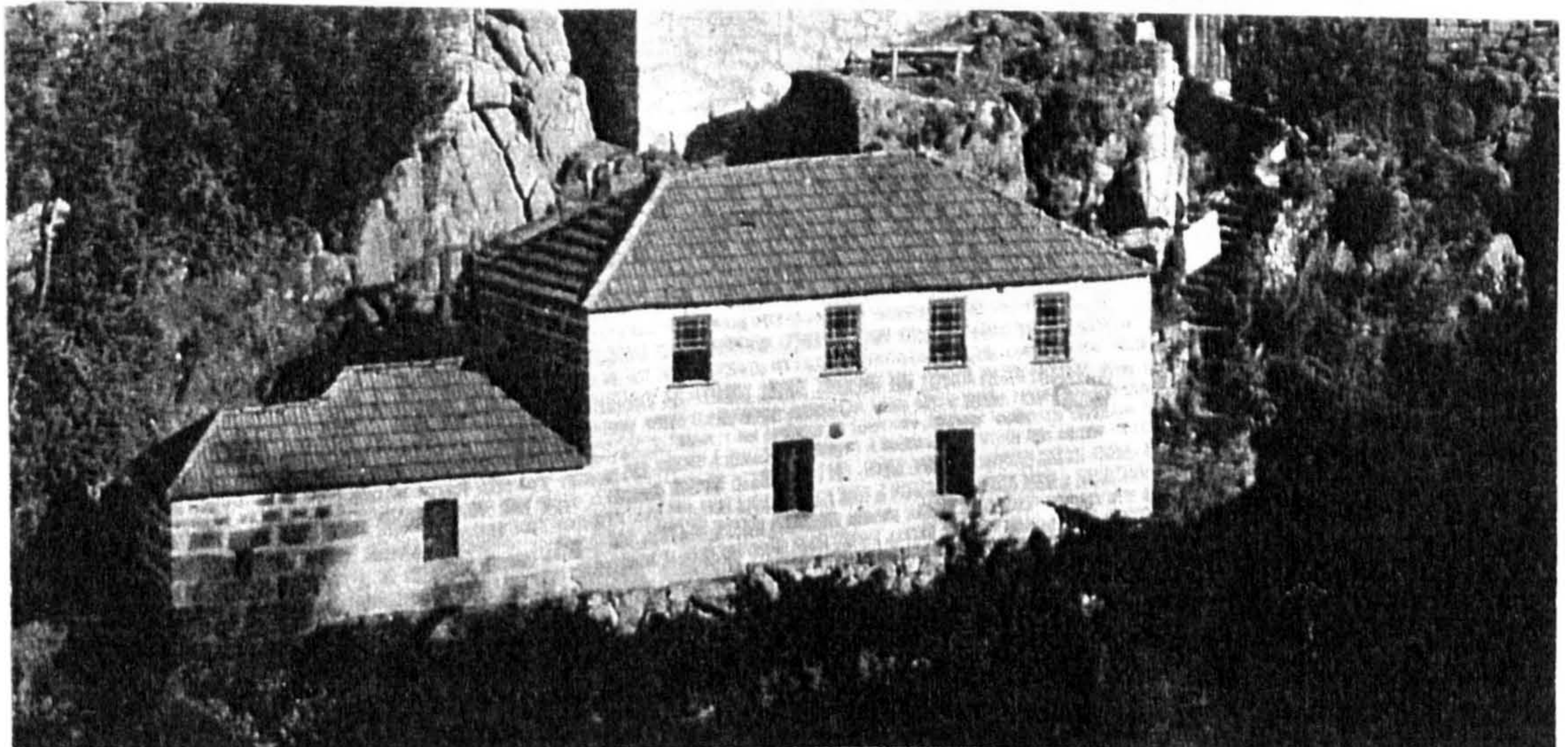
(1) - Illustrations and drawings collected from "Arquitetura Popular em Portugal" and from its remains
