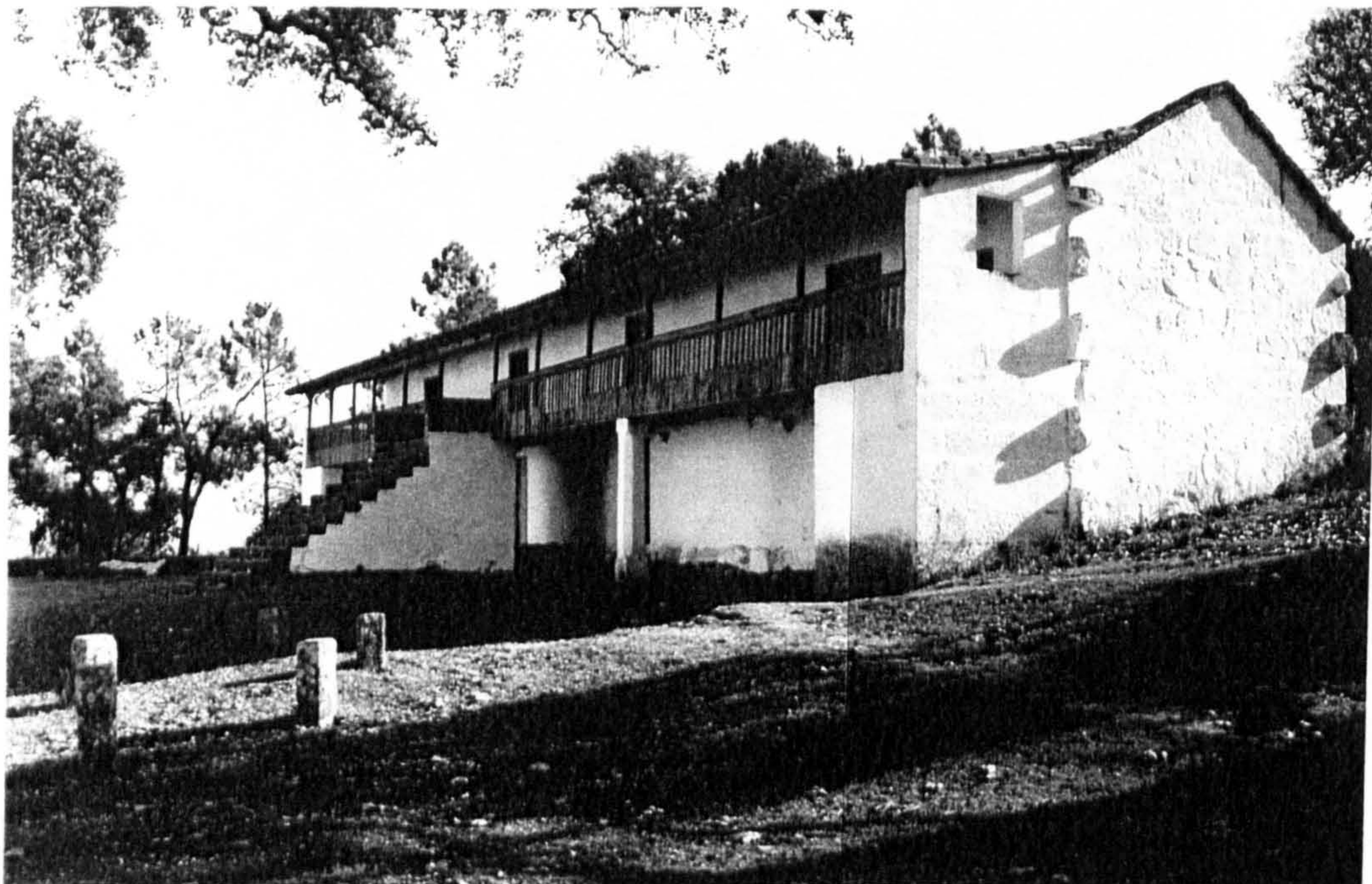
(1) - Illustrations and drawings collected from "Arquitectura Popular em Portugal" and from its remains
