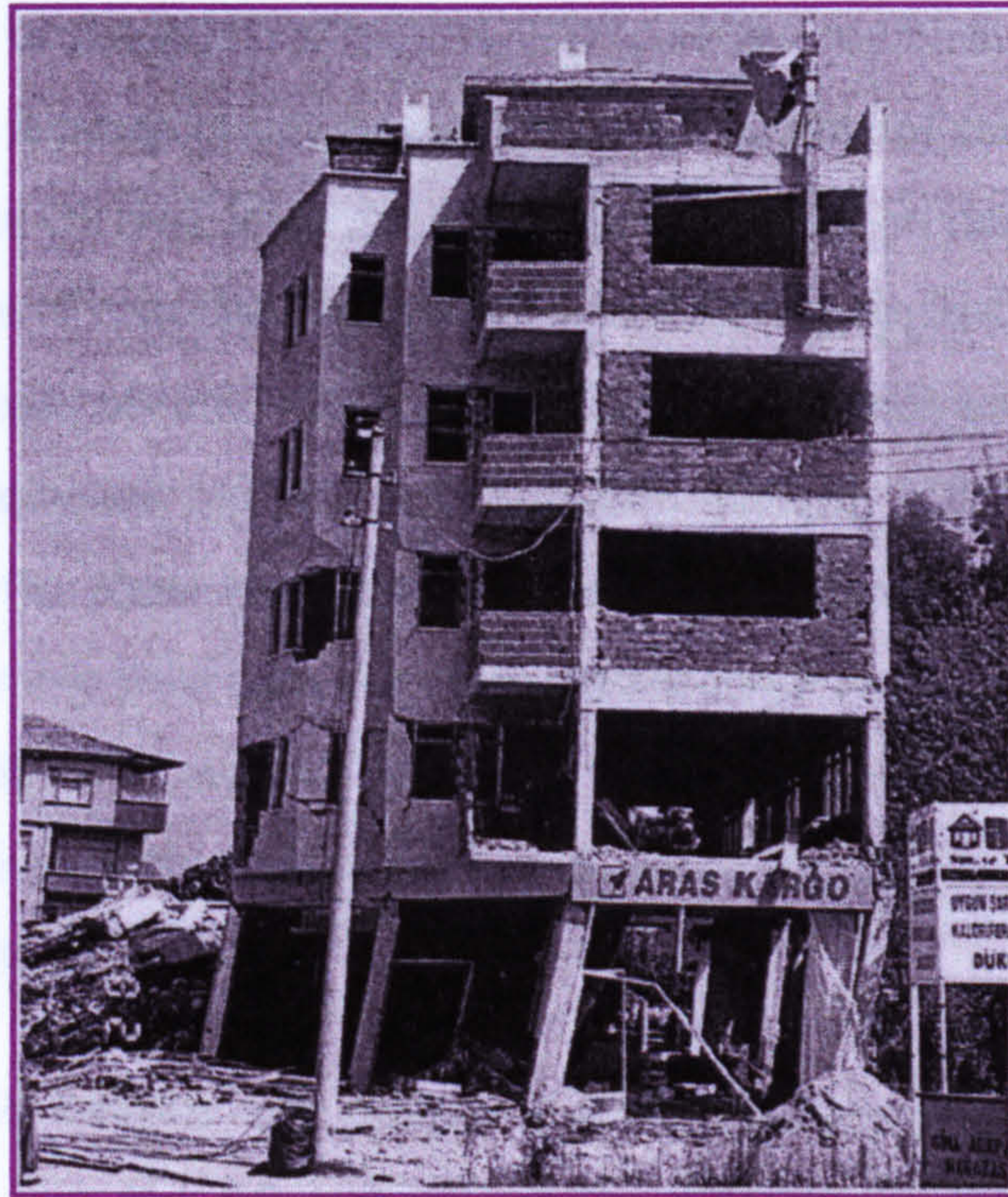
Figure 2.12 Formation of a soft and weak storey, 1999 Turkey earthquake (Sezen...et al, ref [21])
