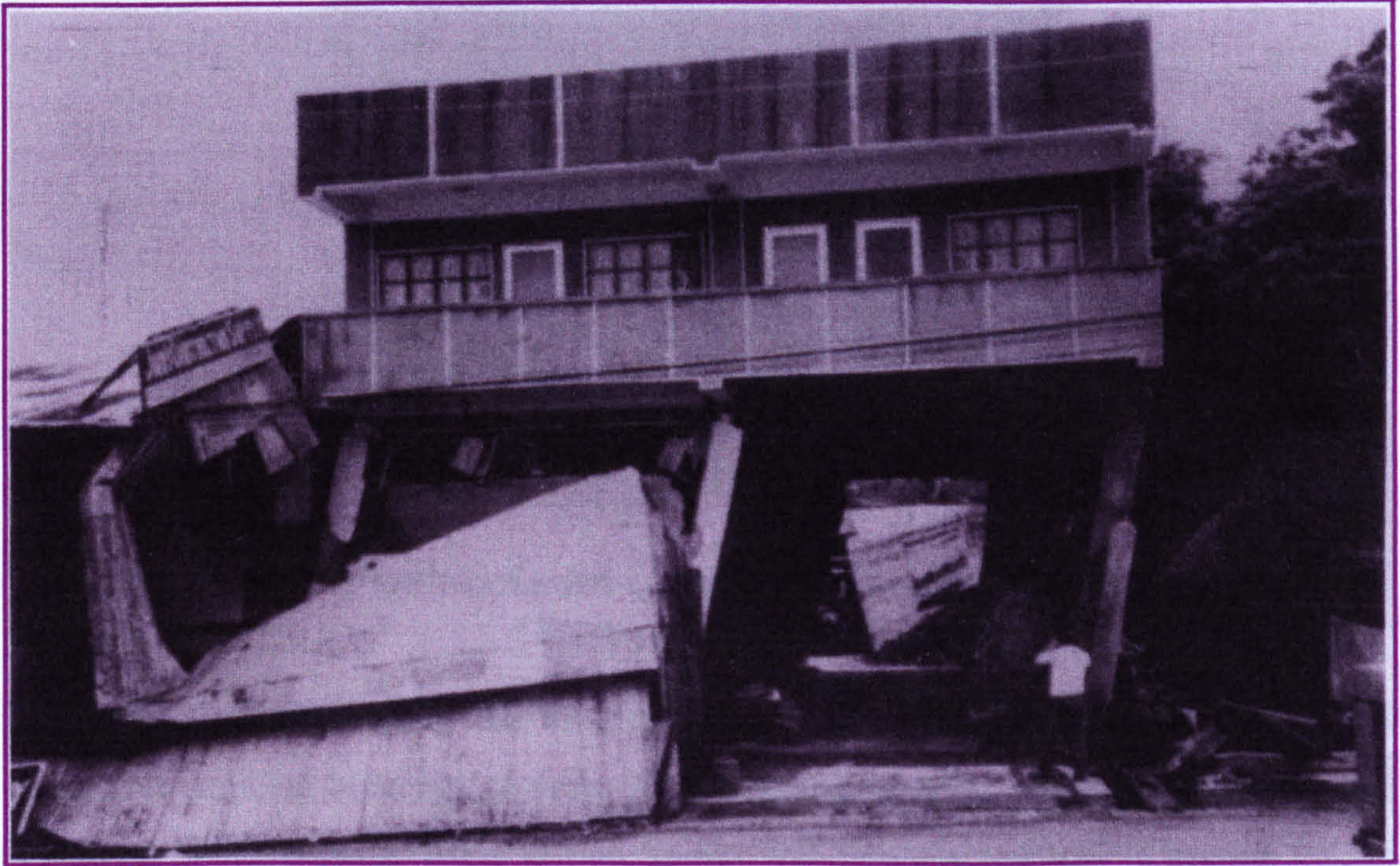
Figure 2.11 Soft –storey sway mechanism, 1990 Philippine earthquake (Paulay & Priestley, ref. [20])
