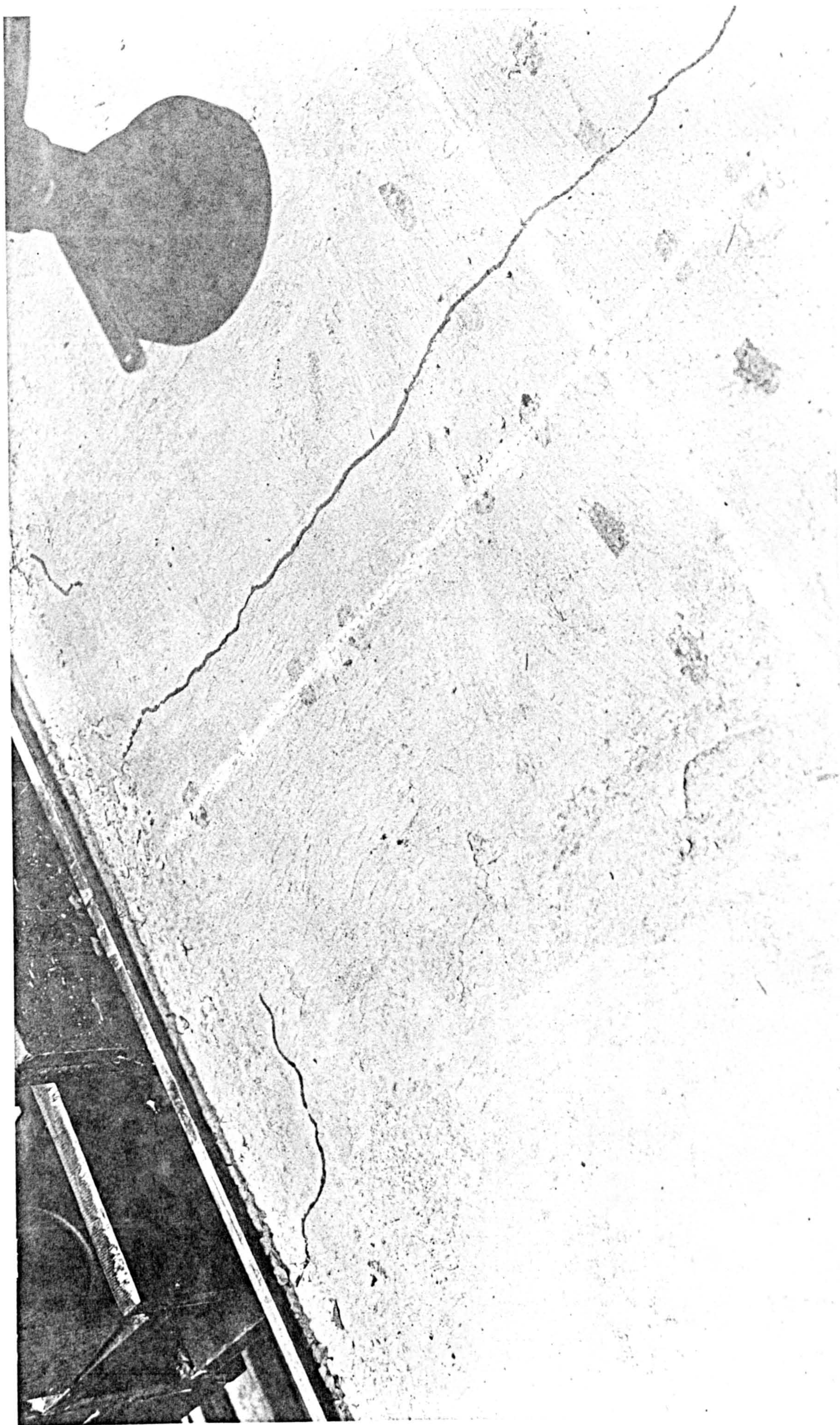
4.4b LONG. CRACK ACCOMPANYING FAILURE OF CSFU2 (TYPICAL FOR ALL CSFUS)
