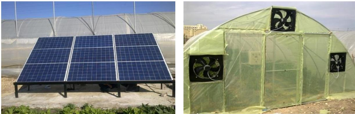
**Figure 1.** Solar energy cells used in the experiment (left), front side of the walk-in tunnel with evaporative cooling system (right).
