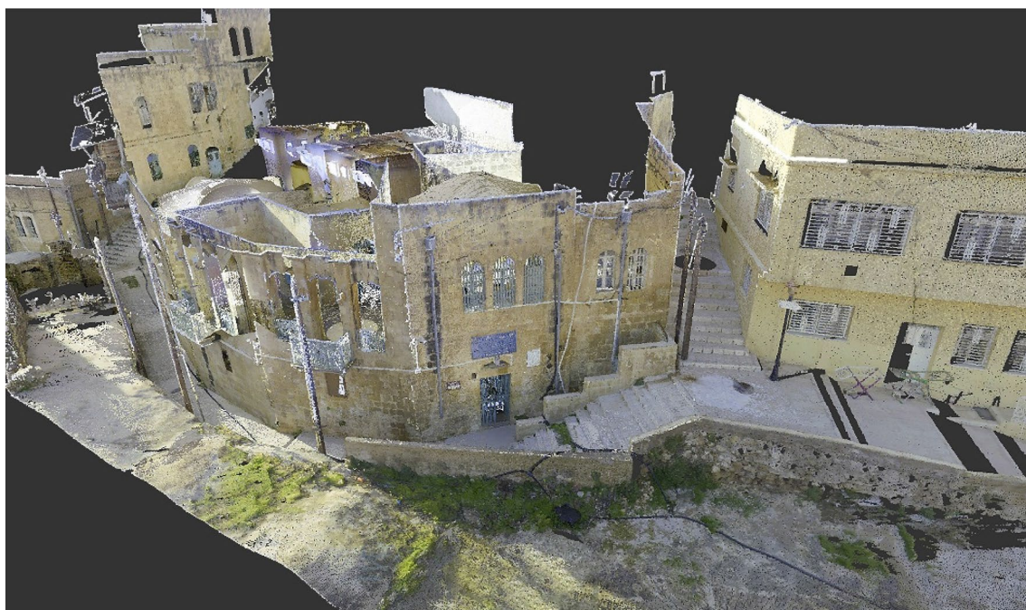
Fig. 6 Detail of the point cloud of the Qaqish House
