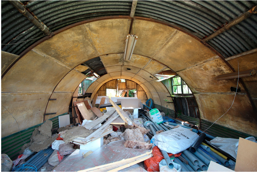
Figure 7. General view inside the kitchen Nissen Hut, showing curved asbestos sheeting (© University of Salford).
