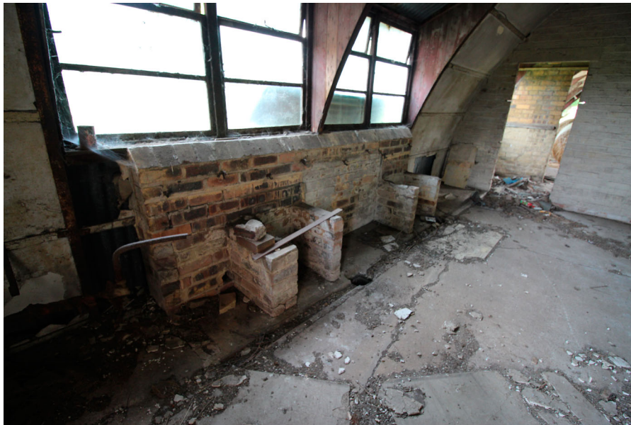
Figure 9. Detail of the remains of the sinks against the northern wall and the open drain set into the concrete floor (© University of Salford).
