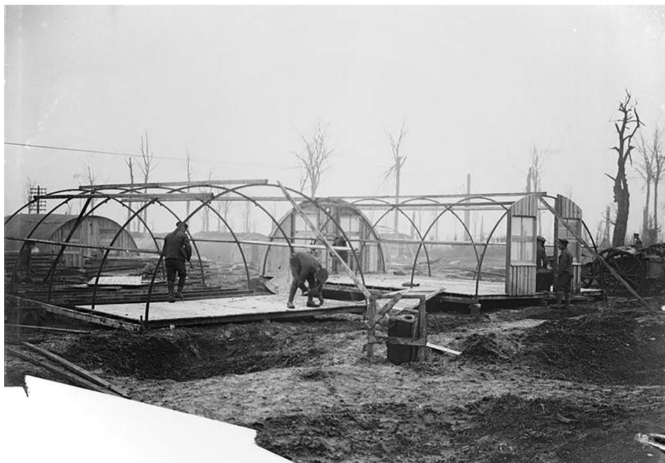
Figure 2. British troops erecting Nissen Bow Huts in France, taken by John Warwick Brooke in November 1916. This is photograph Q 4597 from the collections of the Imperial War Museums (John Warwick Brooke, public domain, via Wikimedia Commons).
