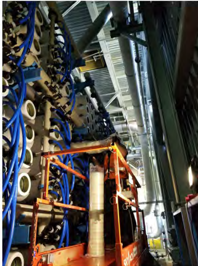
Figure 6: Loading new element without touching membrane itself
