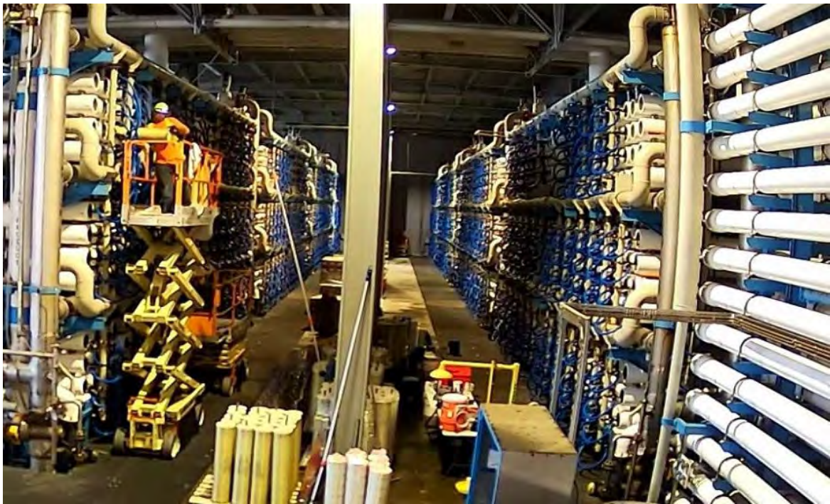
Figure 4-16. Membrane replacement
