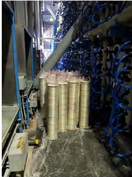
Figure 3: New element prepared in advance in vertical position in their original plastic bags
