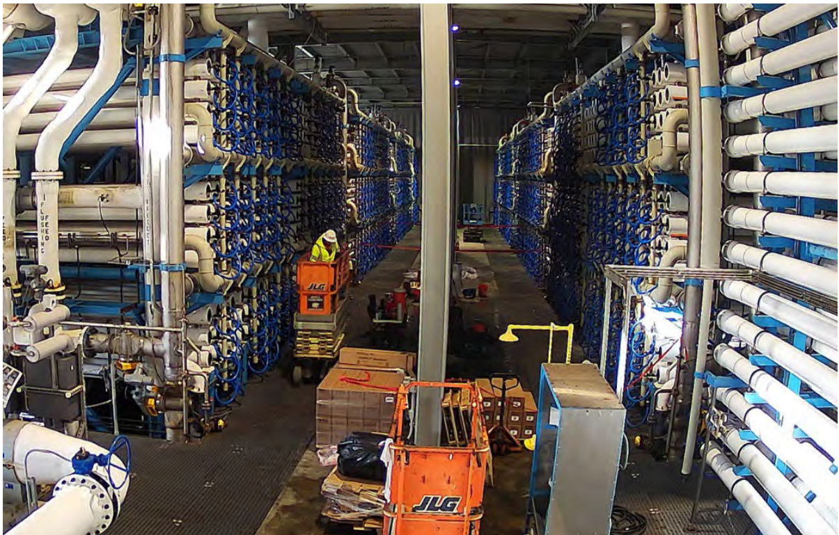
Figure 4-5. A view of the 14 RO trains of the case study
