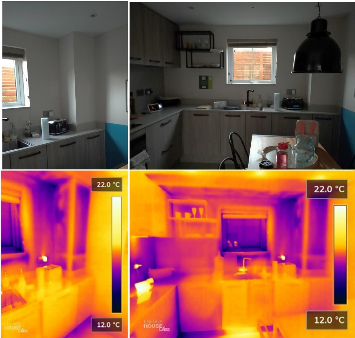
Figure 4.10 Air movement possibly from the cold roof space into the SVP void in the kitchen on the ground floor. Air movement between the SVP void into the surrounding external wall and intermediate floor void was also evident.
