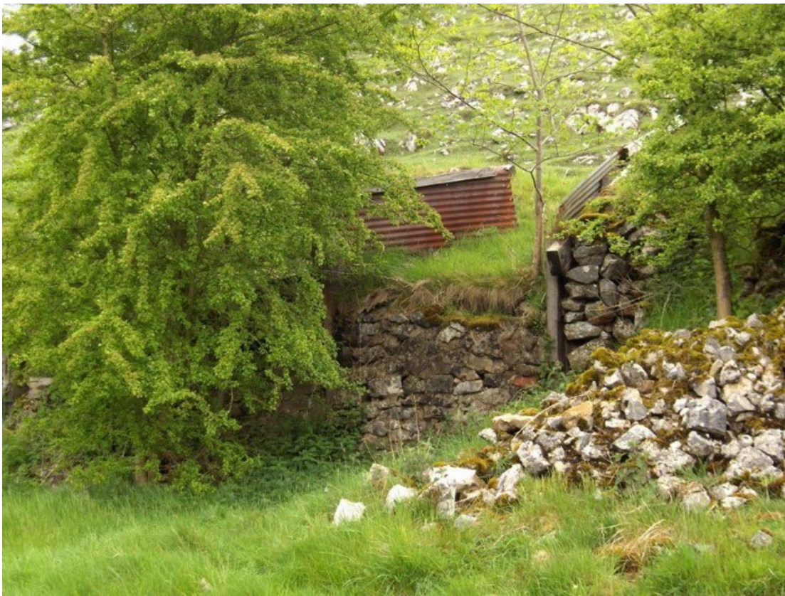
Figure.6:7. Ore chute dropping onto dale floor at Hay Dale. Source (AditNow Mining History Society (ANMHS), 2017)
