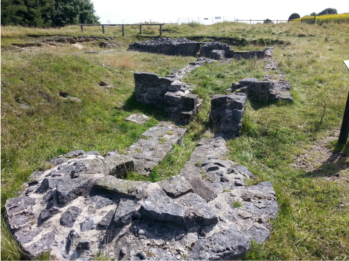
Figure 6:9. The remnants of the chimney base at High Rake. Source (Author, 2016)
