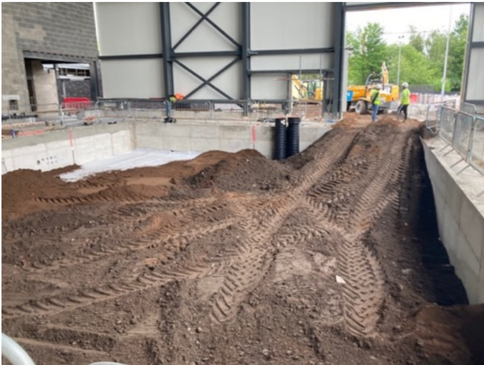
Figure 3. Construction of soil pits, present in each chamber to a depth of 120mm
