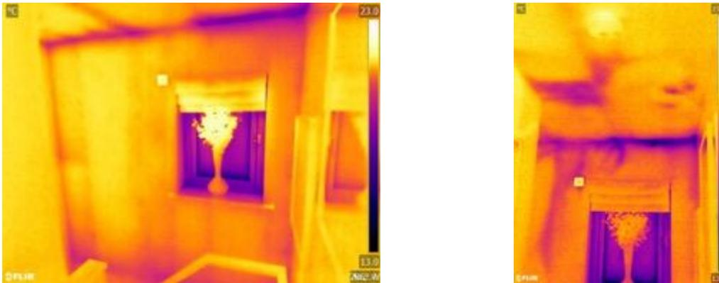
Figure 25. Stairs at atmospheric pressure (left) showing cold bridging at the rear wall/eaves junction. During depressurisation (right) air infiltration visible along the ceiling and wall behind the plasterboard, stemming from the eaves.
