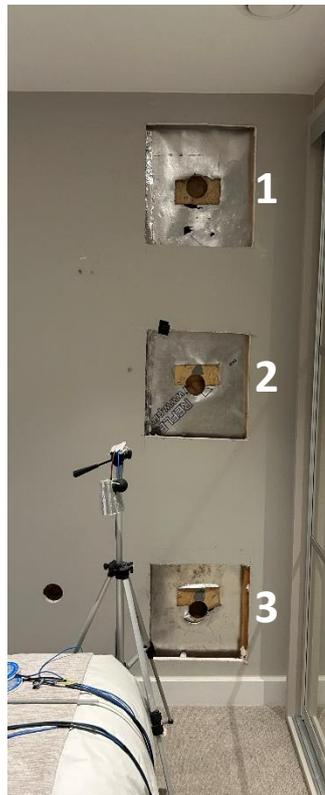
Figure 30. Recess' cut into the plasterboard and VCL layer of the external wall in Bedroom 1
