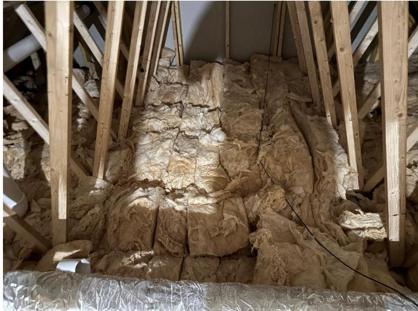
Figure 33. Photograph of the loft insulation. It can be observed that the insulation is not homogenous or evenly distributed across the area of the loft. Suboptimal application of insulation around roof trusses can be observed.
