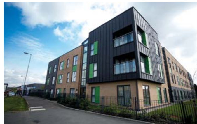
Figure 14: Tameside Court being demolished in 2017, and the replacement apartments at Honiton Avenue
