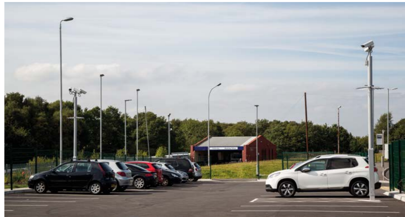
Figure 19: New car park for railway station
