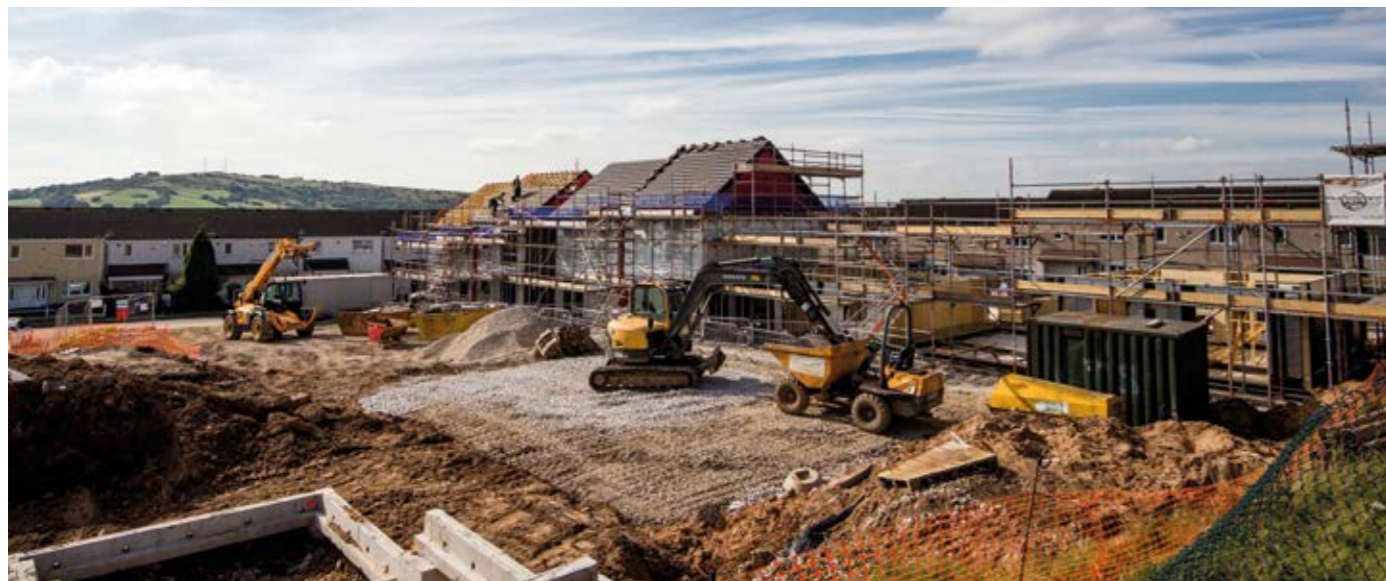
Figure 12: construction on site of new Barratt homes
