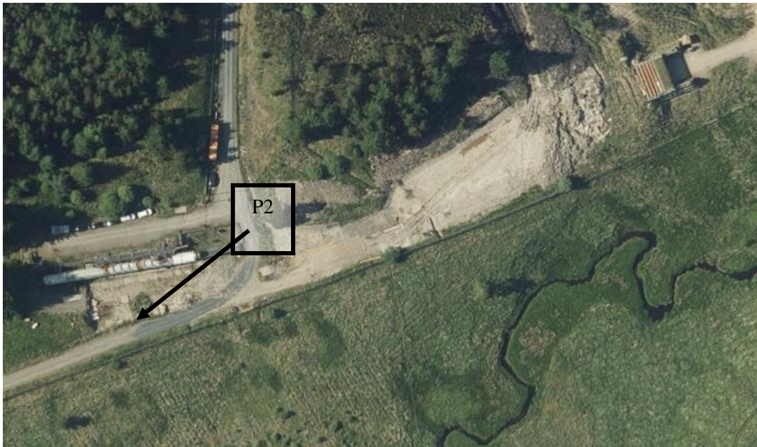
Figure 16. EDH test layout and measurement positions. P1 marks the position of a pressure gauge at the location of the test operator. P2 was a supplementary pressure gauge used during the November trials (see Table 15).
