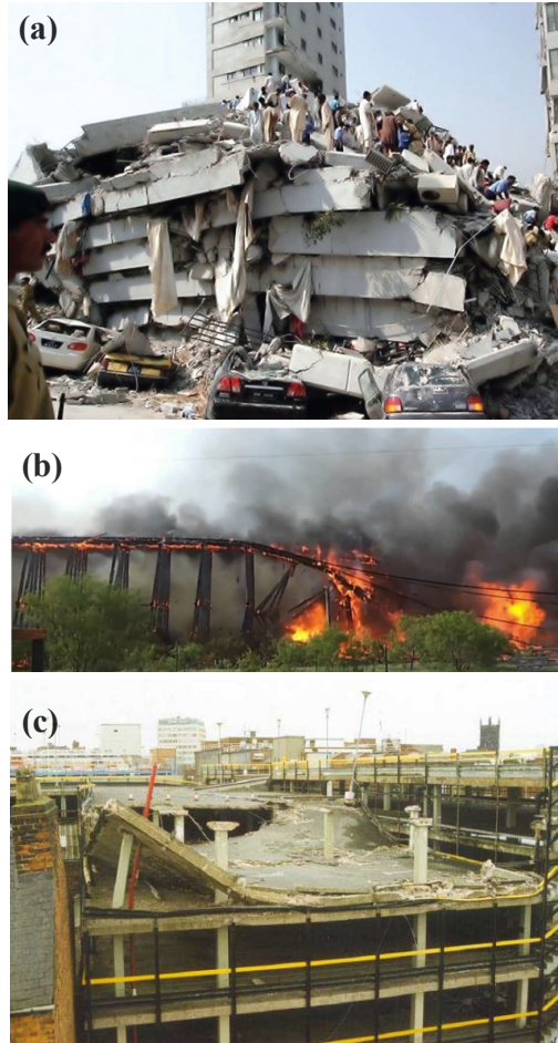
Figure 3: (a) Pancake collapse of a reinforced concrete structure following an Earthquake in Islamabad, Pakistan [42], (b) Domino collapse of a wooden trestle bridge in Texas, the USA [43], and (c) Pipers Row Car Park partial collapse, Wolverhampton, the UK [44].
