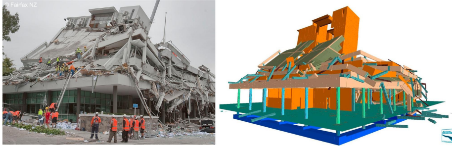
Figure 7: Pyne Gould building collapse comparison between real (left) and simulated (right) collapse shape [64]
